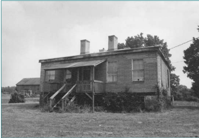
74B-015 Clagett House at Cool Spring Manor 17610 Clagett Landing Road Upper Marlboro vicinity
