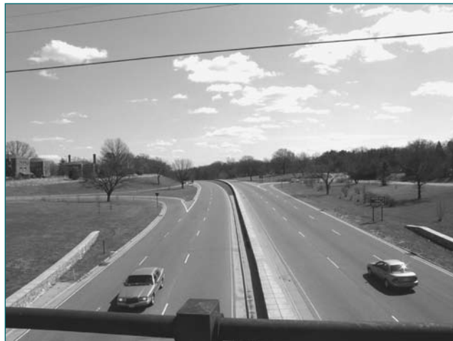
76A-022 Suitland Parkway (NR) From the North Gate of Andrews Air Force Base to Bolling Air Force Base (National Park Service, National Capital Region)
