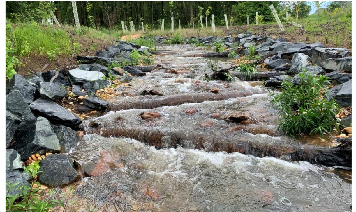
**Figure 25.** Log Roll Bioengineering Technique
