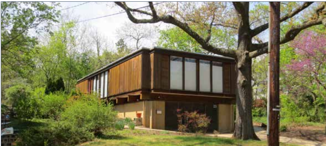
The Edwin Ball House is an example of properties developed as part of the Modern Movement.
