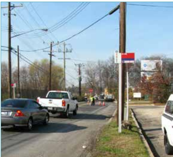
Many bus stops are poorly located and lack ADA accessible landing pads.
