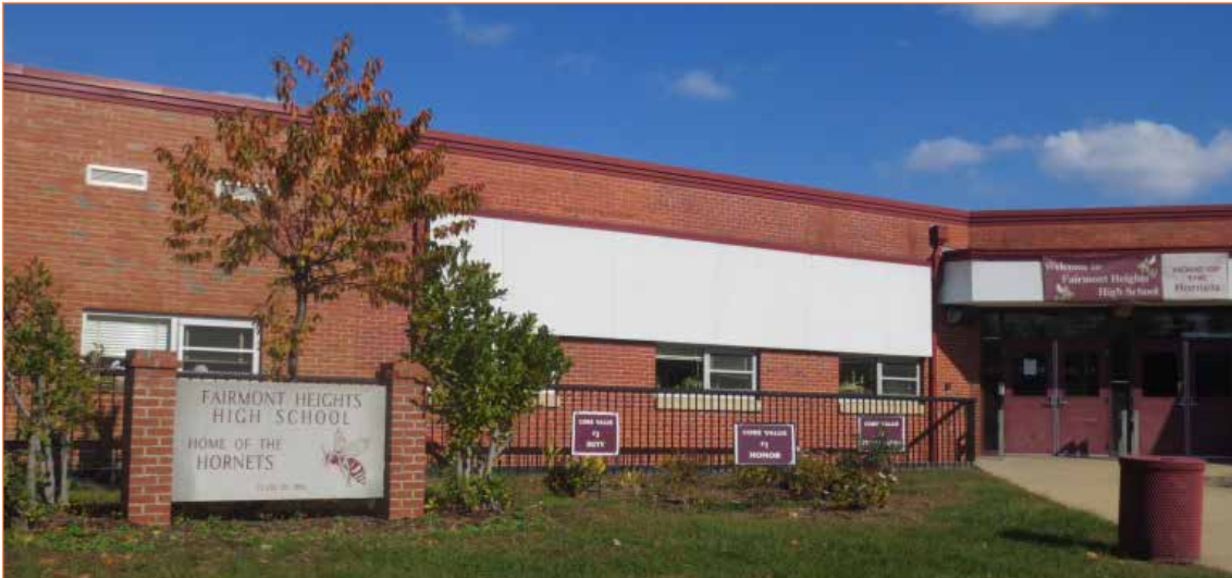
Adaptive reuse of Fairmont Heights High School provides new opportunities for future community uses.
