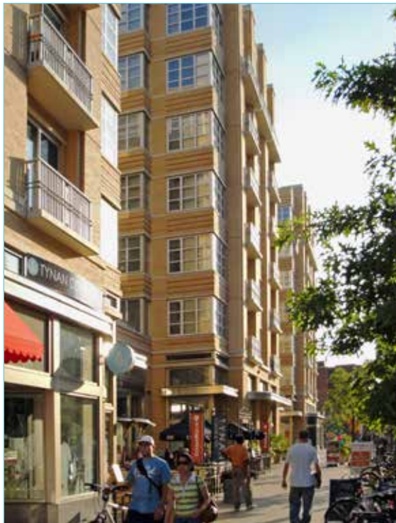
A mix of housing types provides opportunities for age-in-place features such as elevators and universal design.
