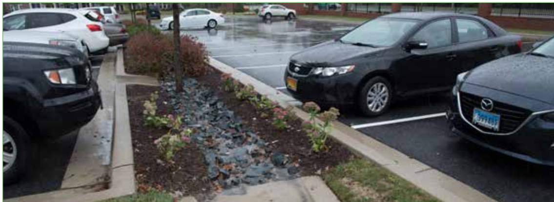
Bioswales are valuable interventions to treat runoff along linear facilities, such as roads, parking lots and buildings.
