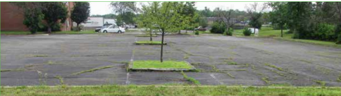
Large impervious surfaces contribute to the urban heat island effect and exacerbate stormwater management concerns in flood-prone areas.
