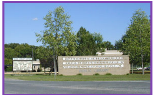
Multi-use public buildings, especially in the rural tier, are an integral part of the communities.
