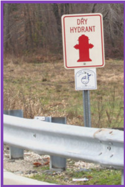
The rural tier portion of the subregion is not served with water and there are dry hydrants throughout the area to provide the volunteers with water.
