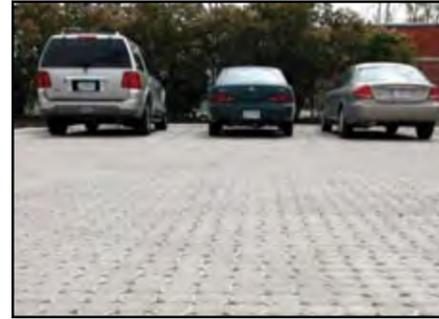
*Typical example of permeable paving*
