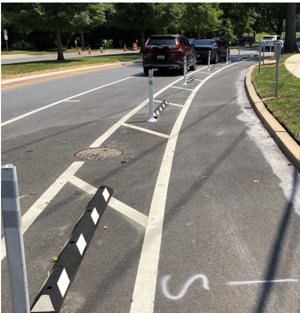
Buffered Bike Lanes – Flex-posts and Curb-stops
