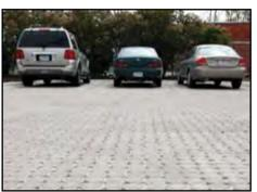
Typical example of permeable paving
