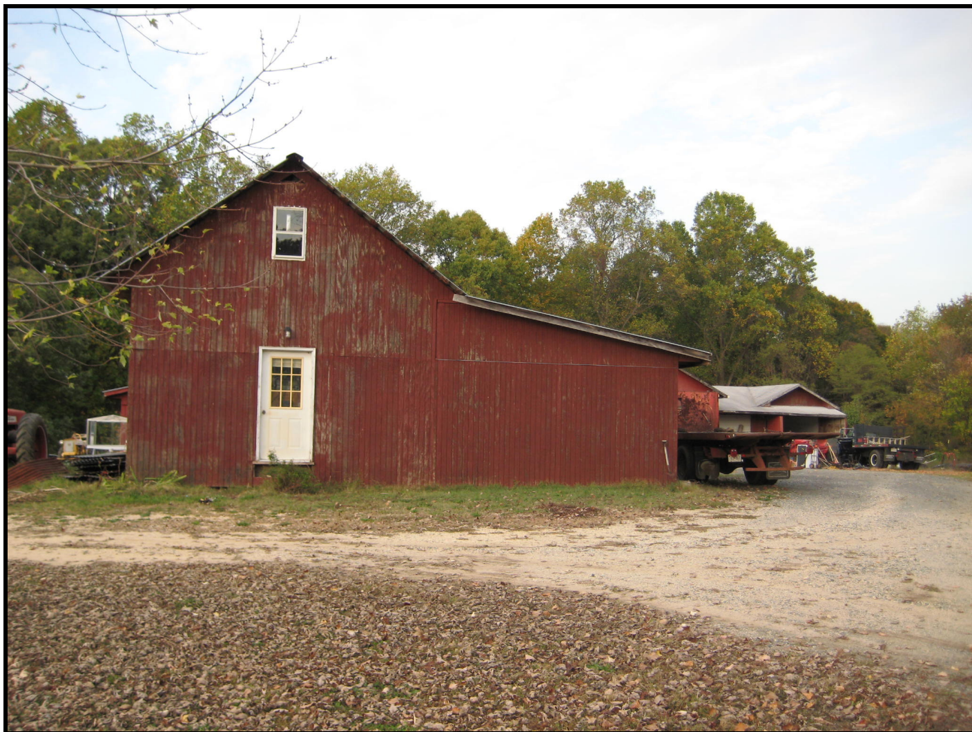
Photo: Garage (2), c. 1930, view of the south elevation, looking north. (November 2007)
