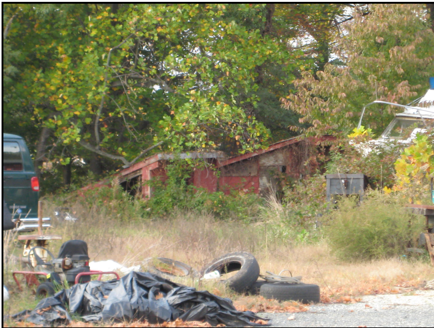
Photo: Shed (3) and Shed (4), c. 1965, view of the southeast elevation, looking northwest. (November 2007)
