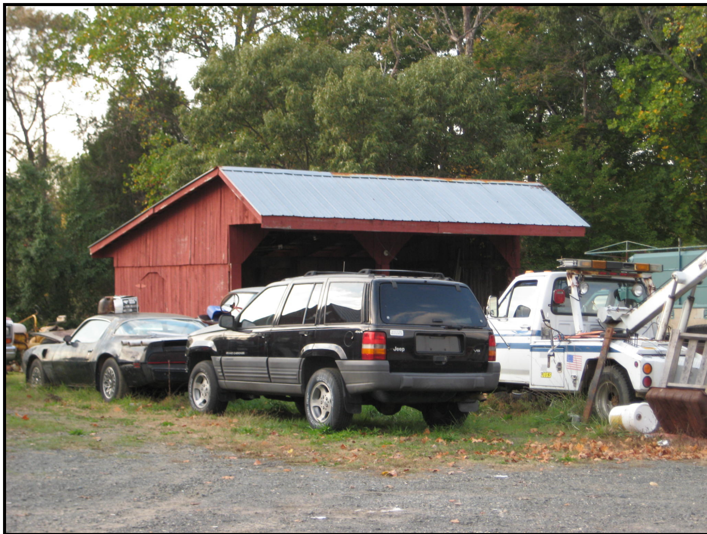
Photo: Garage (3), c. 1950, view of the façade (east elevation), looking west. (November 2007)
