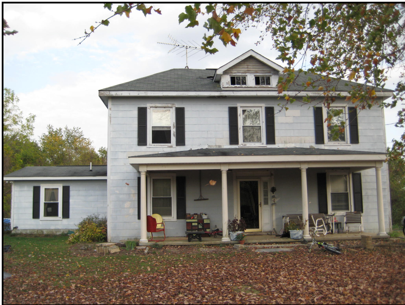
Photo: House at Magruder's Landing, c. 1910 building, view of the façade (west elevation), looking east. (November 2007)
