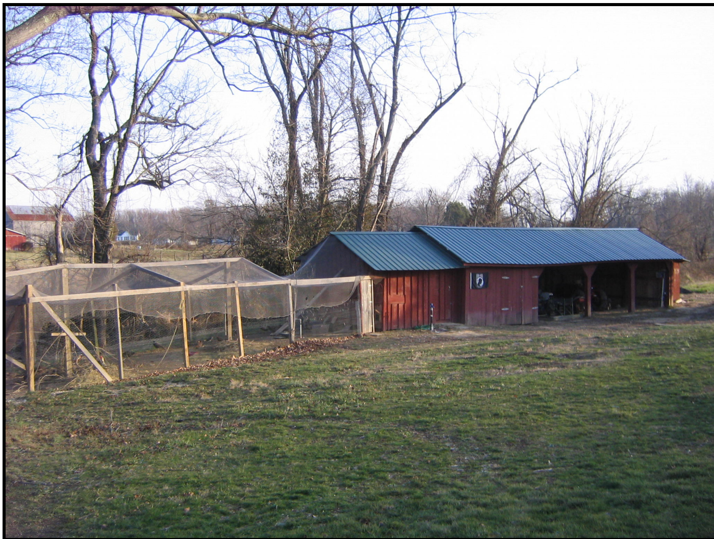
Photo: Shed (2), c. 2005, view of the façade (northwest elevation), looking southeast. (January 2008)
