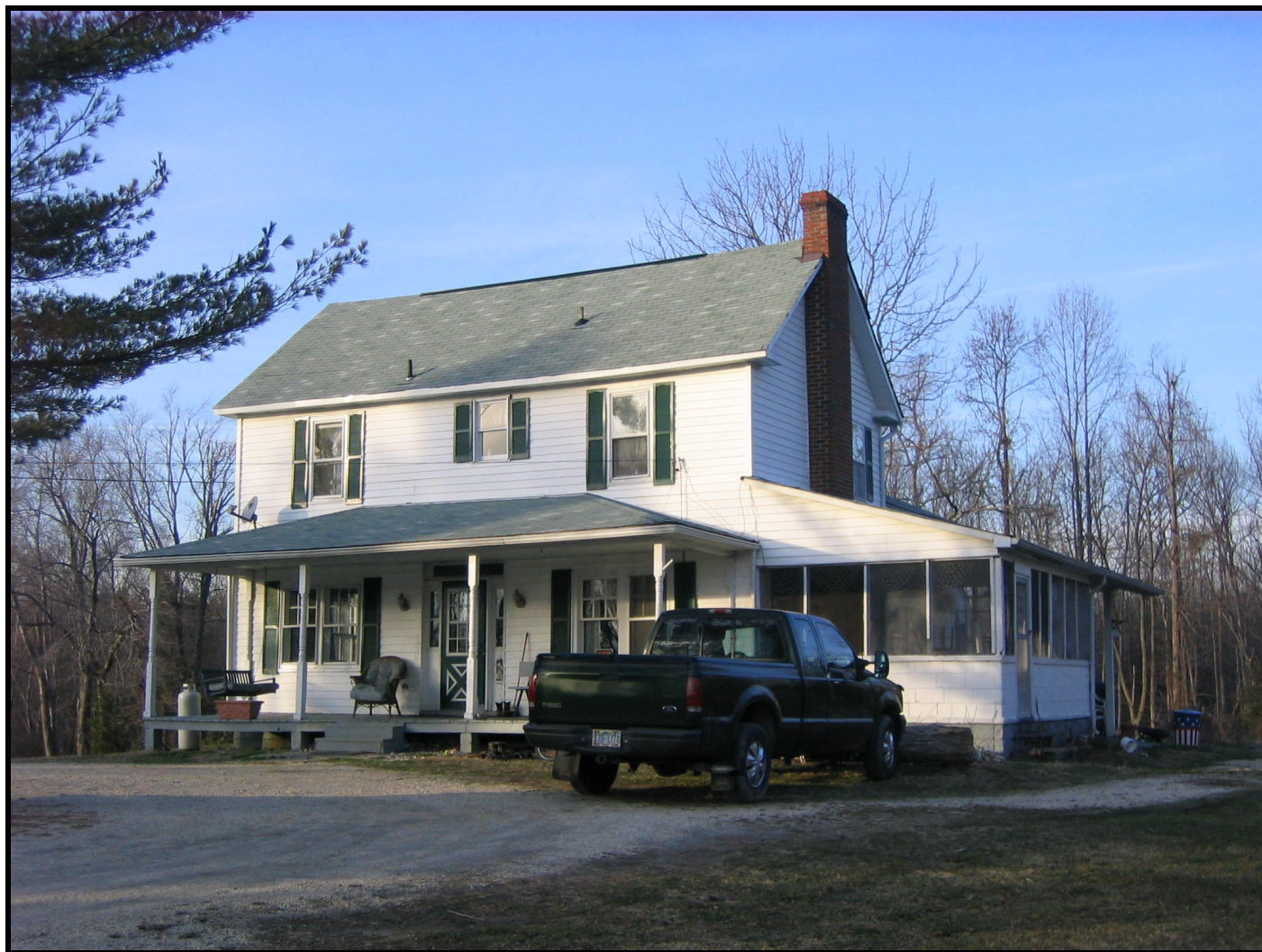
Photo: Orme-Carr House, 1912, view of the southeast corner, looking northwest. (January 2008)
