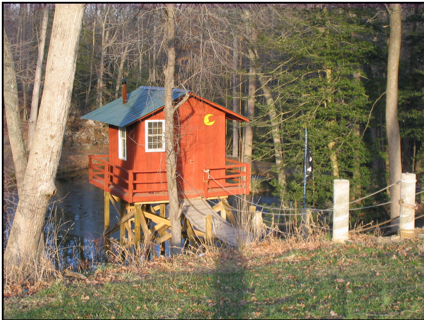
Photo: Elevated Outbuilding, c. 2005, view looking northeast. (January 2008)
