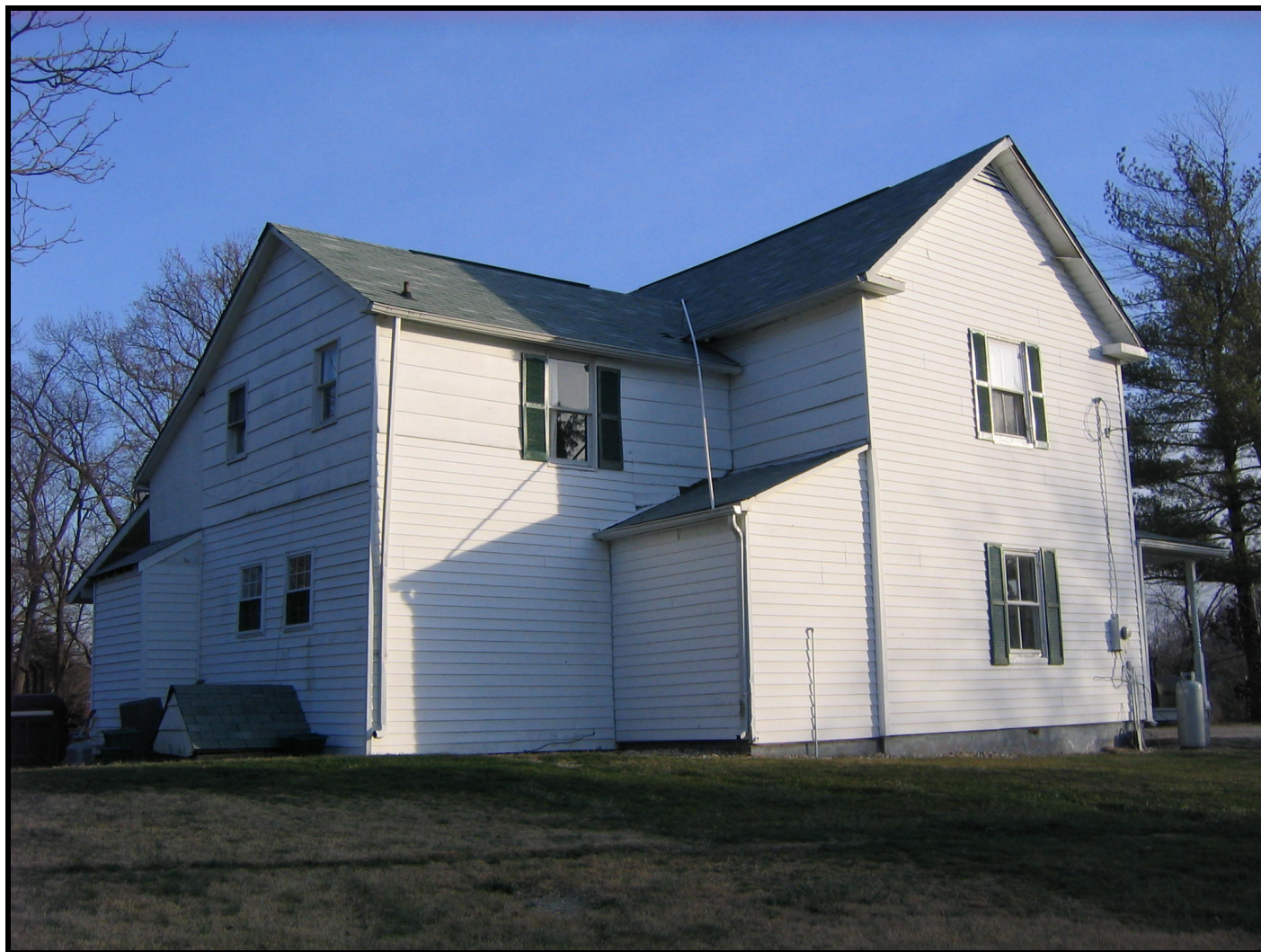
Photo: Orme-Carr House, 1912, view of the northwest corner, looking southeast. (January 2008)
