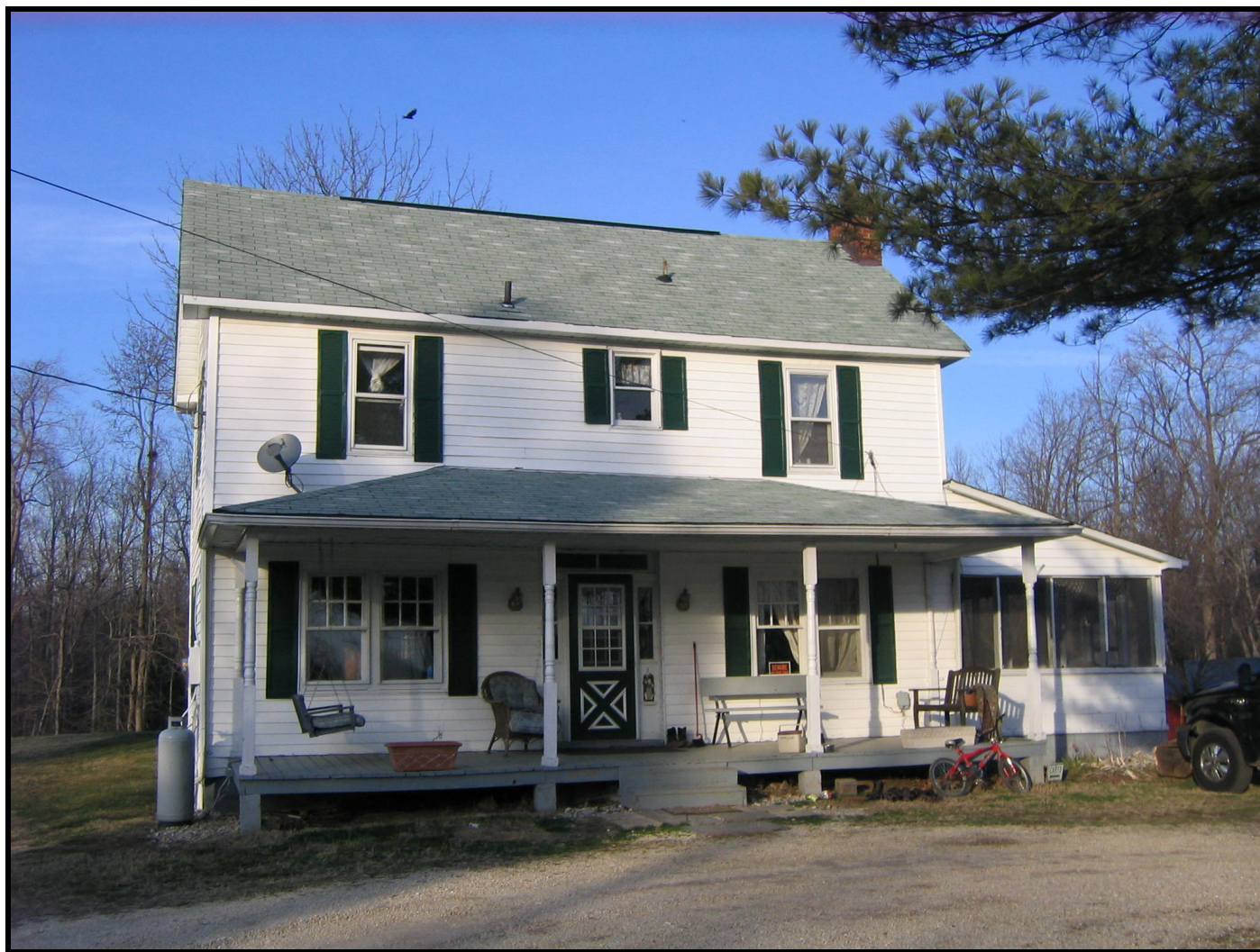
Photo: Orme-Carr House, 1912, view of the façade (south elevation), looking north. (January 2008)
