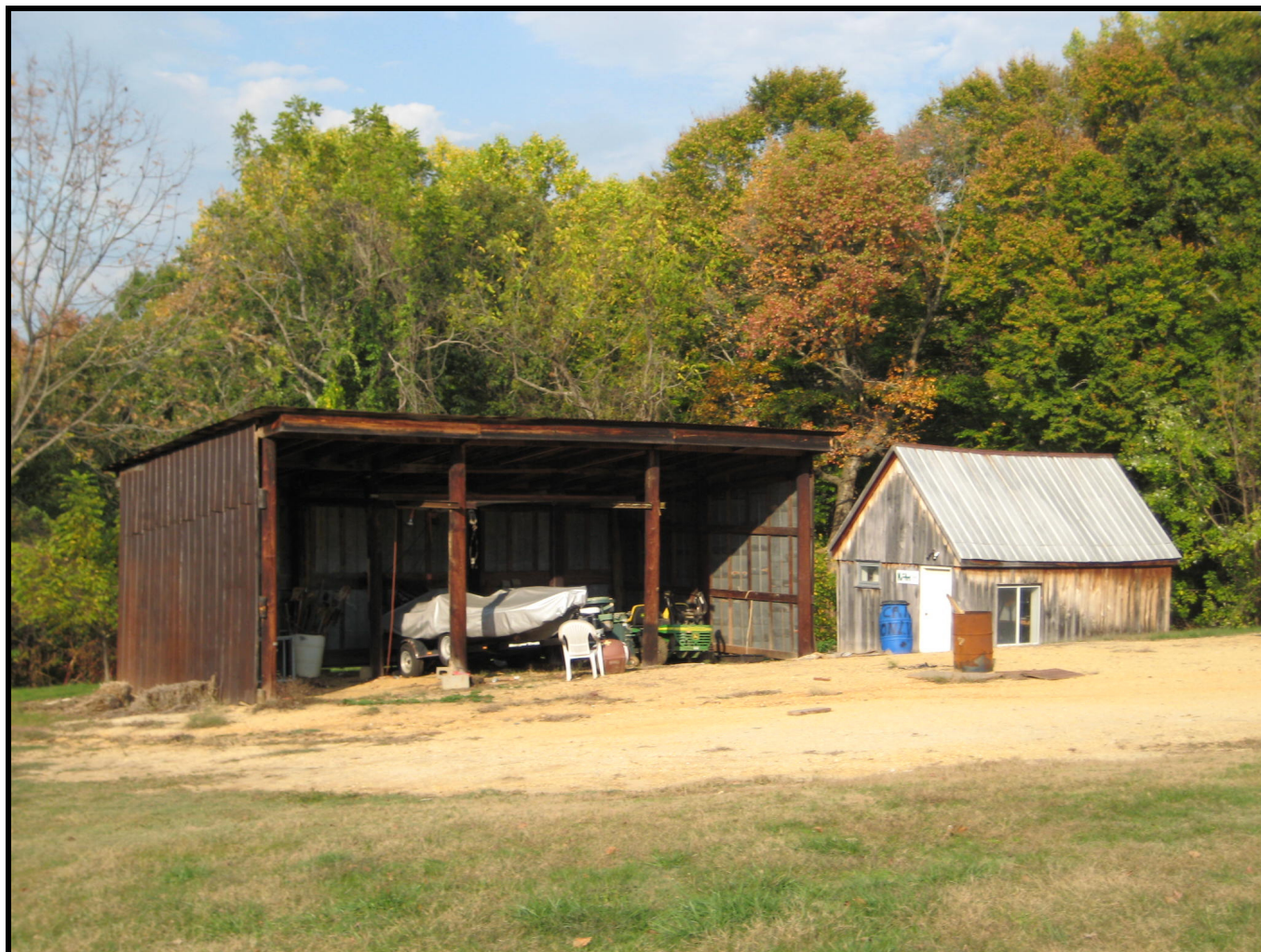
Photo: Shed (1), view of the façade (south elevation), looking northeast. (November 2007)
