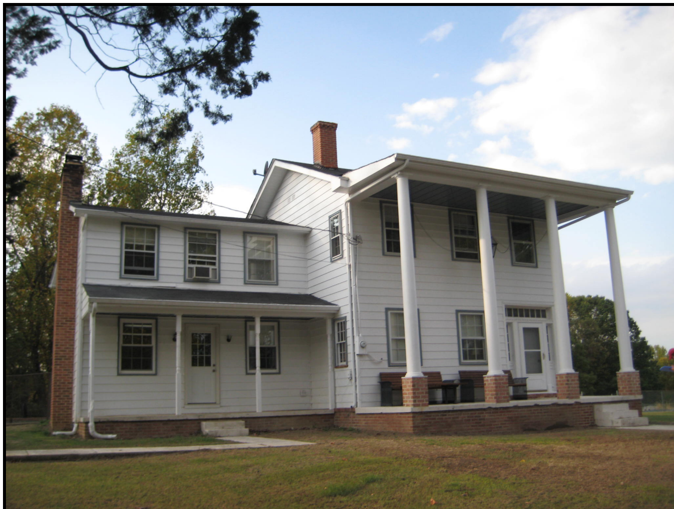
Photo: Margaret Baden House, view of the façade (east elevation), looking west. (November 2007)
