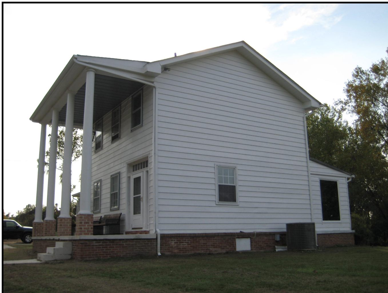
Photo: Margaret Baden House, view of the north (side) elevation, looking southwest. (November 2007)
