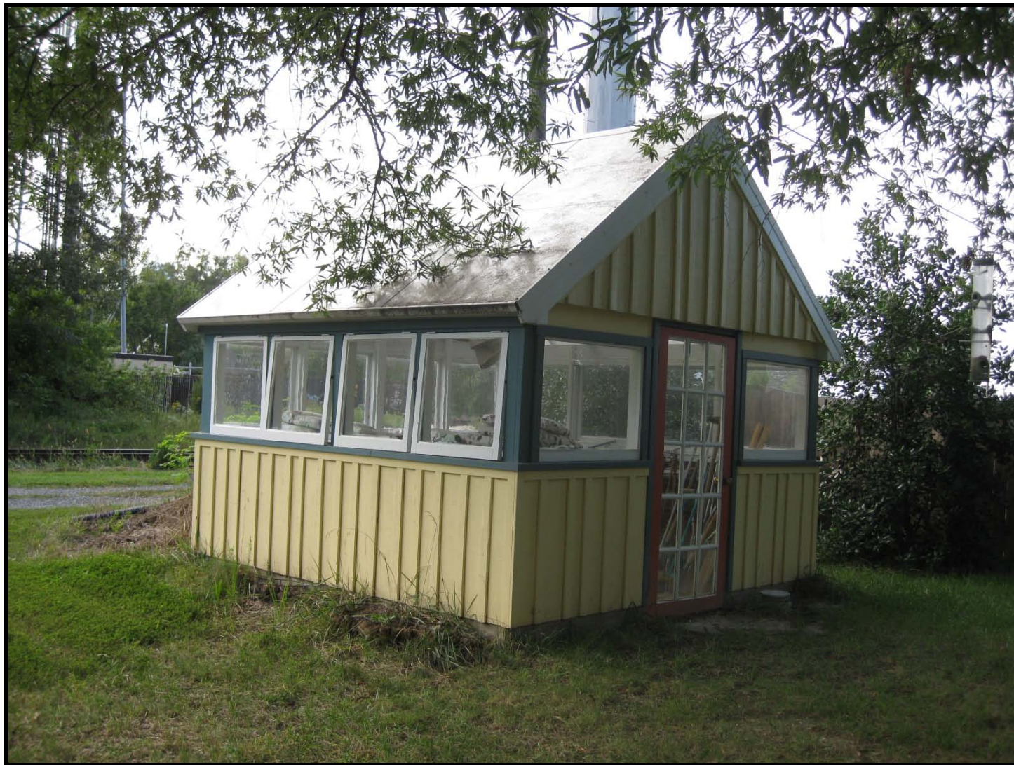
Photo: Greenhouse, Brandywine, facade (northwest elevation) and side (northeast) elevation, looking southeast. (September 2009)
