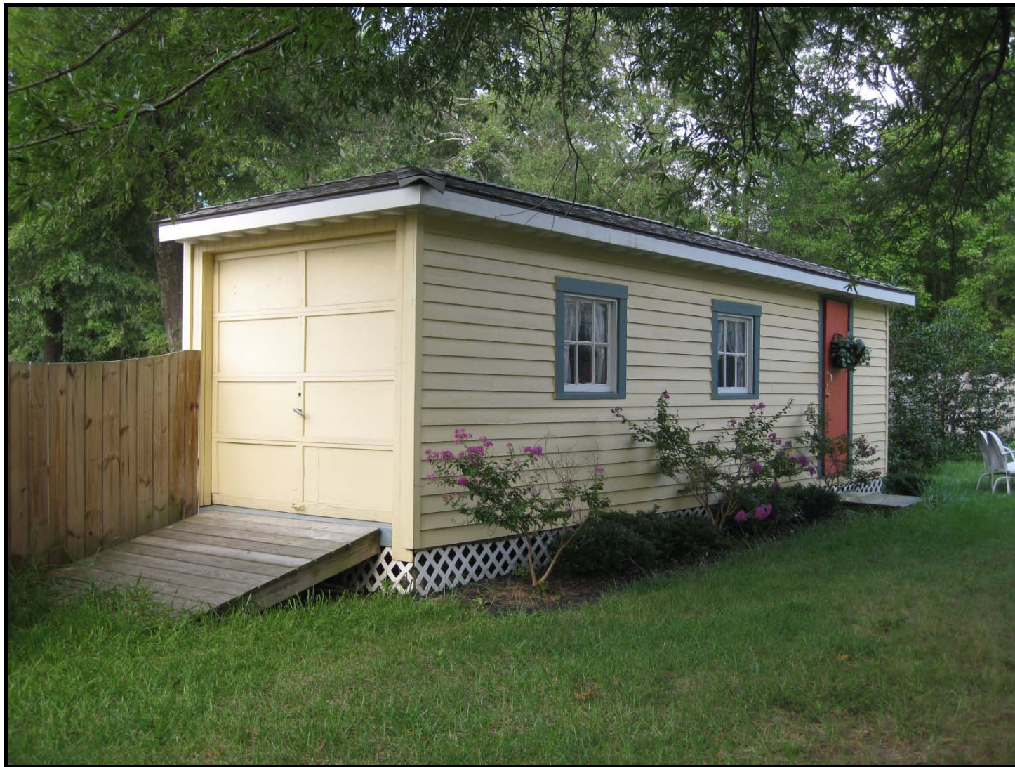
Photo: Shed #2, Brandywine, facade (southeast elevation), looking northwest. (September 2009)
