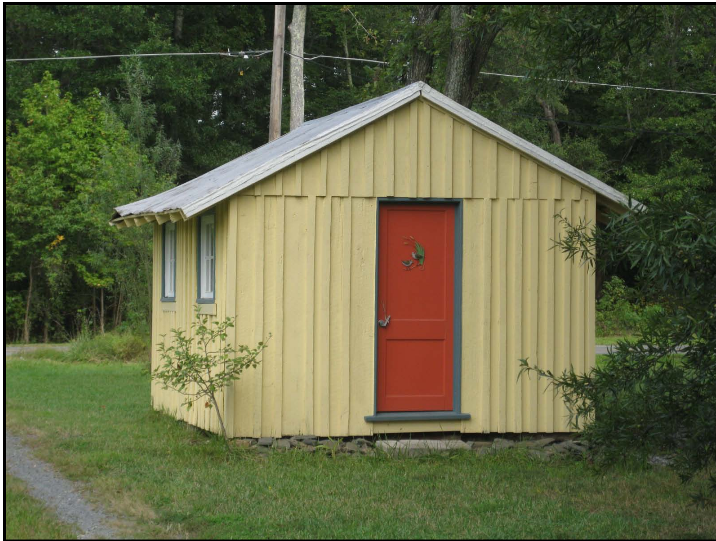
Photo: Shed #1, Brandywine, facade (southeast elevation), looking northwest. (September 2009)
