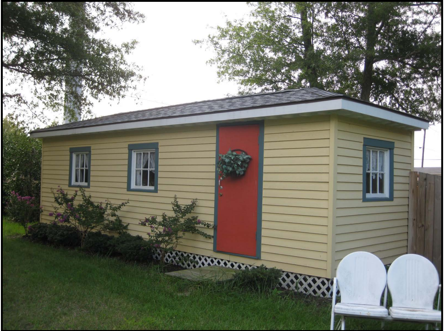
Photo: Shed #2, Brandywine, shed 2, side (northeast) and rear (northwest) elevations, looking southeast. (September 2009)
