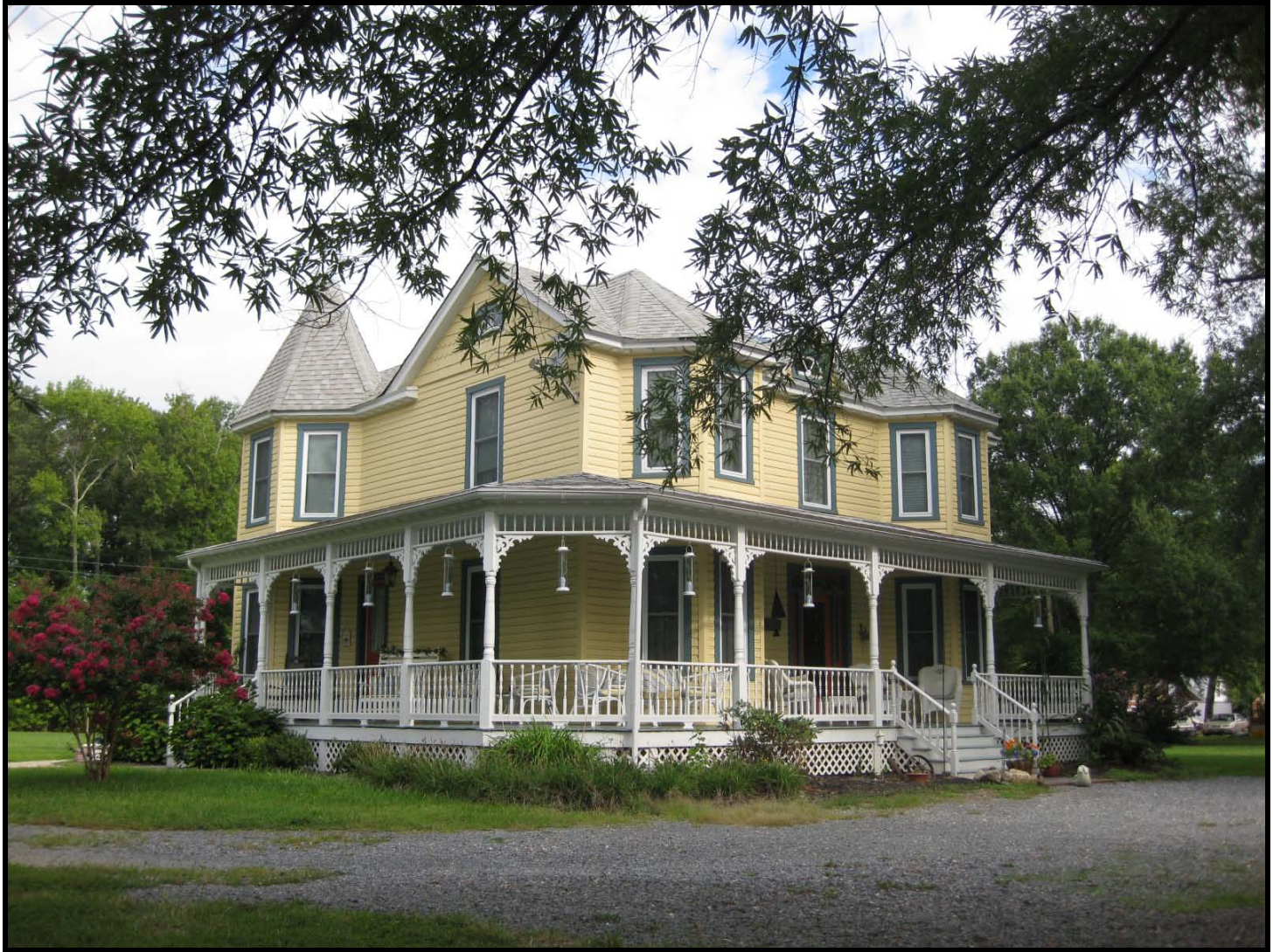
Photo: William B. Early House, Brandywine, façade (southeast elevation) and side (southwest) elevation, looking north. (September 2009)
