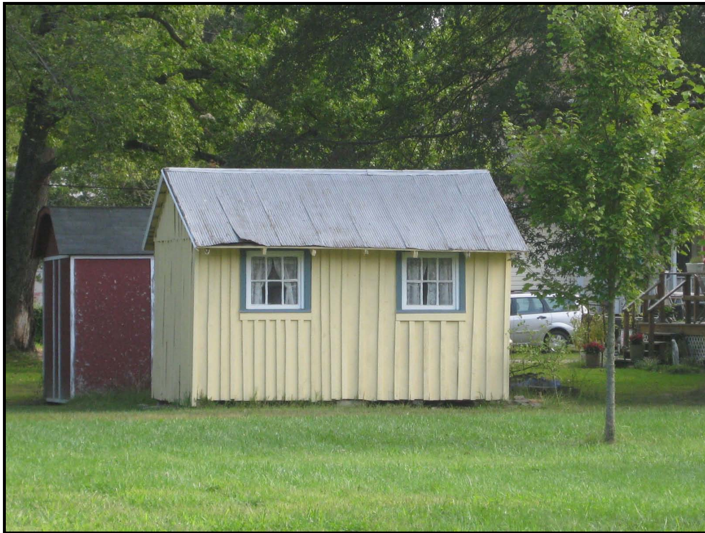
Photo: Shed #1, Brandywine, side (southwest) elevation, looking southeast. (September 2009)
