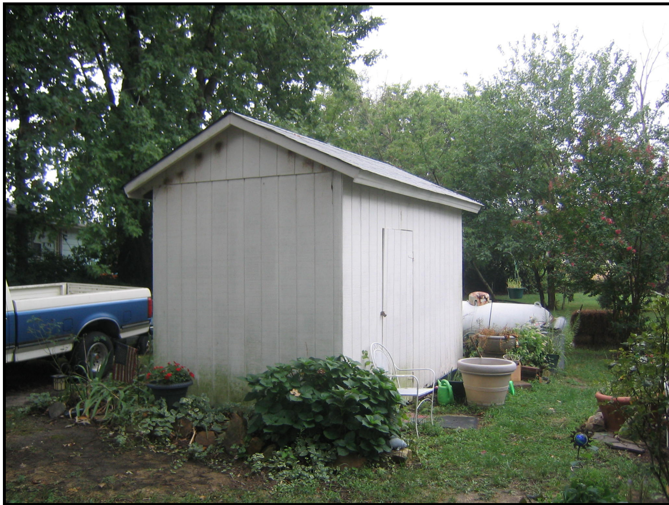
Photo: Prefabricated Shed, looking southwest. (August 2007)
