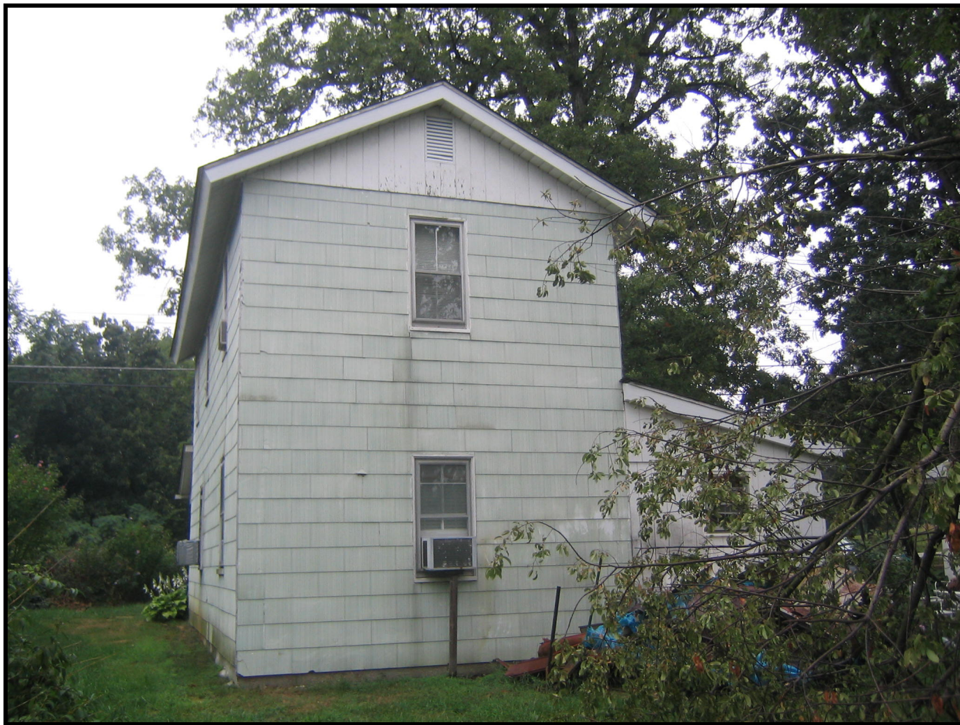
Photo: Old Cheltenham Dwelling, west (rear) elevation, looking east. (August 2007)
