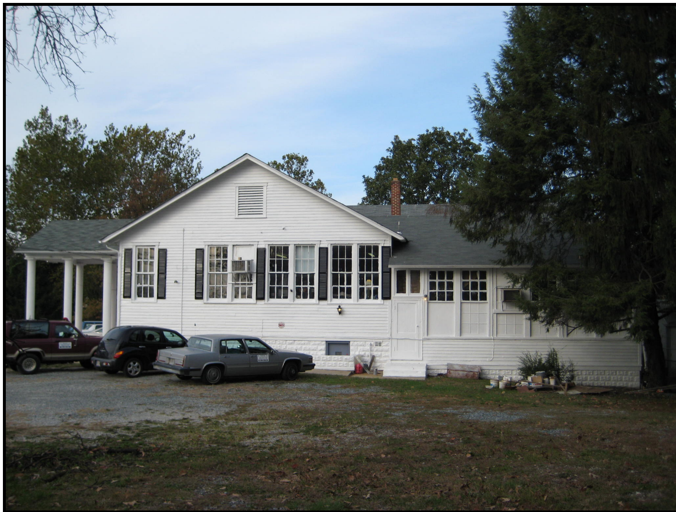
Photo: Forestville School, view of the east (side) elevation, looking west. (November 2007)
