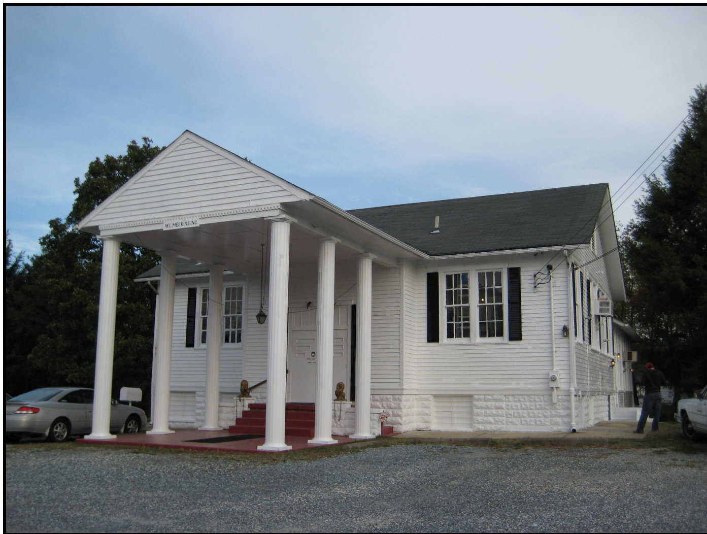
Photo: Forestville School, view of the façade (south elevation), looking north. (November 2007)
