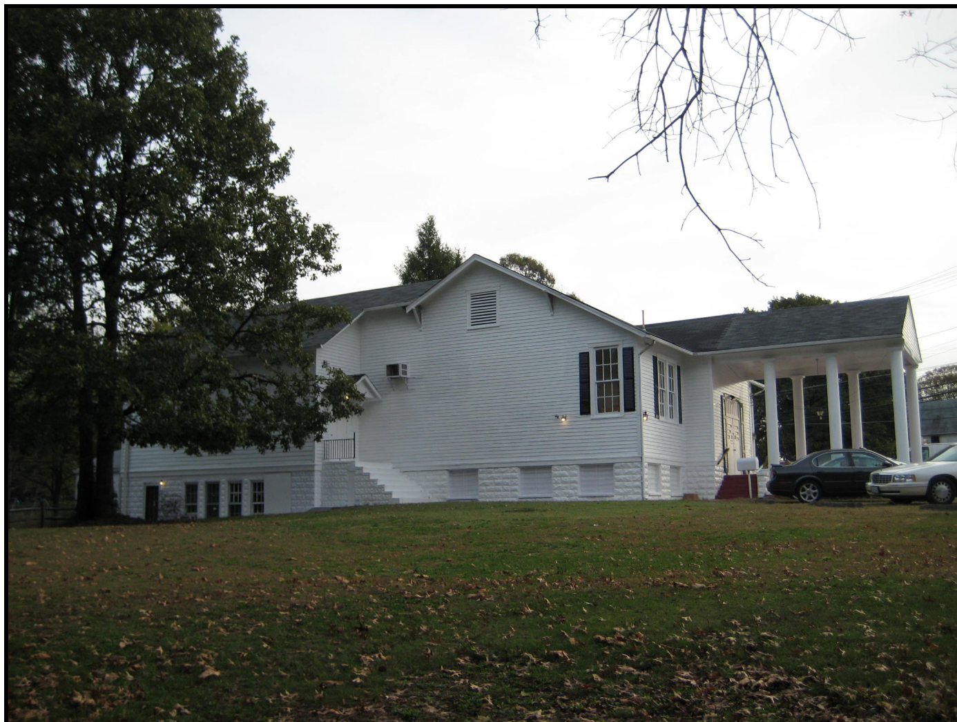
Photo: Forestville School, view of the west (side) elevation, looking northeast. (November 2007)
