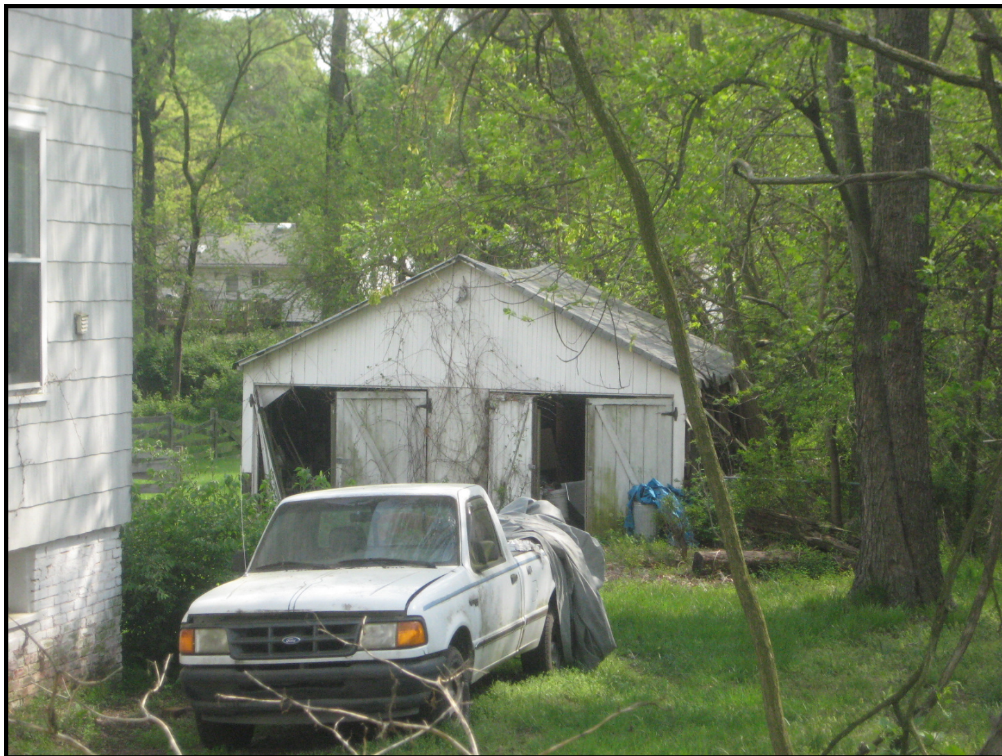
Photo: Garage, Berwyn Heights, view of the façade (north elevation), looking southeast. (April 2008)
