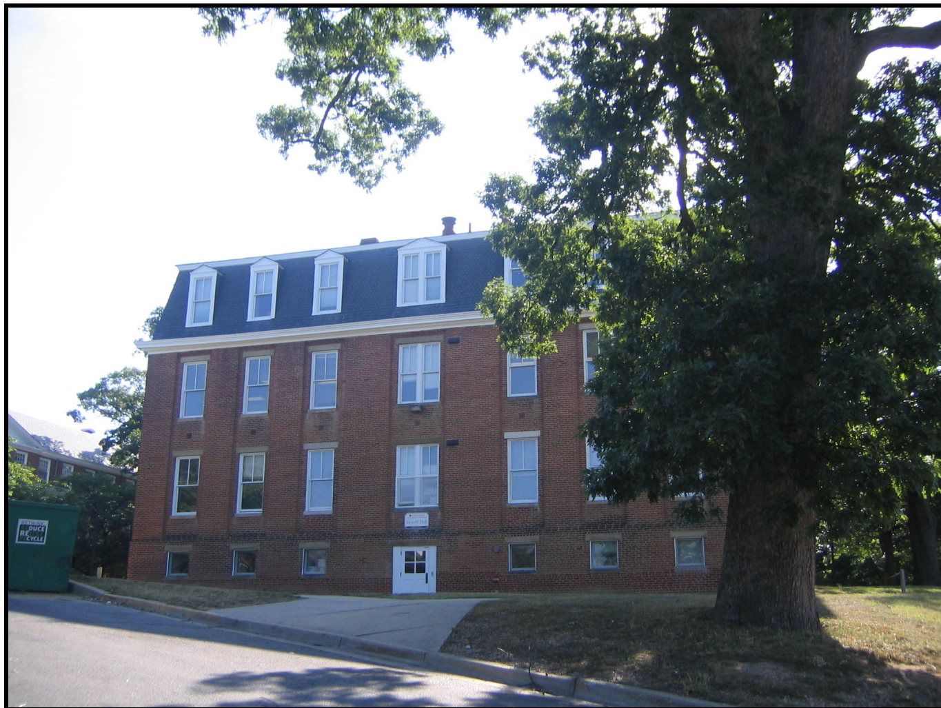
Photo: Morrill Hall, west (rear) elevation, looking east.
