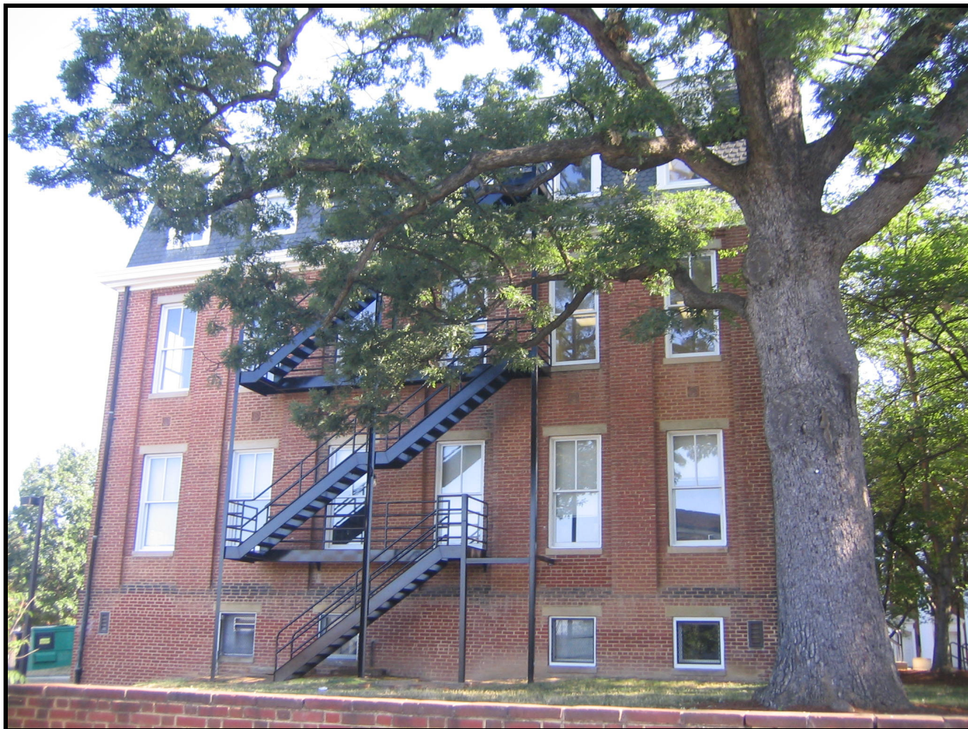
Photo: Morrill Hall, south (side) elevation, looking north.
