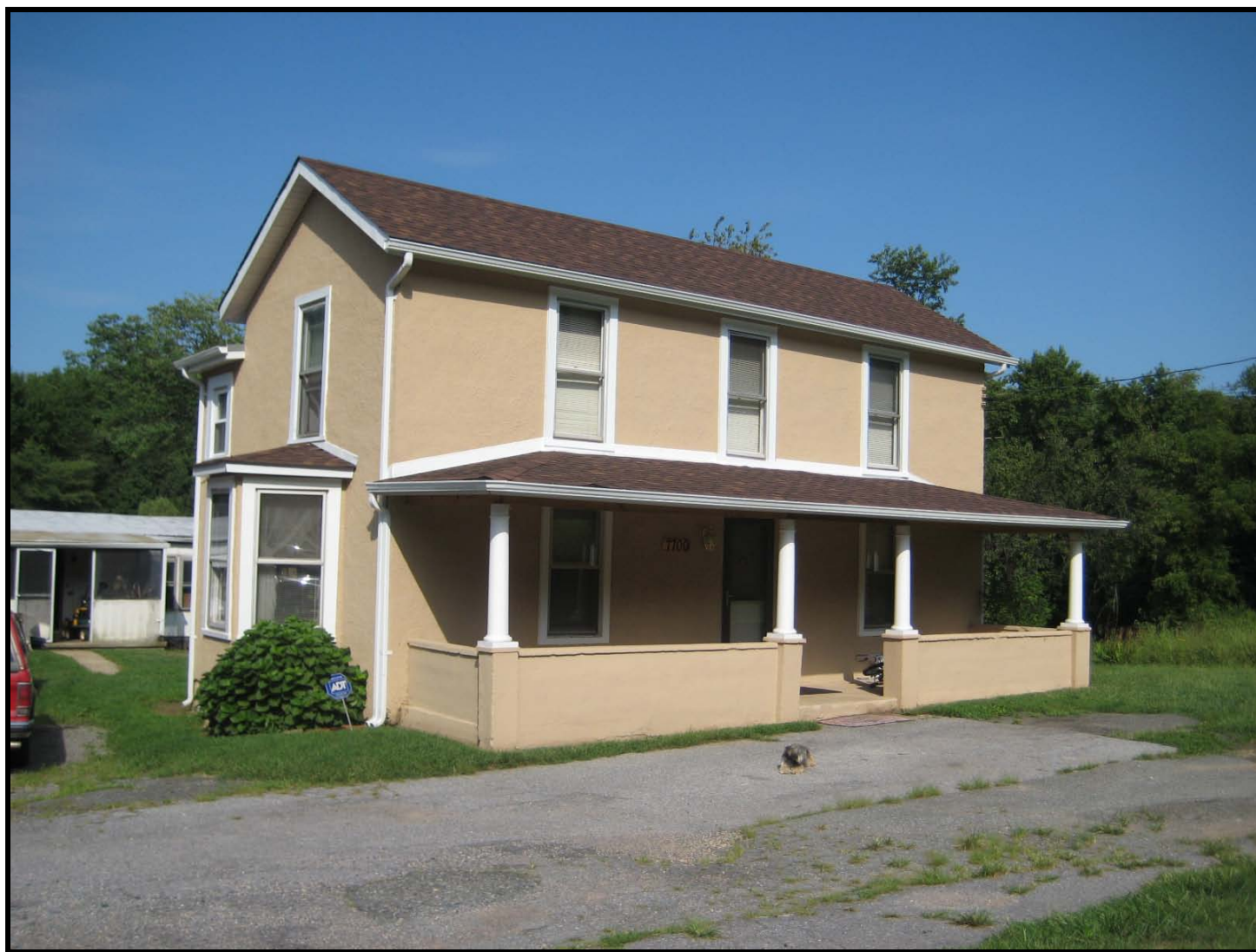
Photo: Thomas Matthews House (c. 1888), Beltsville, façade (southwest elevation), view looking east. (August 2009)
