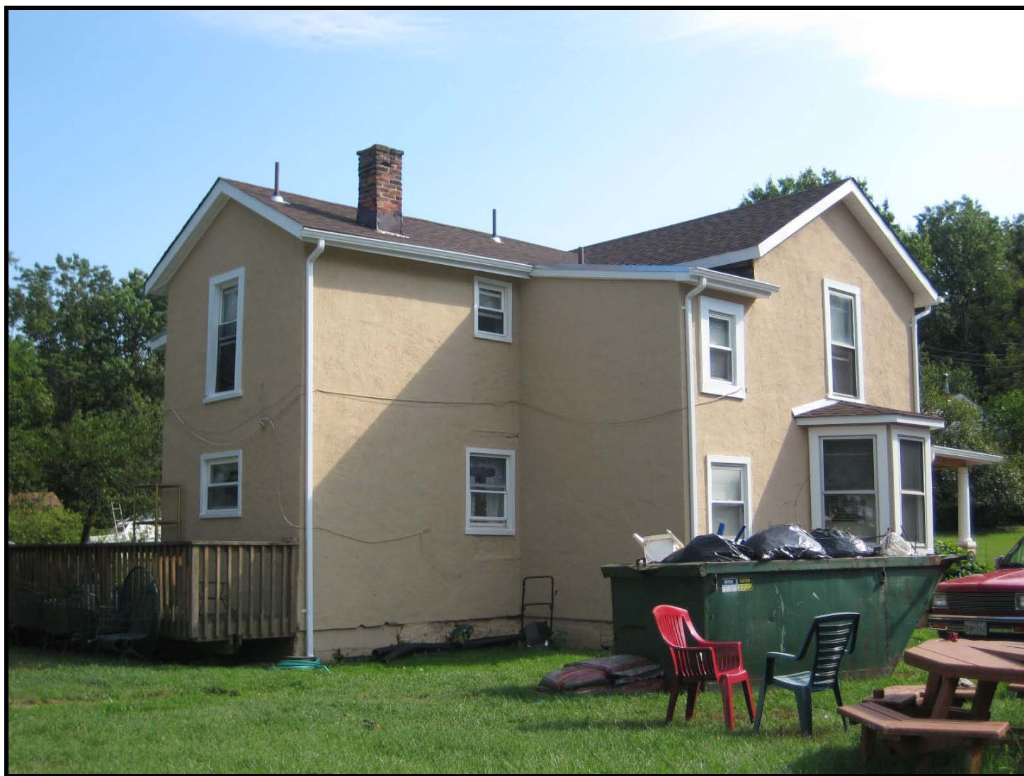
Photo: Thomas Matthews House (c. 1888), Beltsville, rear (northeast) elevation, view looking south. (August 2009)
