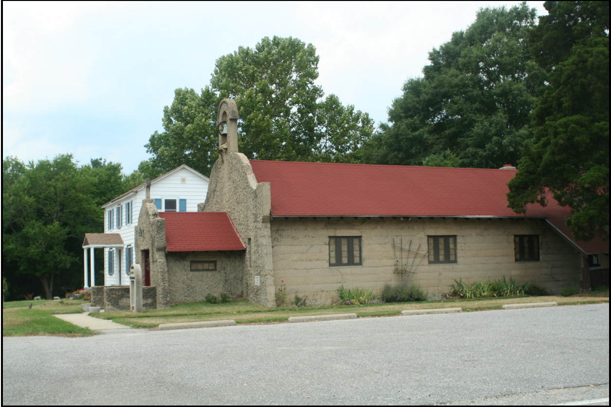
Looking northwest, 14068-14070 Brandywine Road (Chapel of the Incarnation, PG: 85A-032-27) ( EHT Traceries , 2007)
