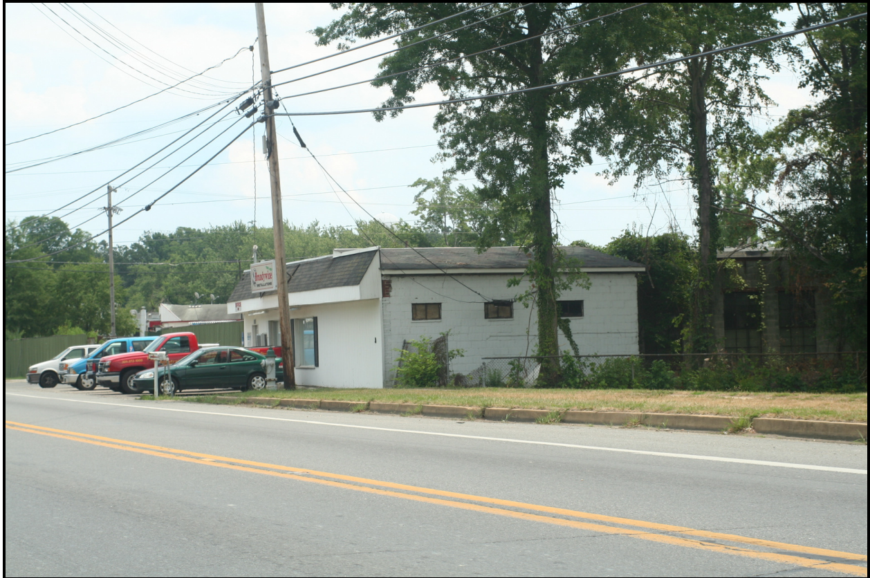
Looking southeast, 14105 Brandywine Road ( EHT Traceries , 2007)
