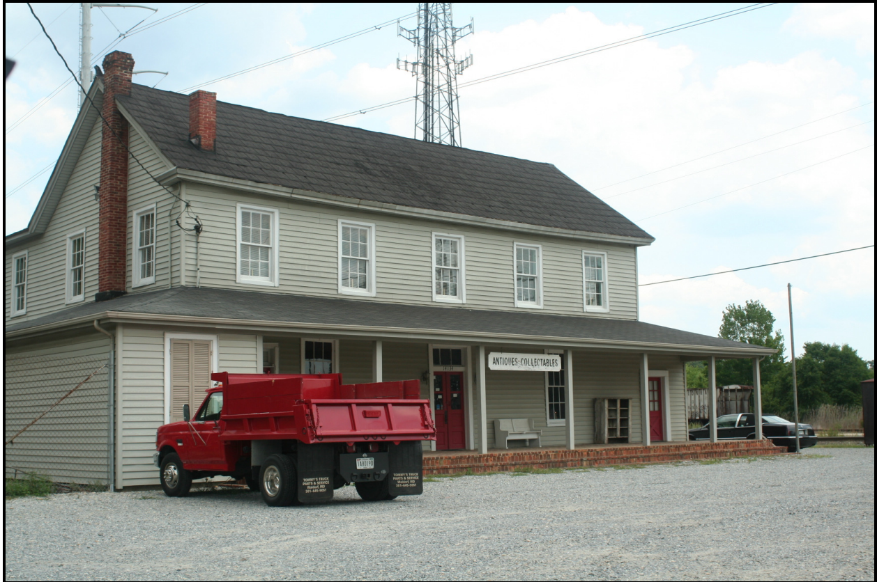
Looking east, W.H. Early Store (PG: 85A-032-11), 14034 Brandywine Road ( EHT Traceries , 2007)
