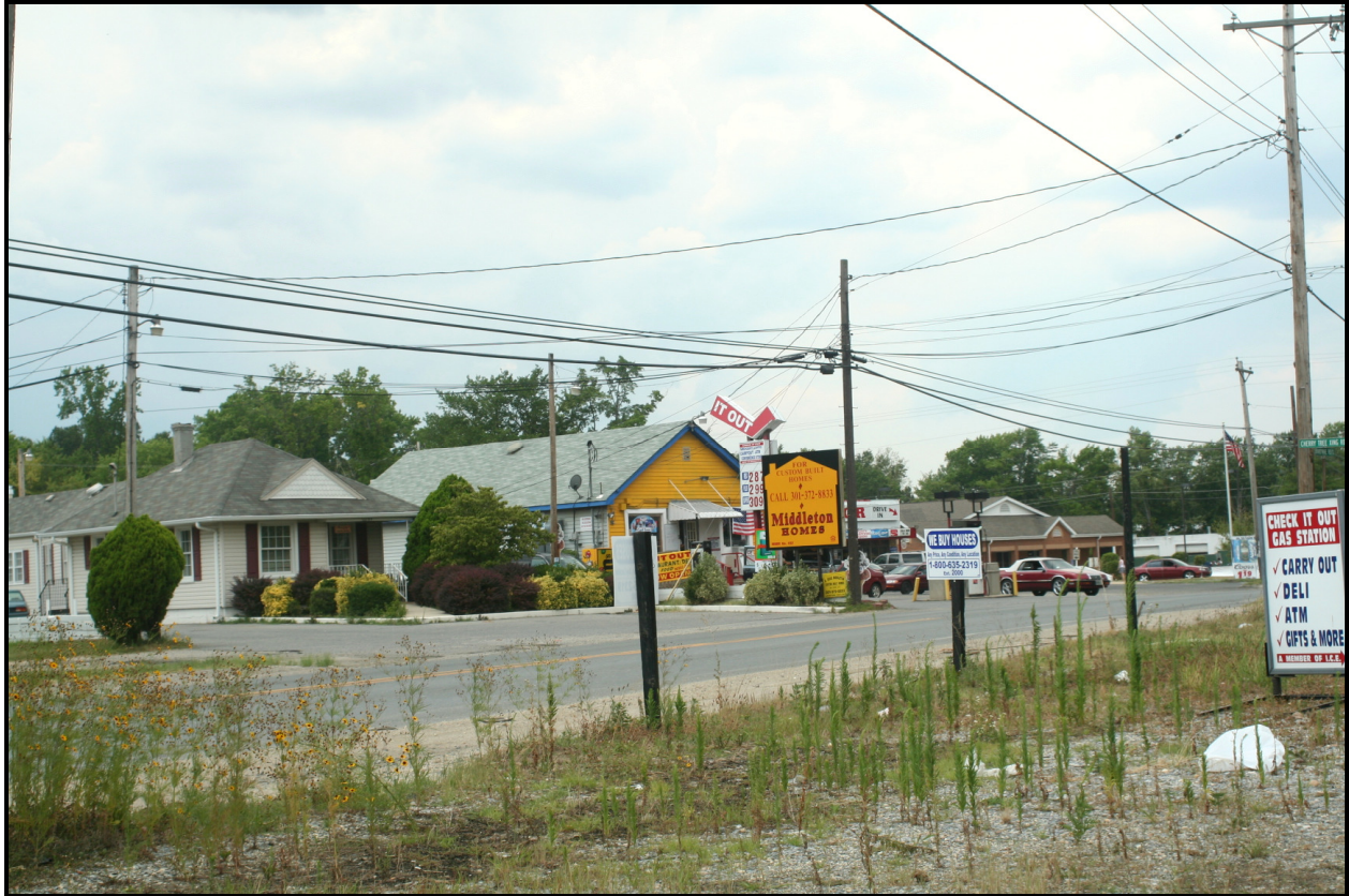
Looking southwest, 14127-14125 Brandywine Road ( EHT Traceries, 2007 )
