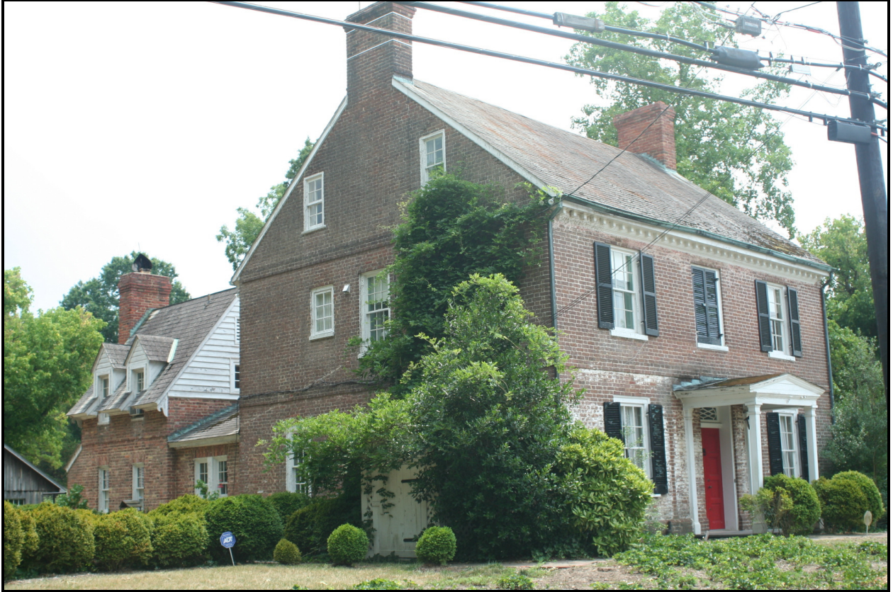
Looking southwest, Hardy's Tavern (PG: 84-023-05), 2305 Floral Park Road ( EHT Traceries , 2007)
