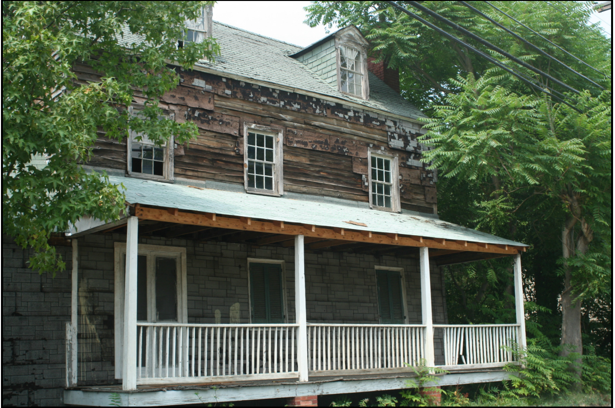
Looking north, Piscataway Tavern (PG: 84-023-03), 2204 Floral Park Road ( EHT Traceries , 2007)
