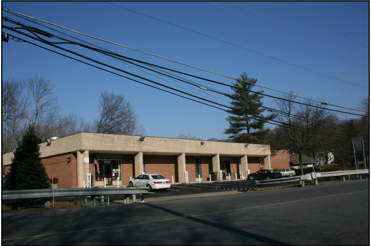
Looking north, 10909 Fort Washington Road ( EHT Traceries, 2009 )
