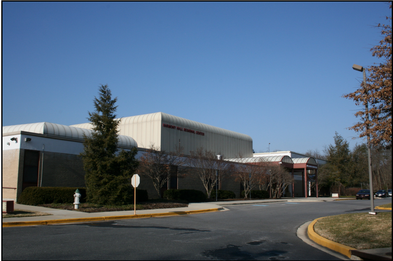
Looking northwest, Harmony Hall Regional Center, 10701 Livingston Road, in Broad Creek Historic District ( EHT Traceries , 2009)
