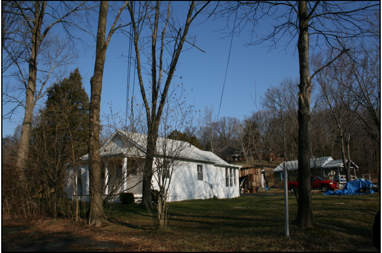
Looking northeast, 11011-11009 Fort Washington Road ( EHT Traceries, 2009 )
