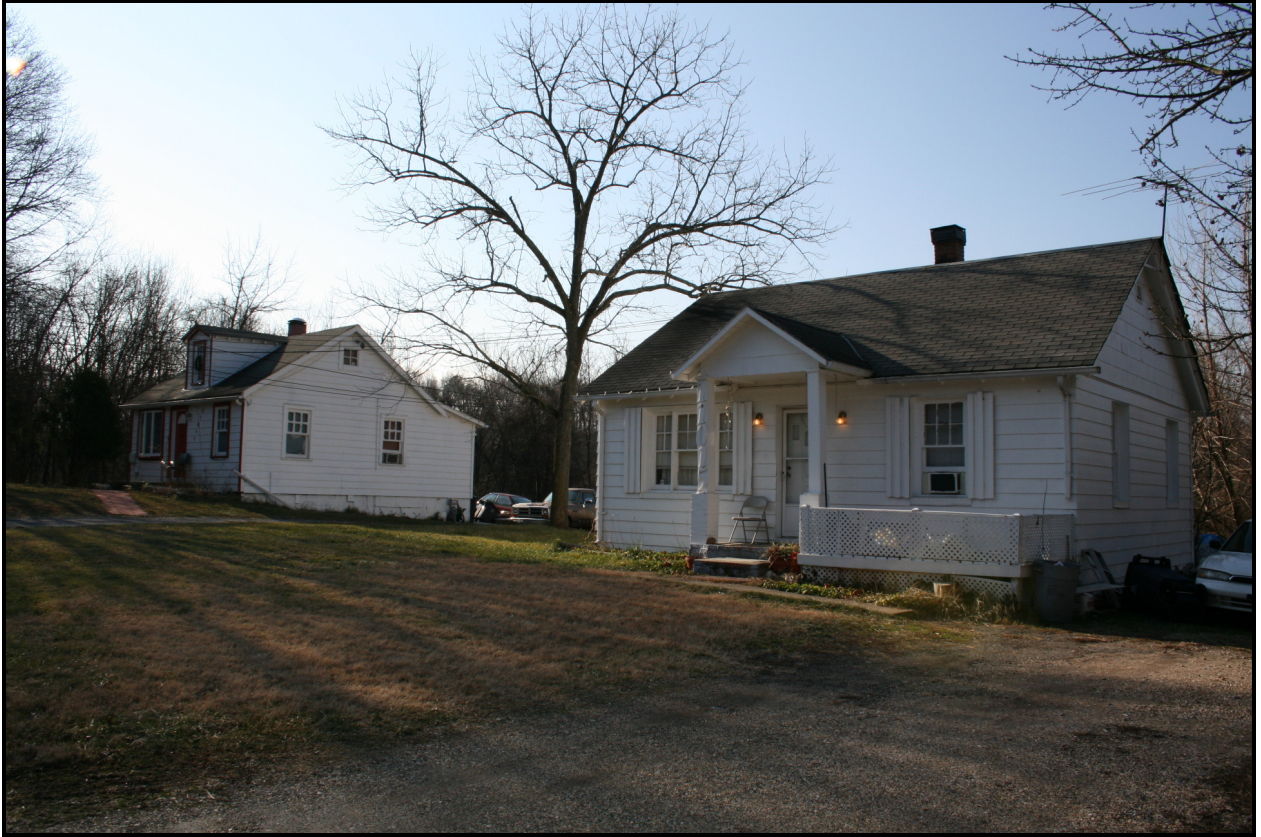
Looking south, 11015-11019 Livingston Road ( EHT Traceries , 2009)
