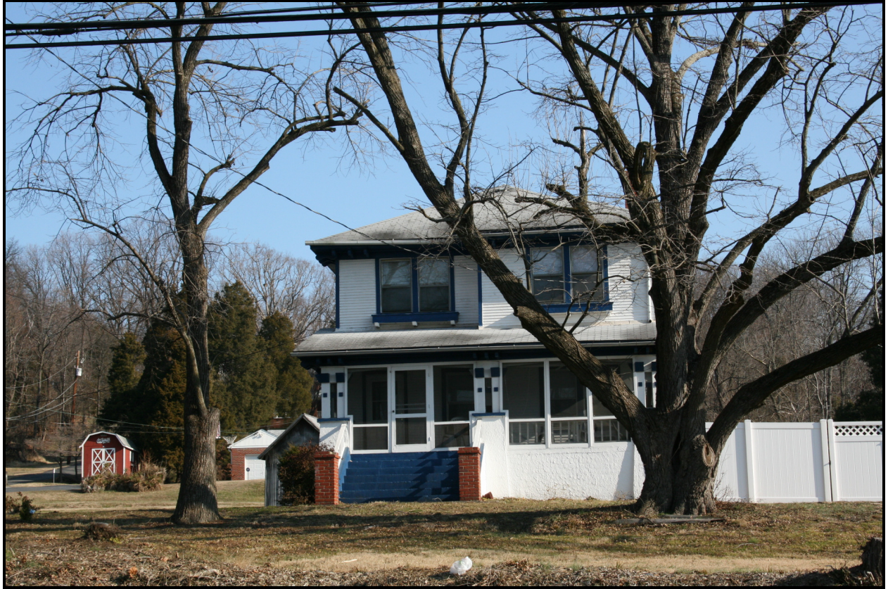
Looking east, 10706 Livingston Road ( EHT Traceries , 2009)
