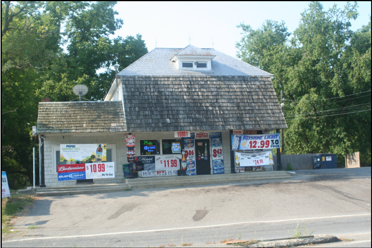
Looking south, 16001 Marlboro Pike, Wells Corner (EHT Traceries, 2007)
