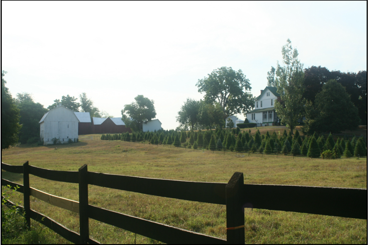
Looking southeast, Wyvill House/Linden Hill (PG: 79-063-50), 4102 Old Crain Highway ( EHT Traceries , 2007)
