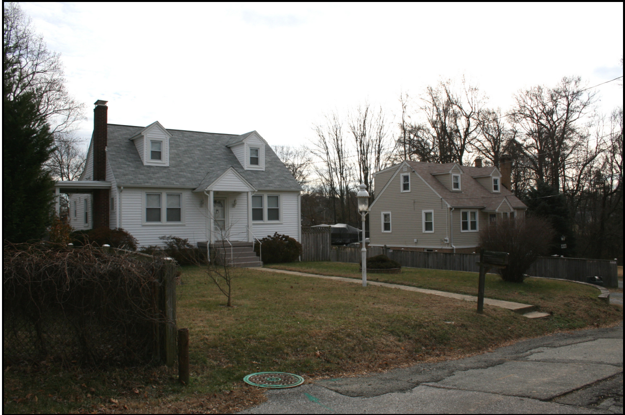
Glenn Hills, looking south, 5211-5209 Glenn Hills Roadway ( EHT Traceries, 2008 )
