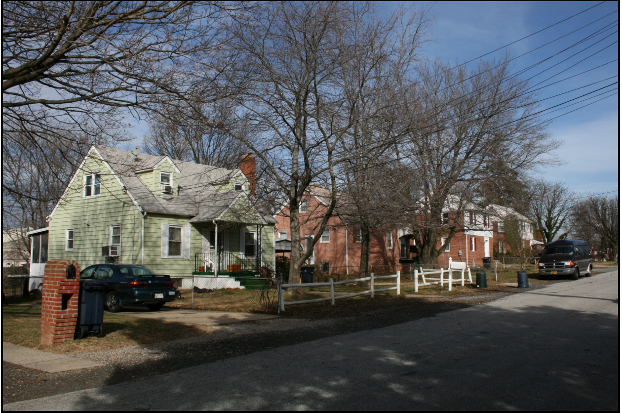
T.B. Middleton Farm, looking northeast, 5711-5709-5705 Linda Lane ( EHT Traceries , 2008)
