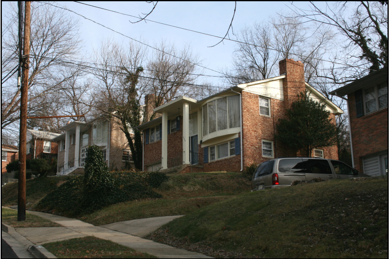
Looking southeast, 2409-2411 Fairlawn Street, Hillcrest Heights ( EHT Tracerics, 2009 )
