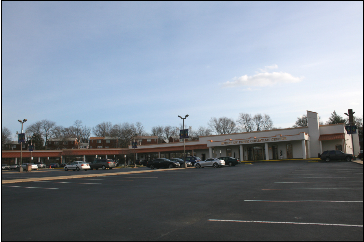
Looking south, Spirit of Faith Christian Center, 2261 Oxon Run Drive, Oxon Run Hills ( EHT Traceries, 2009 )
