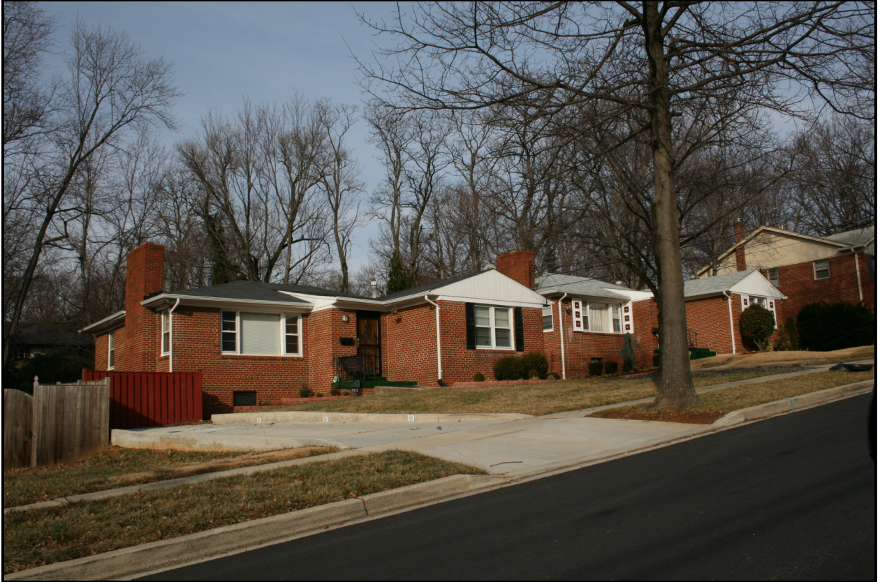
Looking northeast, 2414-2414 Fairlawn Street, Hillcrest Heights ( EHT Traceries , 2009)
