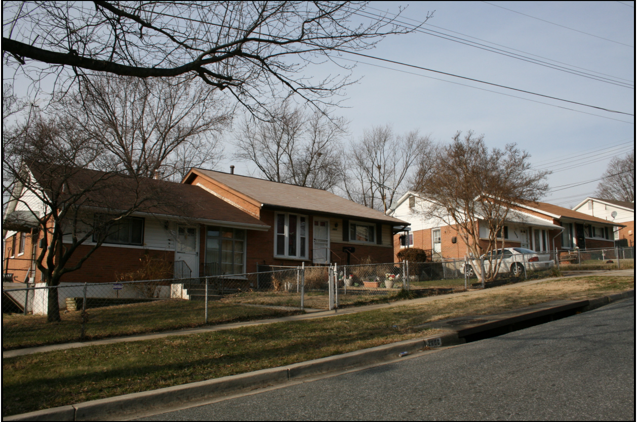
Looking north, 2600/2602-2604/2606 Afton Street (twin houses), Good Hope Hills ( EHT Traceries , 2009)
