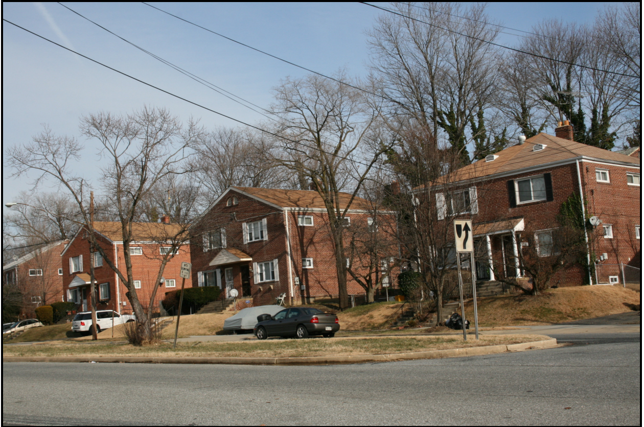
Looking northeast, 4030/4028-4026/4024-4022/4020 Lyons Street (twin houses), Hillcrest Heights ( EHT Traceries , 2009)
