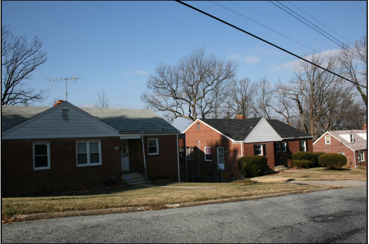
Looking northwest, 5701-5611-5609 Ottawa Street ( EHT Traceries , 2009)
