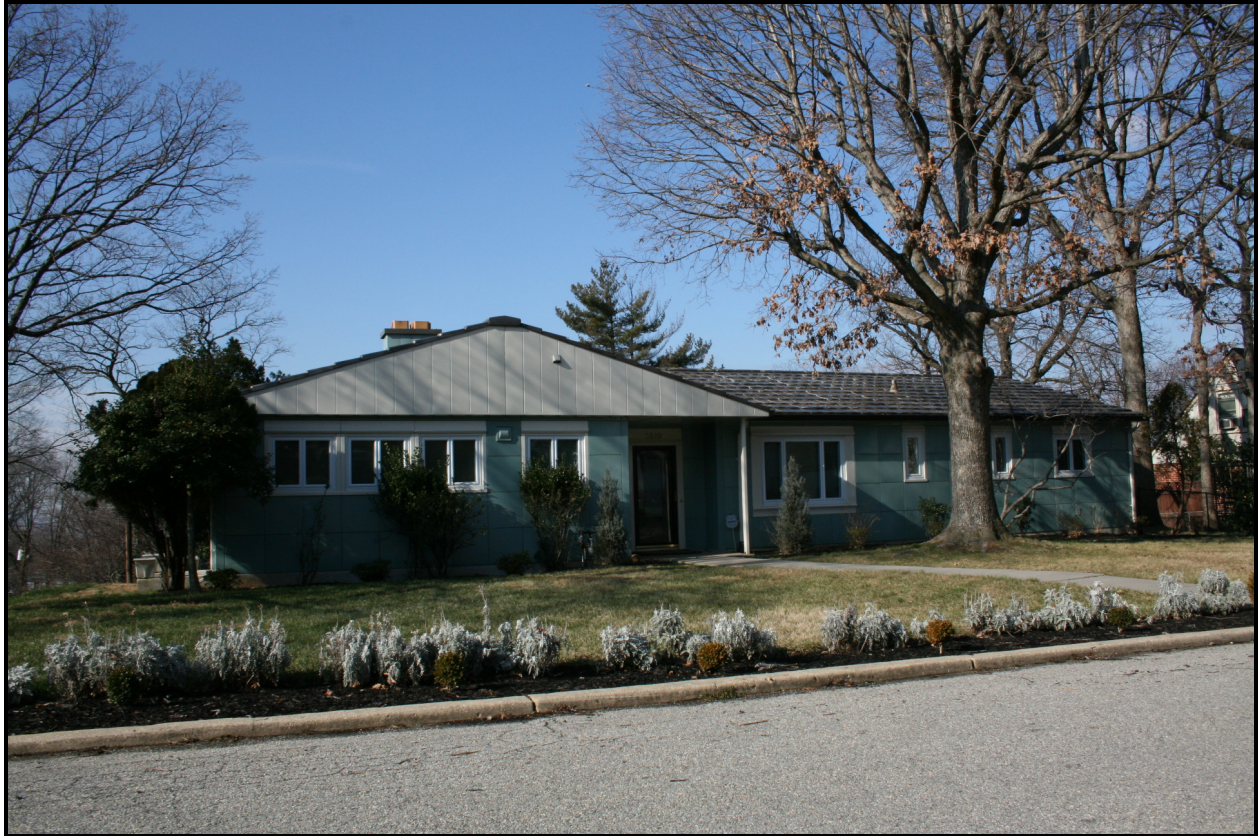
Looking west, 5819 Black Hawk Drive (Lustron house) ( EHT Traceries , 2009)
