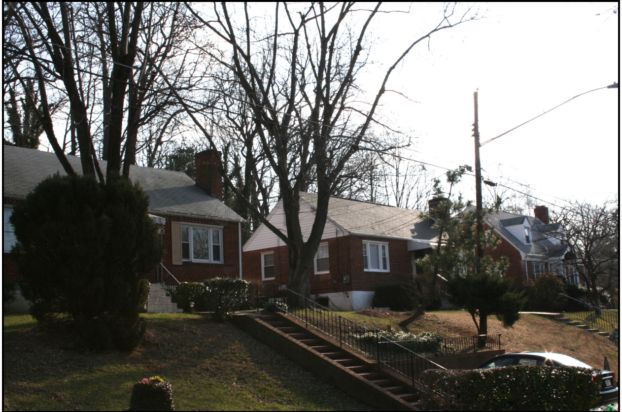
Looking southeast, 5712-5714-5716 Arapahoe Drive ( EHT Traceries , 2009)
