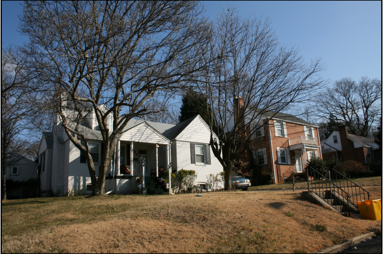
Looking east, 107-105 Rolph Drive ( EHT Traceries , 2009)
