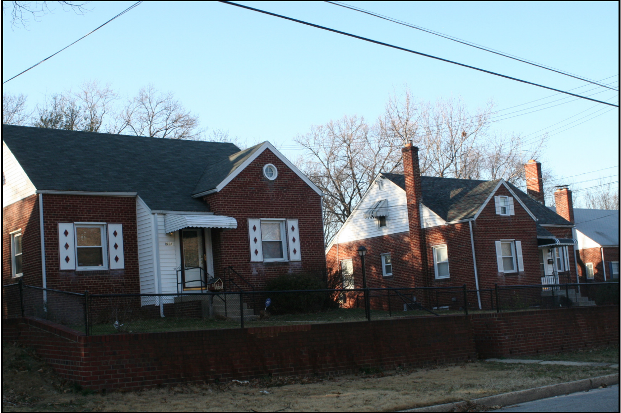
Looking north, 2207-2205 Ramblewood Drive ( EHT Traceries, 2008 )
