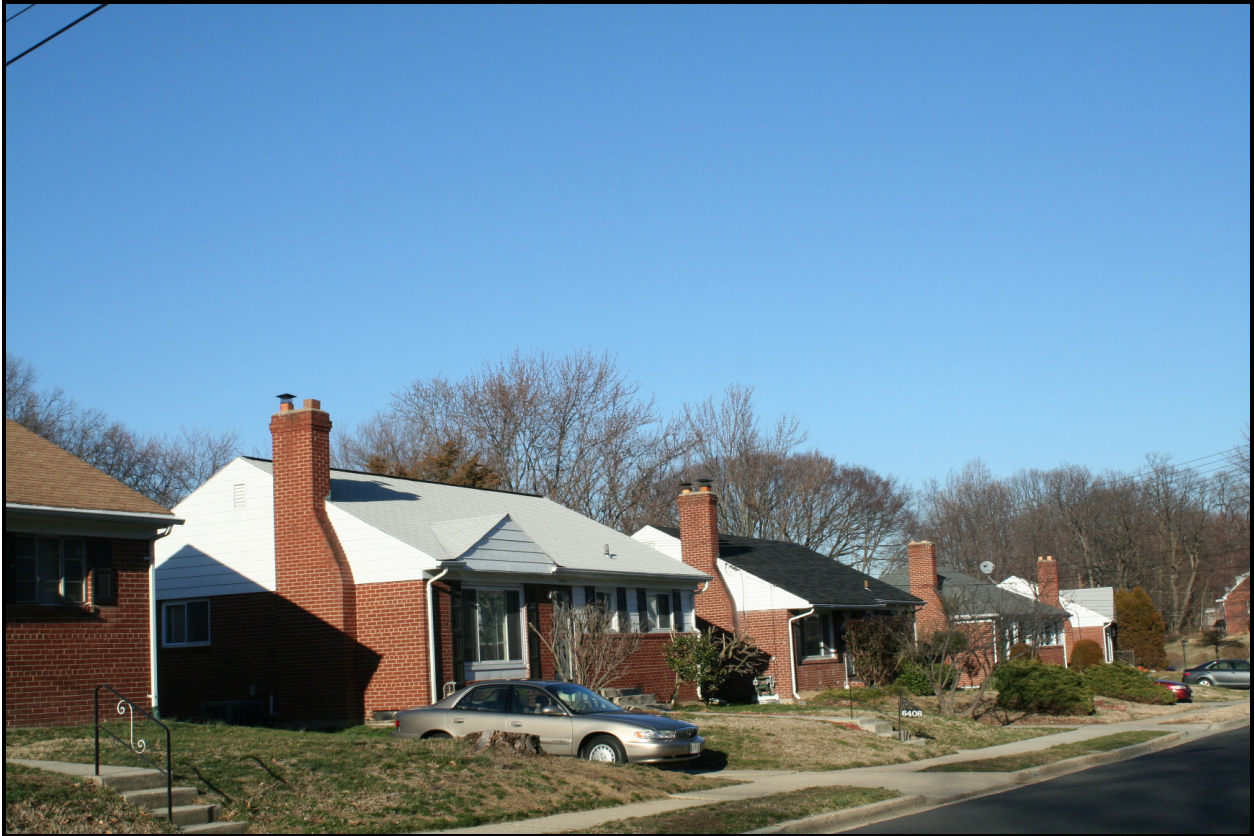
Looking northeast, 6408-6410-6412-6414 Elmhurst Street ( EHT Traceries , 2008)
