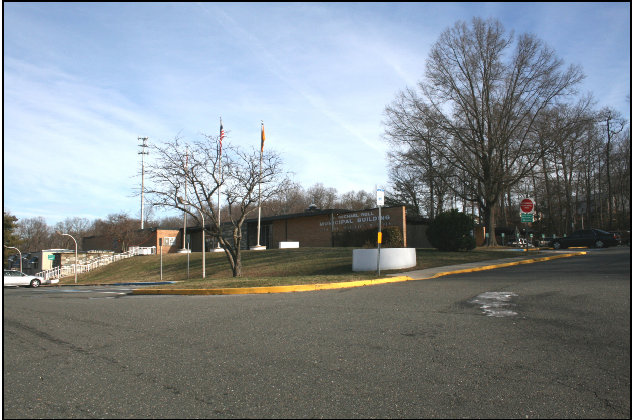
Looking northeast, 2000 Marbury Drive, District Heights Municipal Building ( EHT Tracerics, 2008 )
