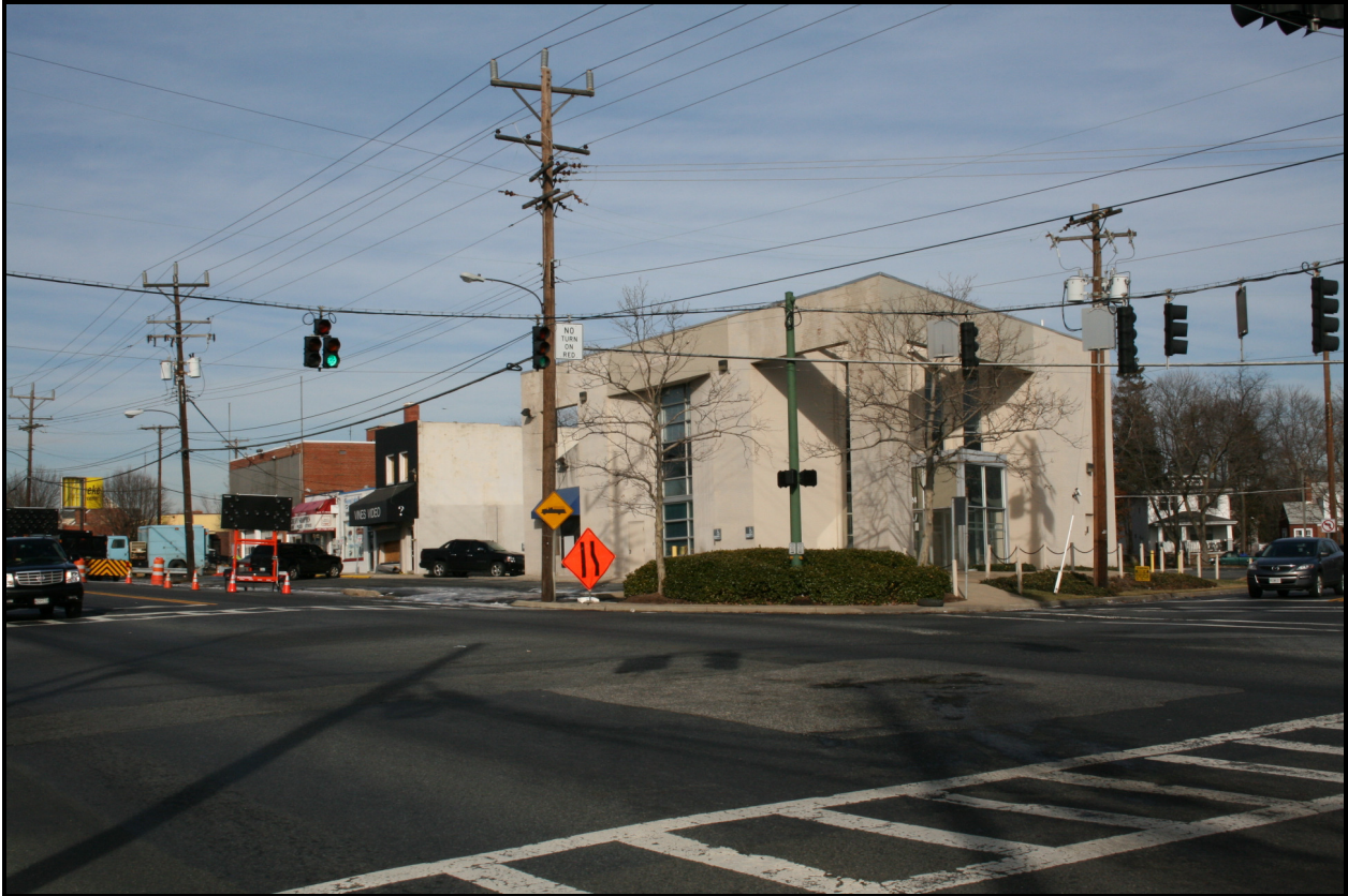
Looking northwest, 6224-6222-6220 Marlboro Pike ( EHT Tracerics, 2008 )
