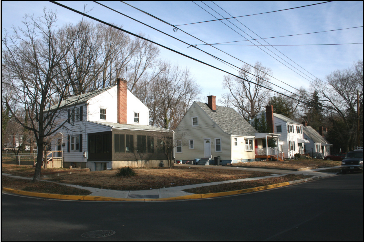
Looking northeast, 6500-6502-6504-6506 Kipling Parkway ( EHT Traceries, 2008 )
