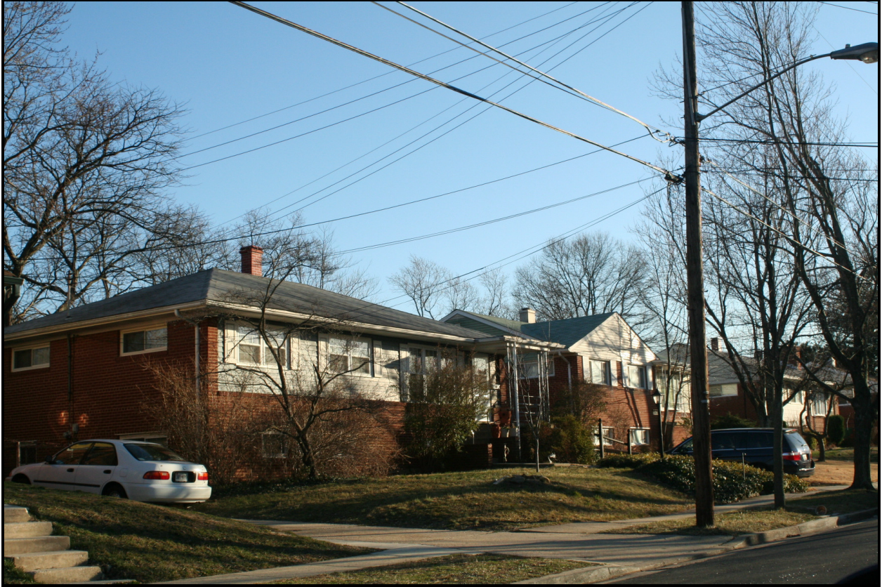
Looking south, 7209-7207 Lansdale Street ( EHT Traceries, 2008 )
