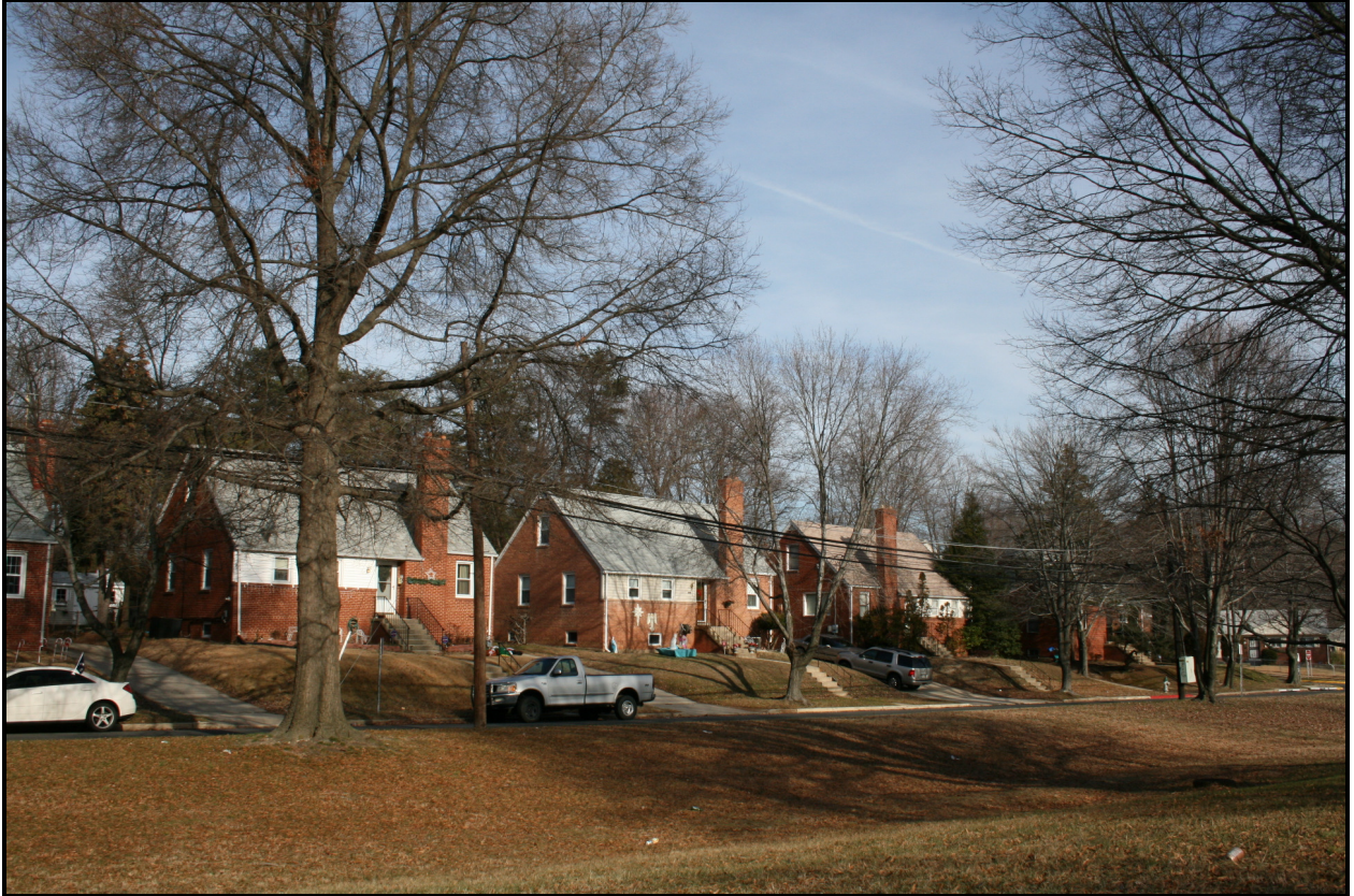
Looking northeast, 6714-6716-6718 Kipling Parkway ( EHT Traceries , 2008)
