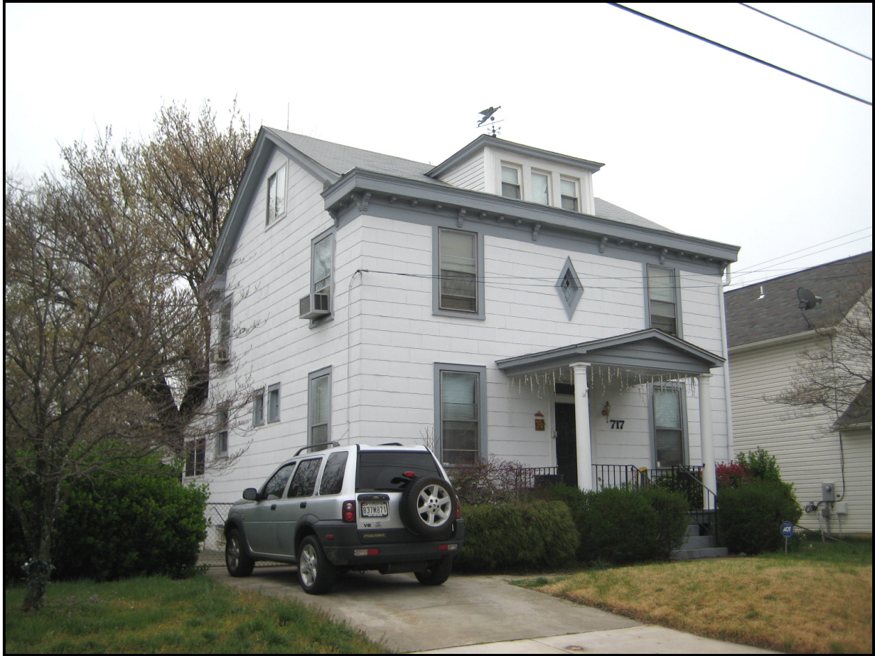
Looking southeast, 717 59th Avenue, John Trammell/Judge James Taylor House ( EHT Traceries , 2008)
