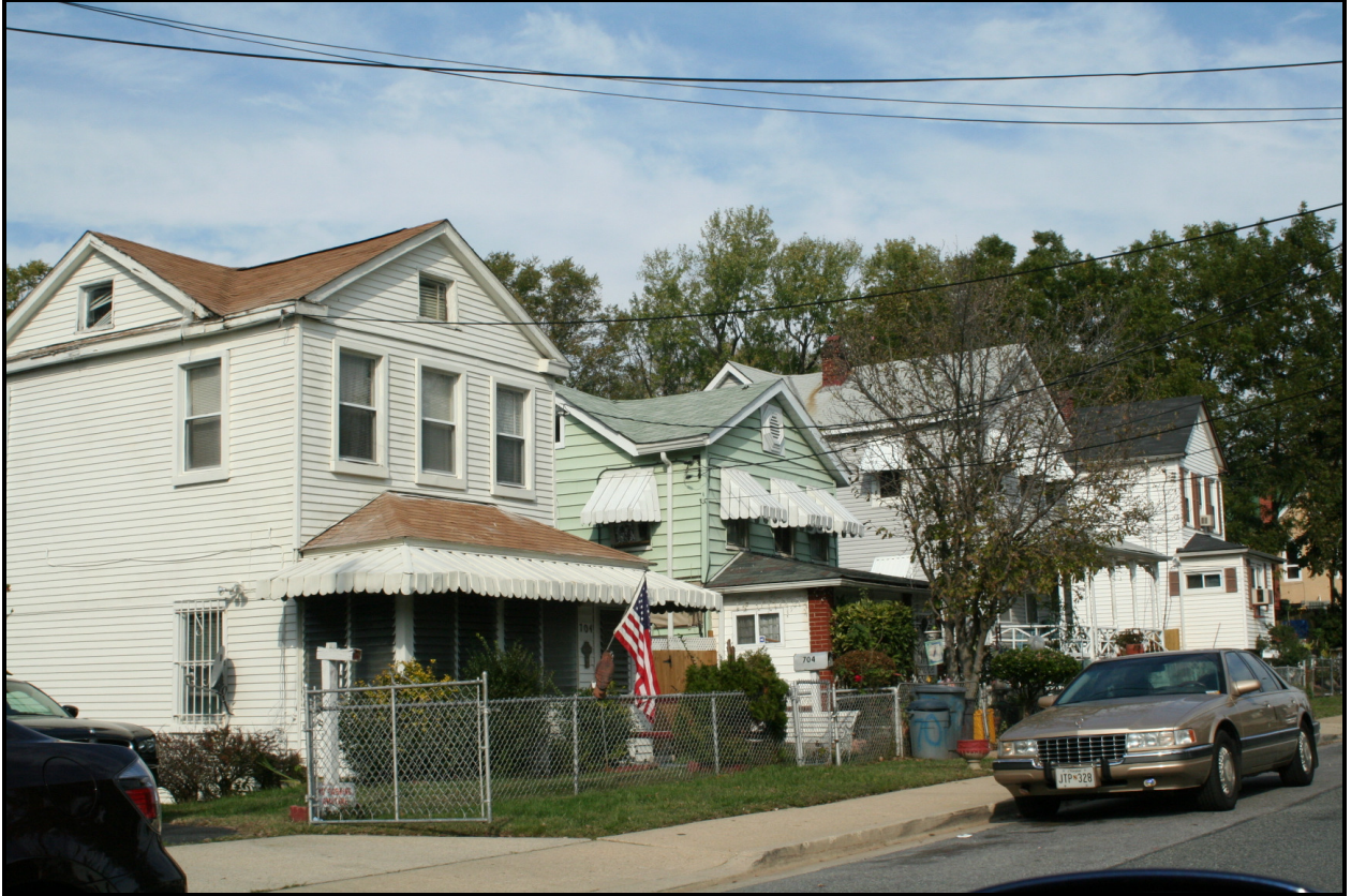
Looking north, 704-710 59th Avenue ( EHT Traceries , 2007)
