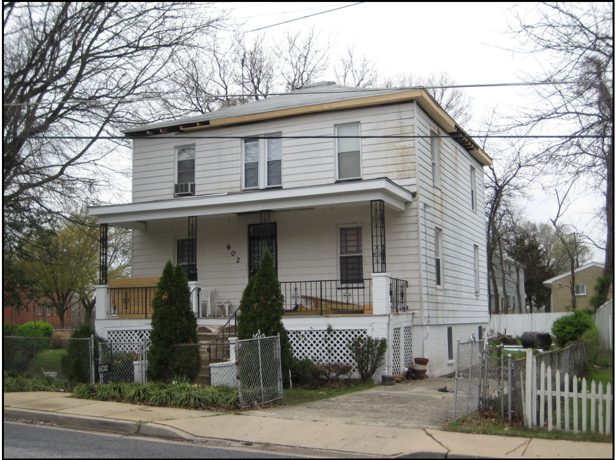
Looking west, 602 60th Place, Cornelius Fonville House ( EHT Traceries , 2008)
