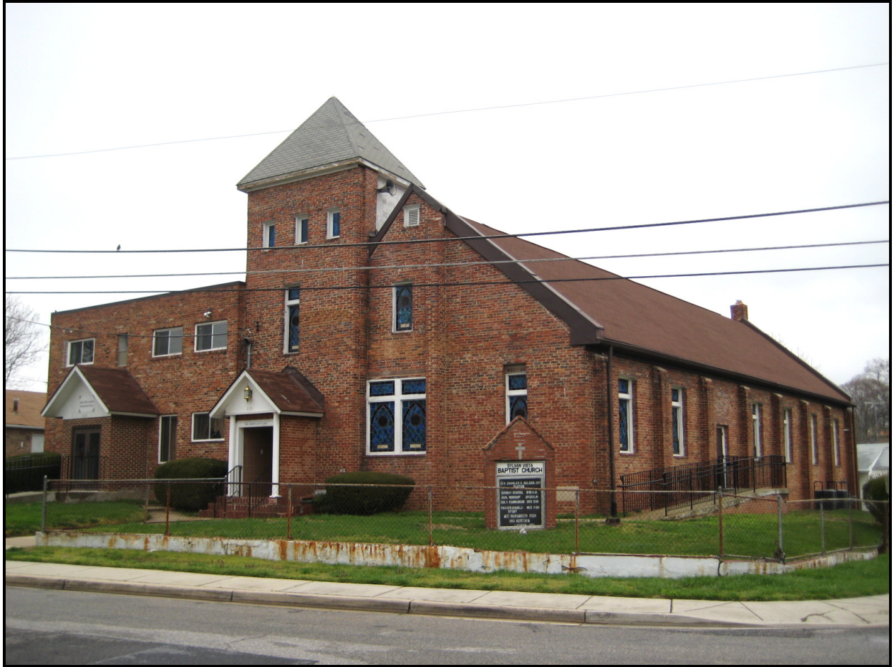
Looking northeast, 1101 60th Avenue, Sylvan Vista Baptist Church ( EHT Traceries, 2008 )
