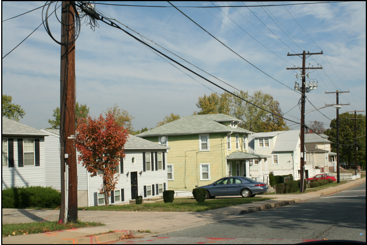
Looking north, 706-708-710 59th Avenue ( EHT Tracerics , 2007)
