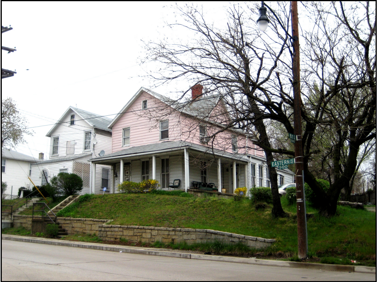
Looking north, 505 Eastern Avenue, William Sidney and Portia Washington Pittman House ( EHT Traceries , 2008)
