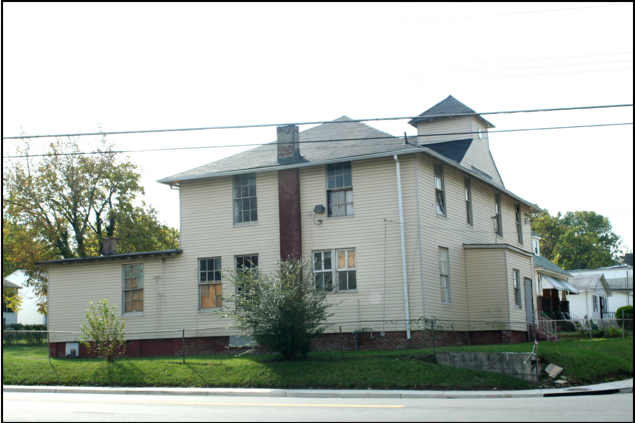
Looking southeast, 737 61st Avenue, Fairmount Heights School (PG: 72-009-09) ( EHT Traceries, 2007 )
