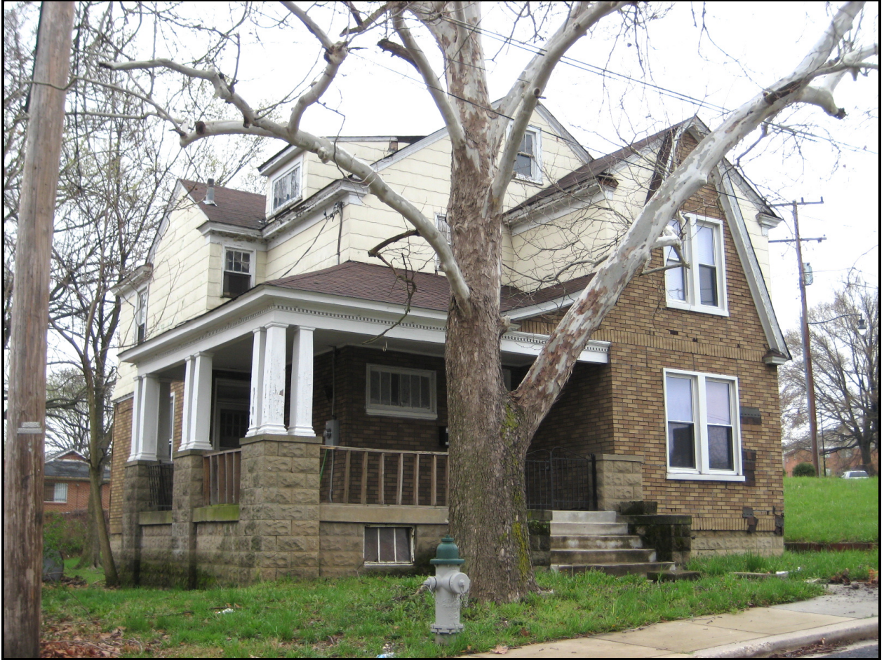
Looking southeast, 701 58th Avenue, Louis Brown House ( EHT Traceries , 2008)
