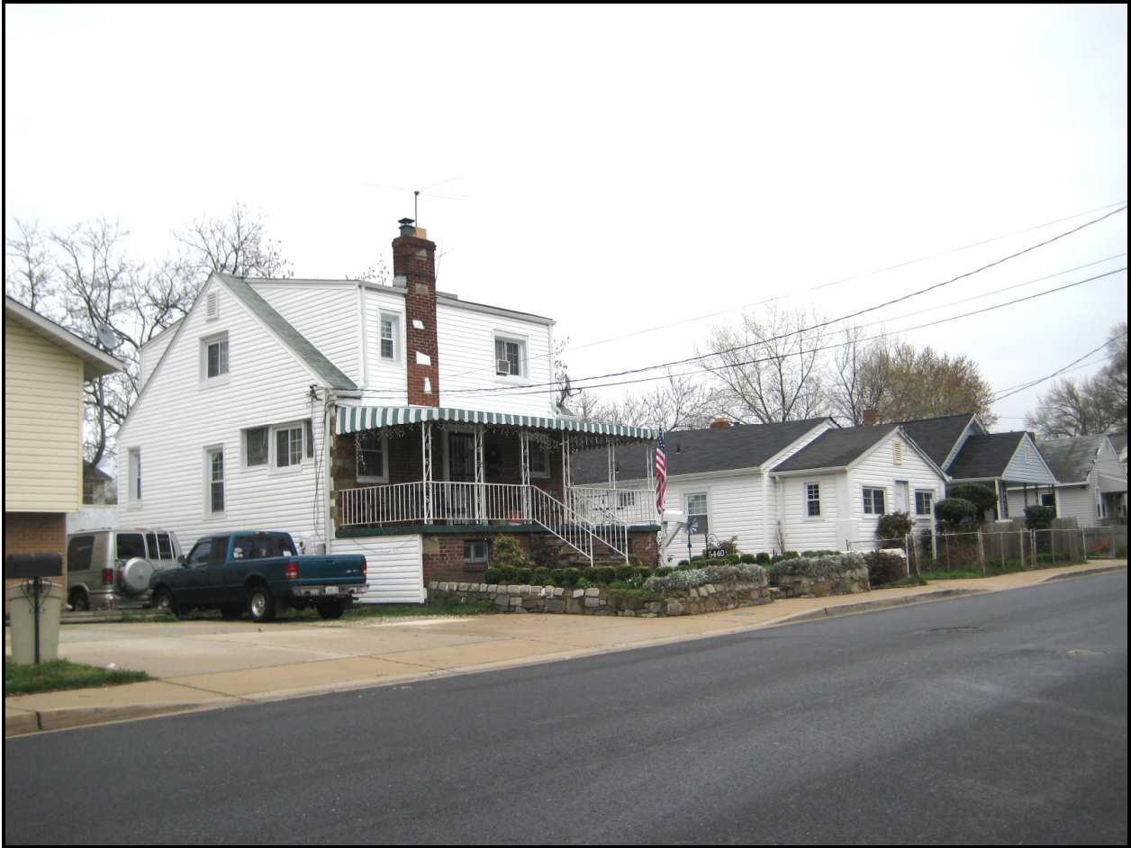
Looking southeast, 5438-5440 Addison Road ( EHT Traceries , 2008)
