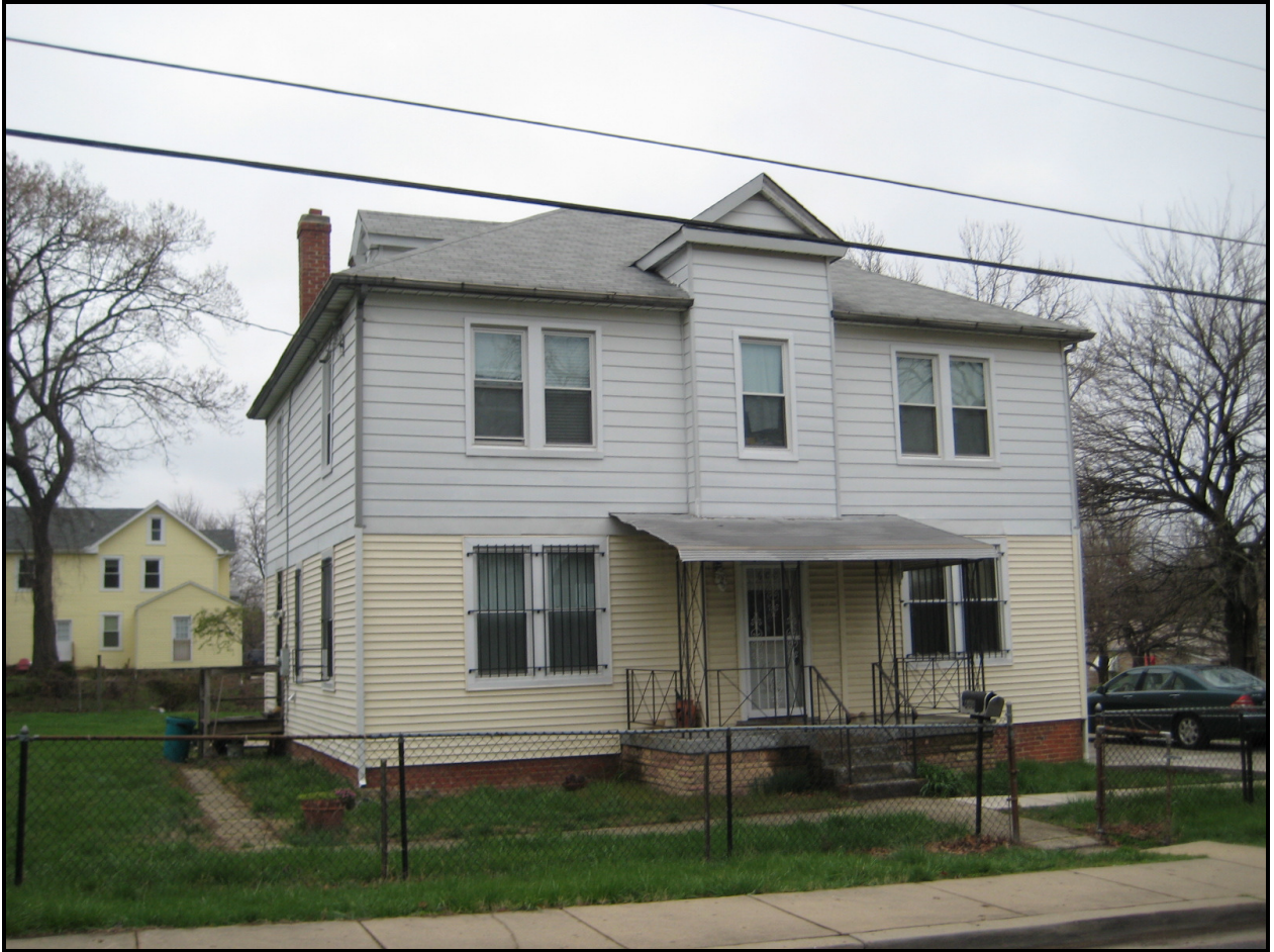
Looking north, 608 60th Place, Henry Pinckney House ( EHT Traceries , 2008)
