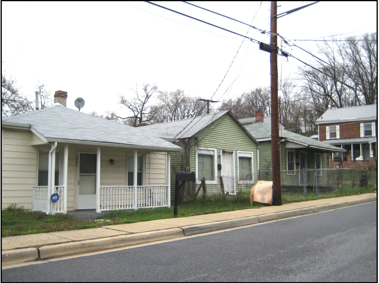
Looking northeast, 5502-5504-5506 Jefferson Heights Drive ( EHT Traceries, 2008 )
