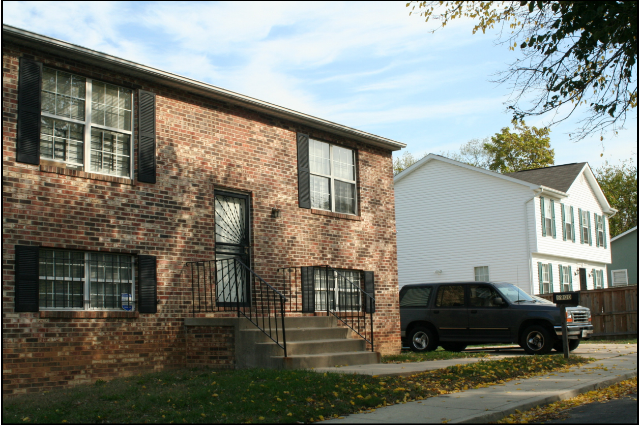
Looking northeast, 5900-5902 J Street ( EHT Traceries , 2007)
