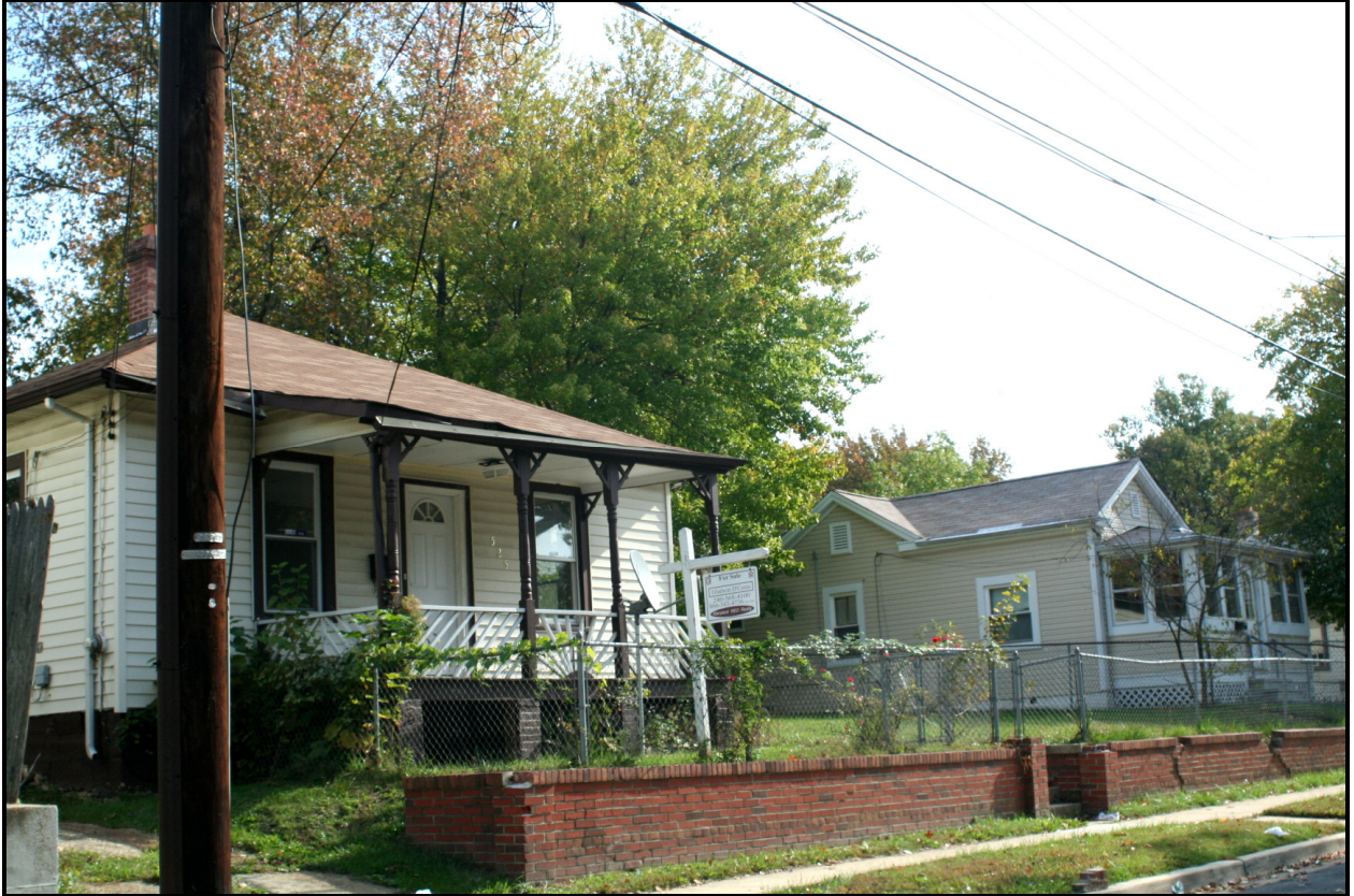
Looking southeast, 525-523 68th Street ( EHT Traceries, 2007 )
