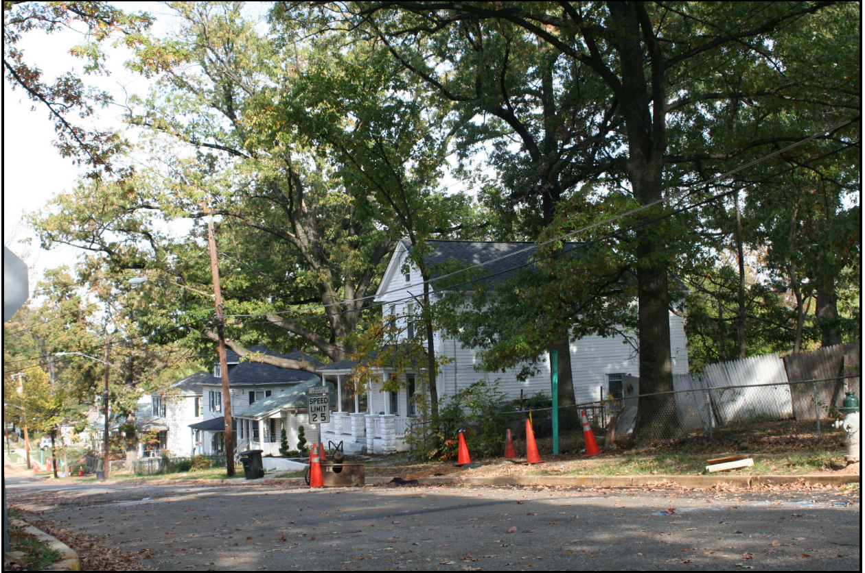
Looking northwest, 505-507-509-511 68th Place ( EHT Traceries, 2007 )
