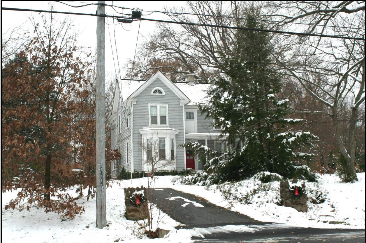
Looking south, Van Horn House (PG: 70-052-26), 10911 Prospect Hill Road ( EHT Traceries , 2007)
