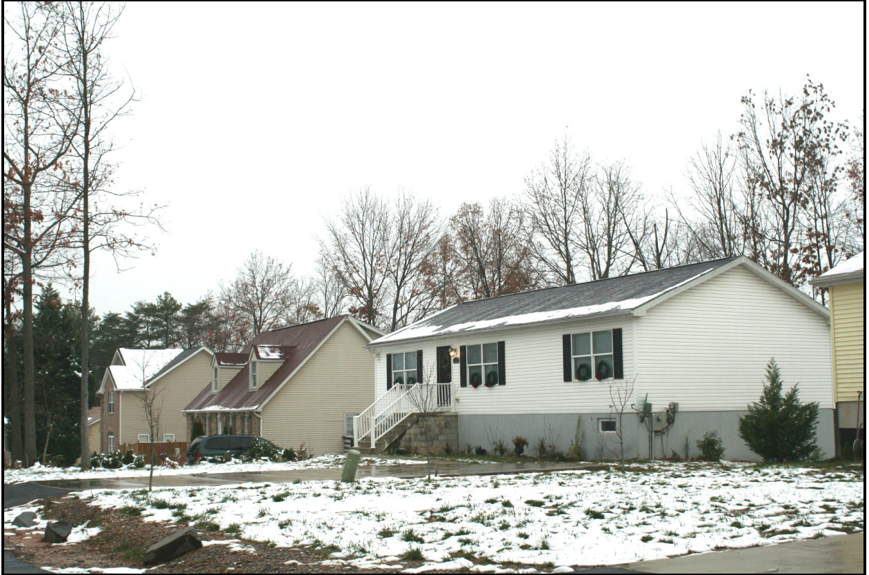
Looking east, 9714-9712-9706 Maryland Street ( EHT Traceries, 2007 )
