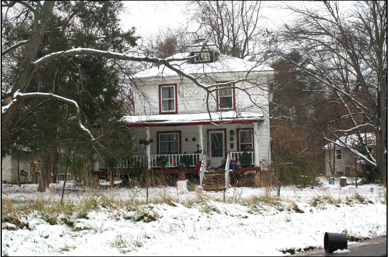
Looking south, Thomas J. Calloway House (PG: 70-049-33) (NR), 9949 Elm Street ( EHT Traceries , 2007)
