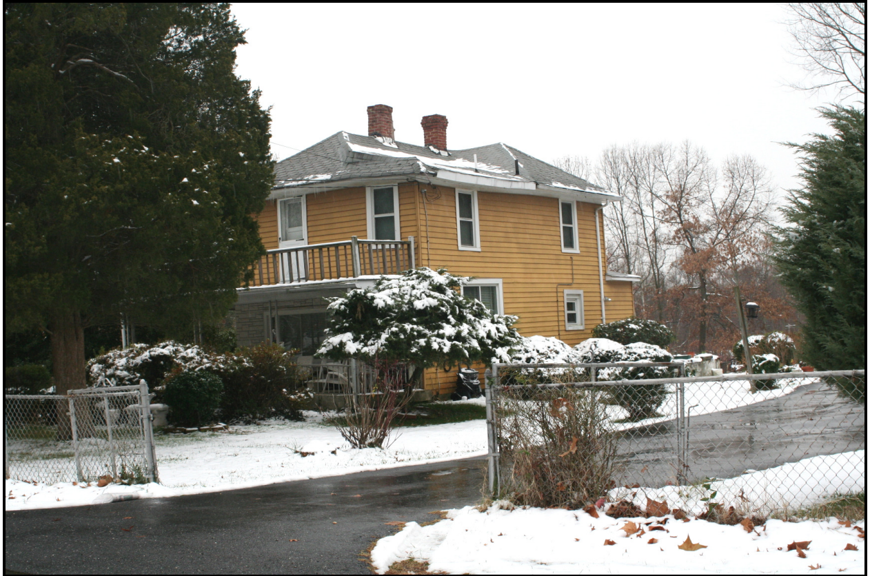
Looking southwest, 5500 Lincoln Street ( EHT Traceries , 2007)
