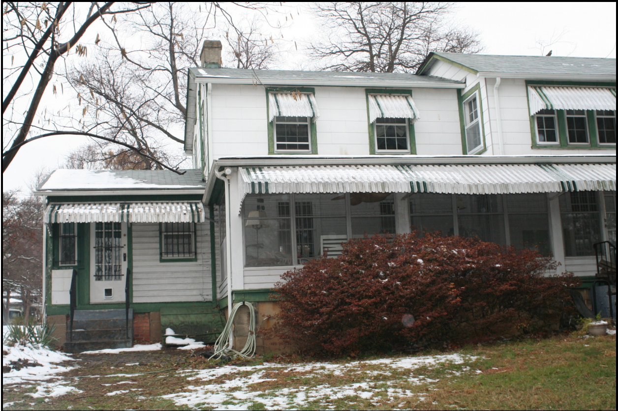
Looking west, Wormley House (PG: 69-023-17), 7533 Ardwick-Ardmore Road ( EHT Traceries , 2007)
