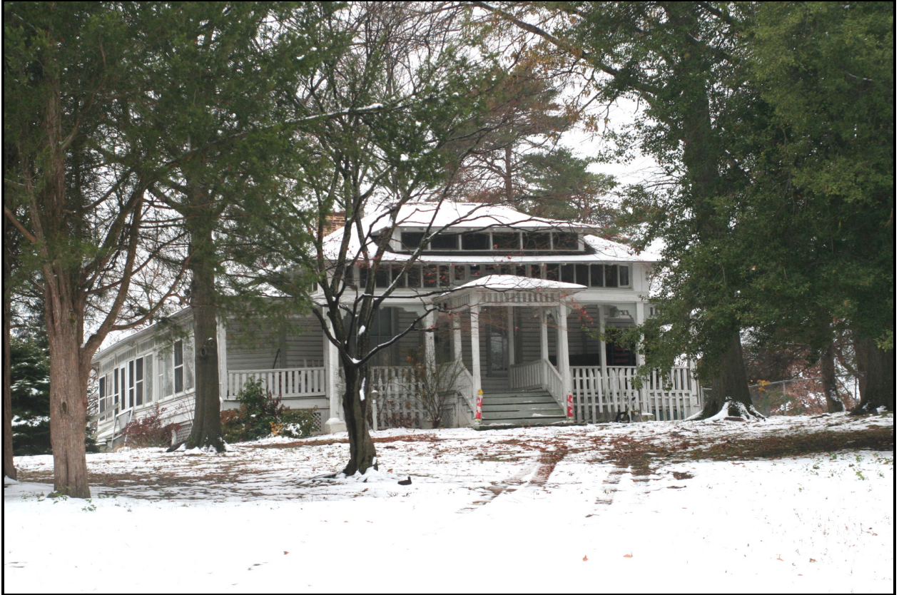
Looking west, Thomas W. Hunster House (PG: 69-023-27), 7523 Ardwick-Ardmore Road ( EHT Traceries , 2007)
