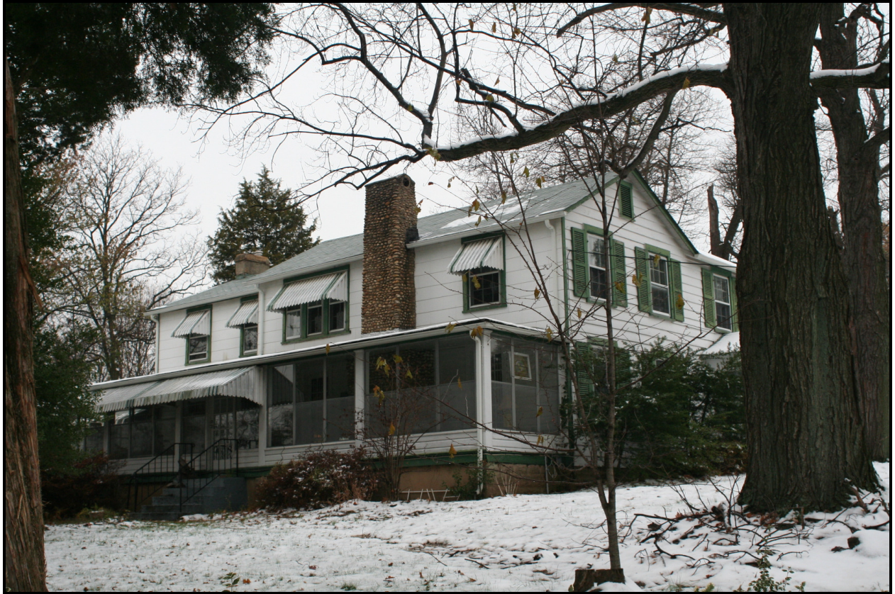
Looking southwest, Wormley House (PG: 69-023-17), 7533 Ardwick-Ardmore Road ( EHT Traceries , 2007)
