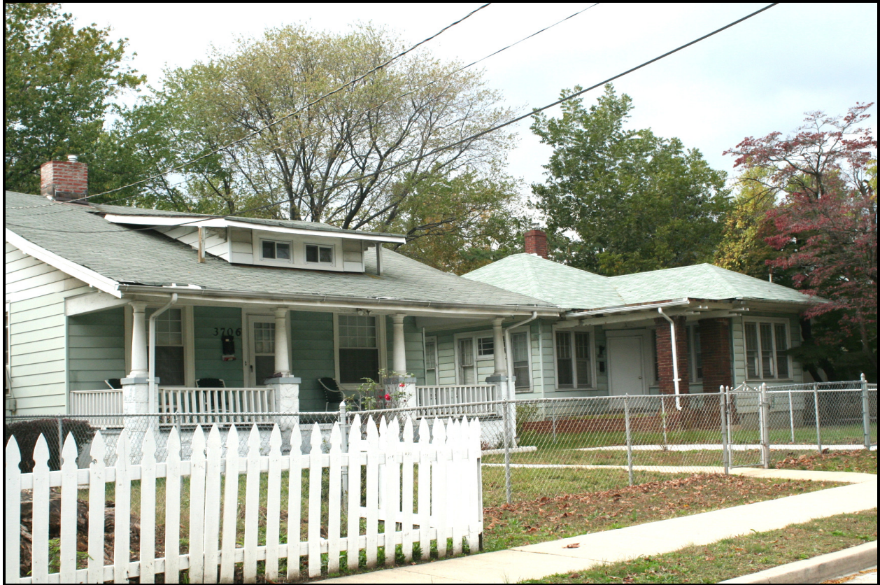
Looking northwest, 3706-3708 41st Avenue ( EHT Traceries , 2007)
