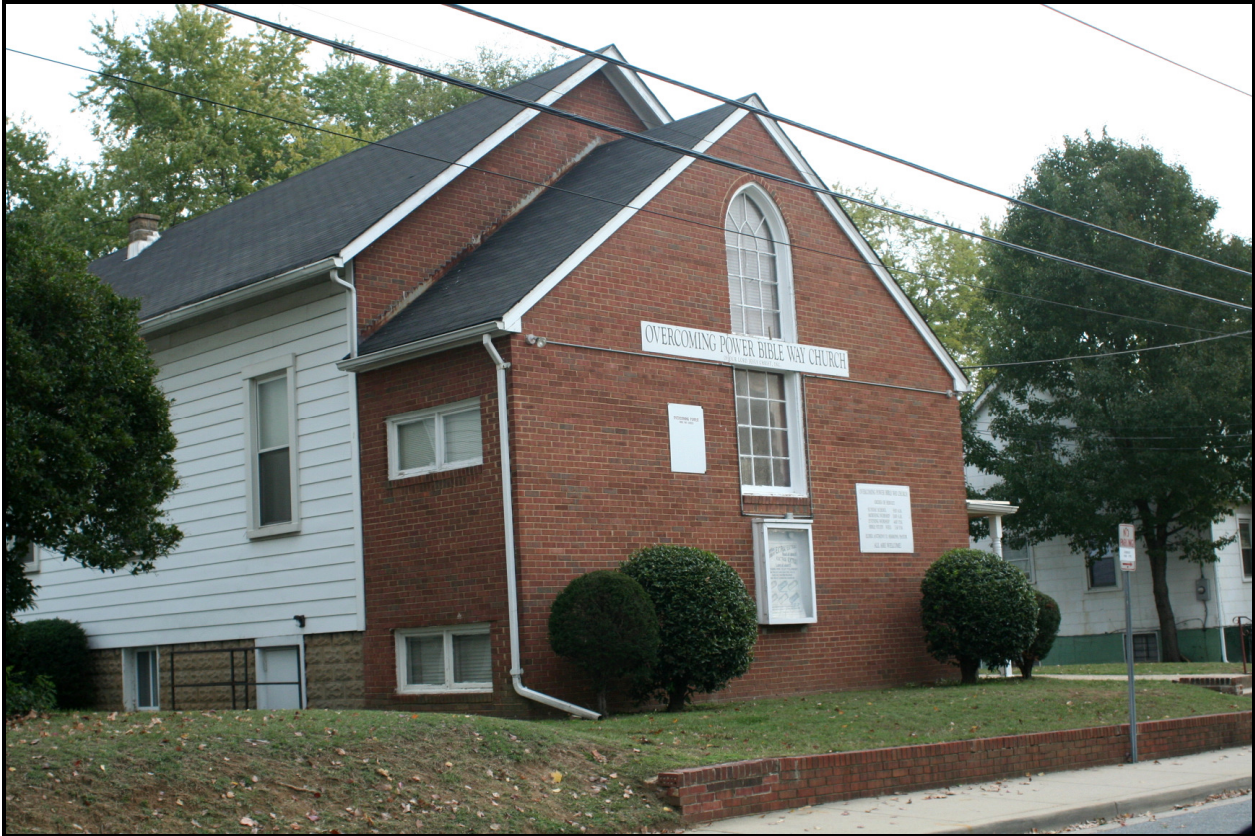
Looking east, 3713 42nd Avenue, Overcoming Power Bible Way Church ( EHT Traceries, 2007 )
