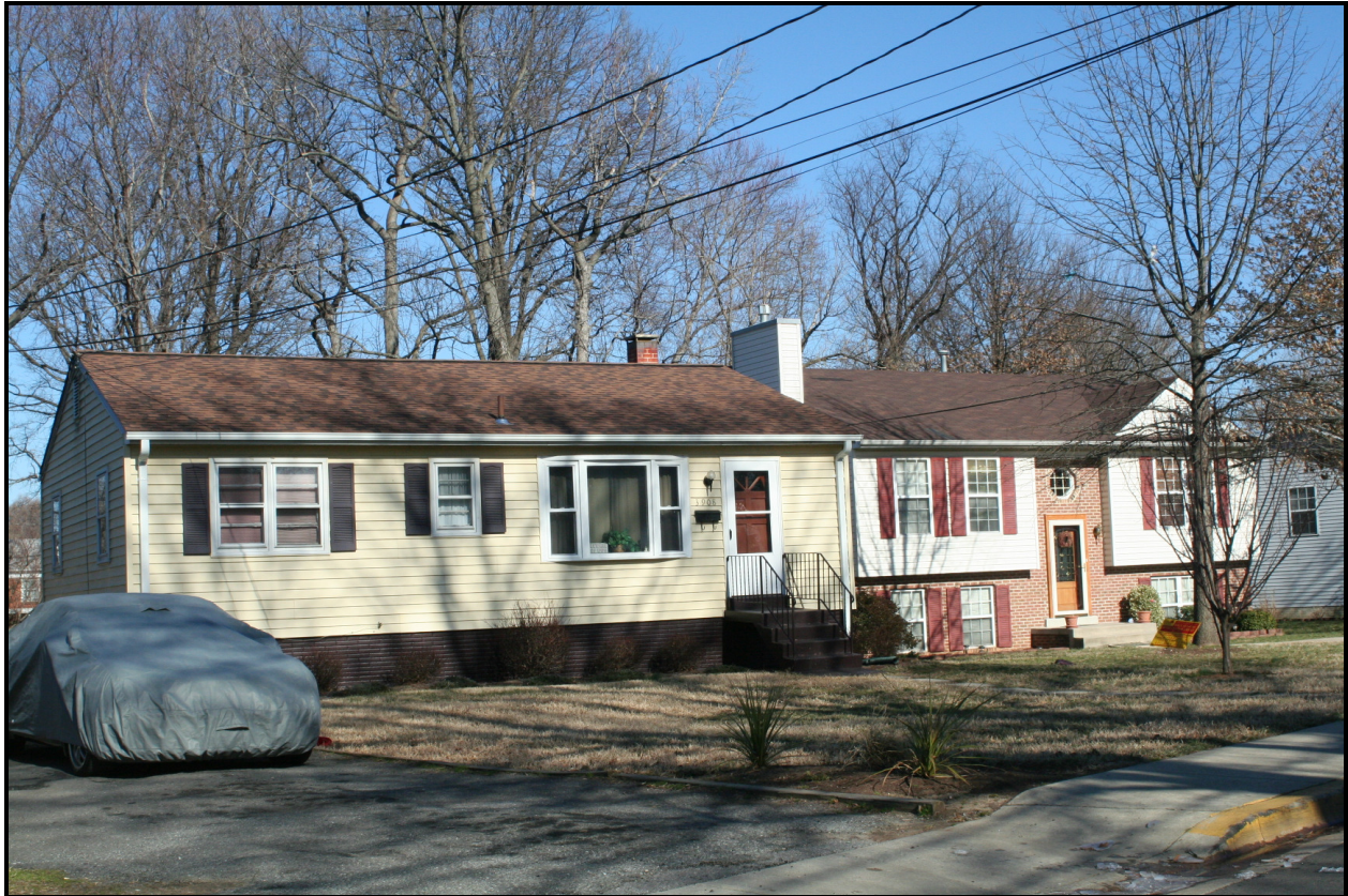
Looking northeast, 3908-3910 Windom Road ( EHT Traceries , 2008)
