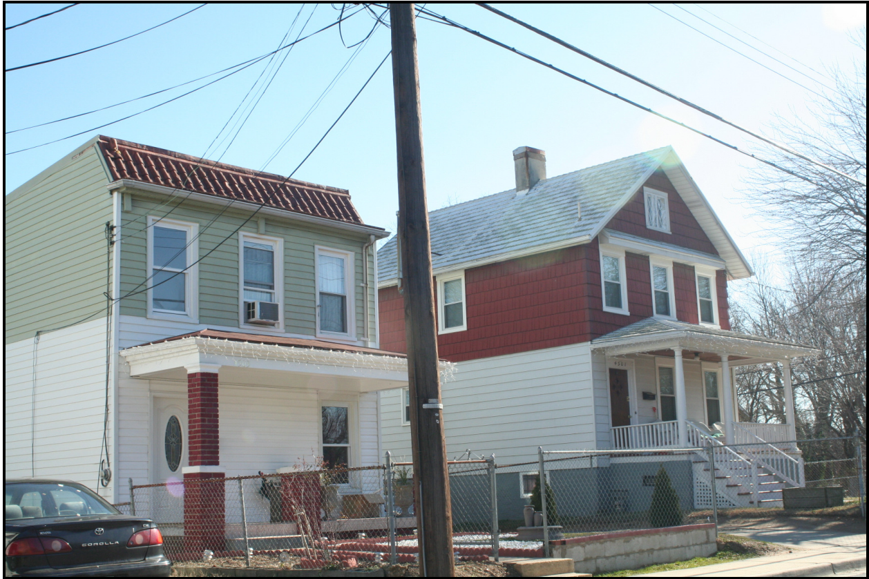
Looking south, 4503-4501 40th Street ( EHT Traceries, 2008 )
