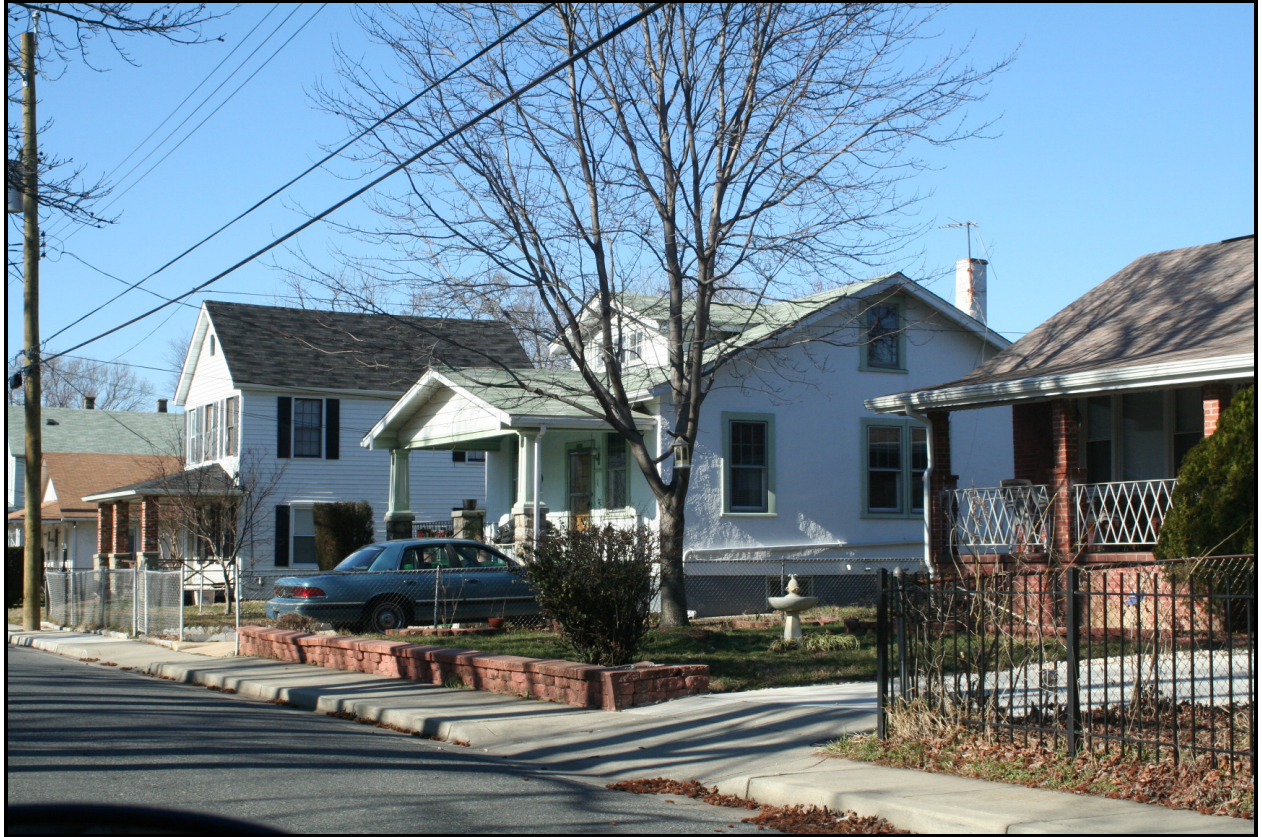
Looking northwest, 3920-3918 Allison Street ( EHT Traceries, 2008 )
