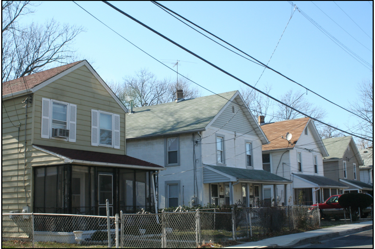
Looking west, 4021-4019-4017-4015 Webster Street ( EHT Traceries , 2008)
