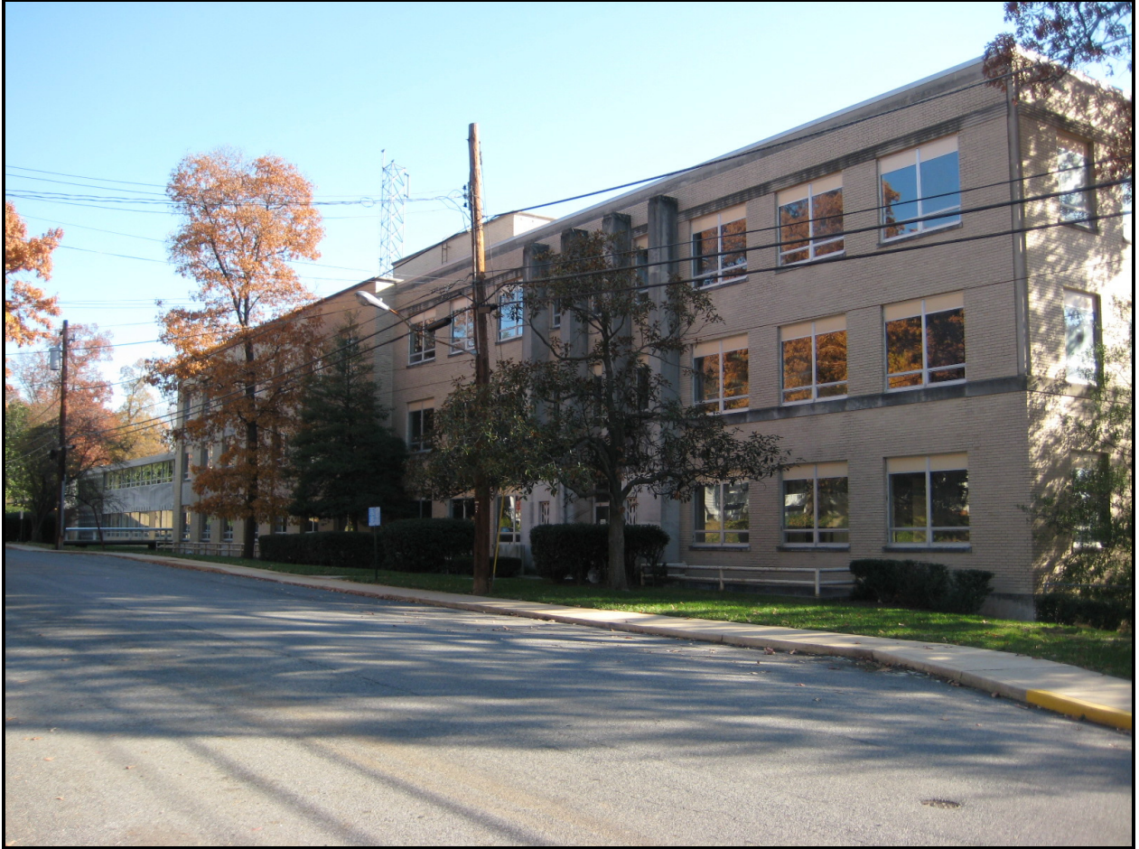
Looking southeast, 4017 Hamilton Street, Washington Suburban Sanitary Commission ( EHT Tracerics, 2007 )
