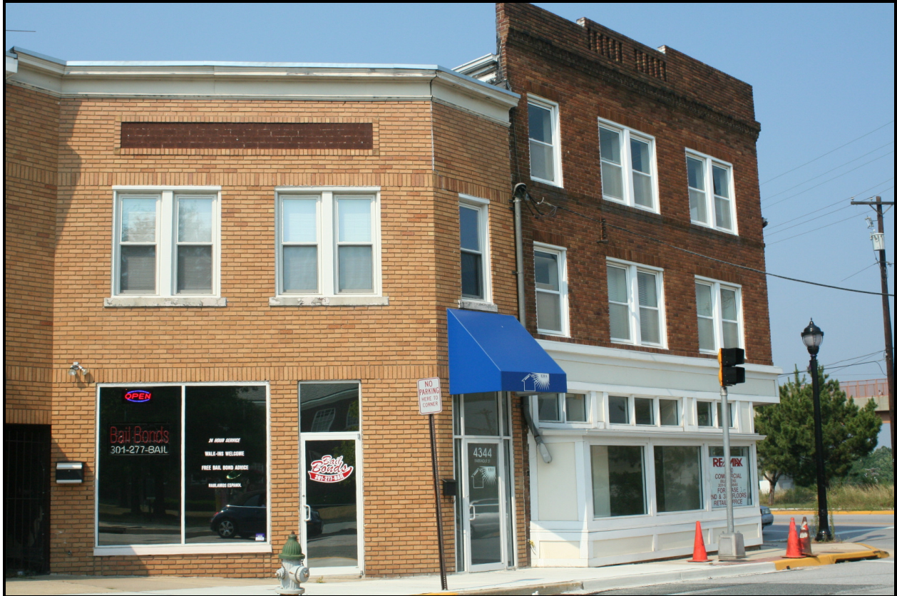
Looking north, 4344 Farragut Street and 5108 Baltimore Avenue ( EHT Traceries, 2007 )
