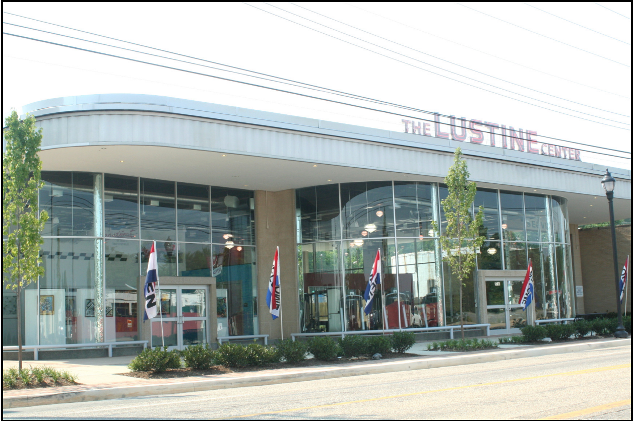
Looking northwest, 5710 Baltimore Avenue, The Lustine Center ( EHT Traceries, 2007 )
