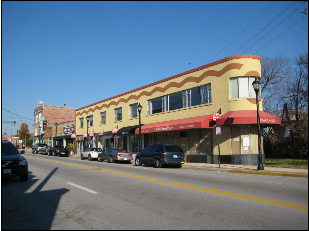
Looking northeast, Magruder Flatiron Building (PG: 68-041-14), 5101 Baltimore Avenue ( EHT Traceries , 2007)
