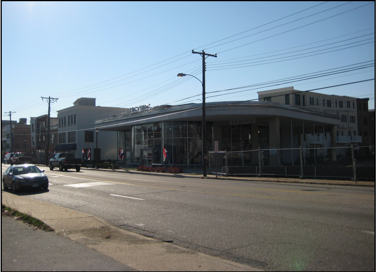
Looking southwest, 5710 Baltimore Avenue, The Lustine Center ( EHT Tracerics, 2007 )
