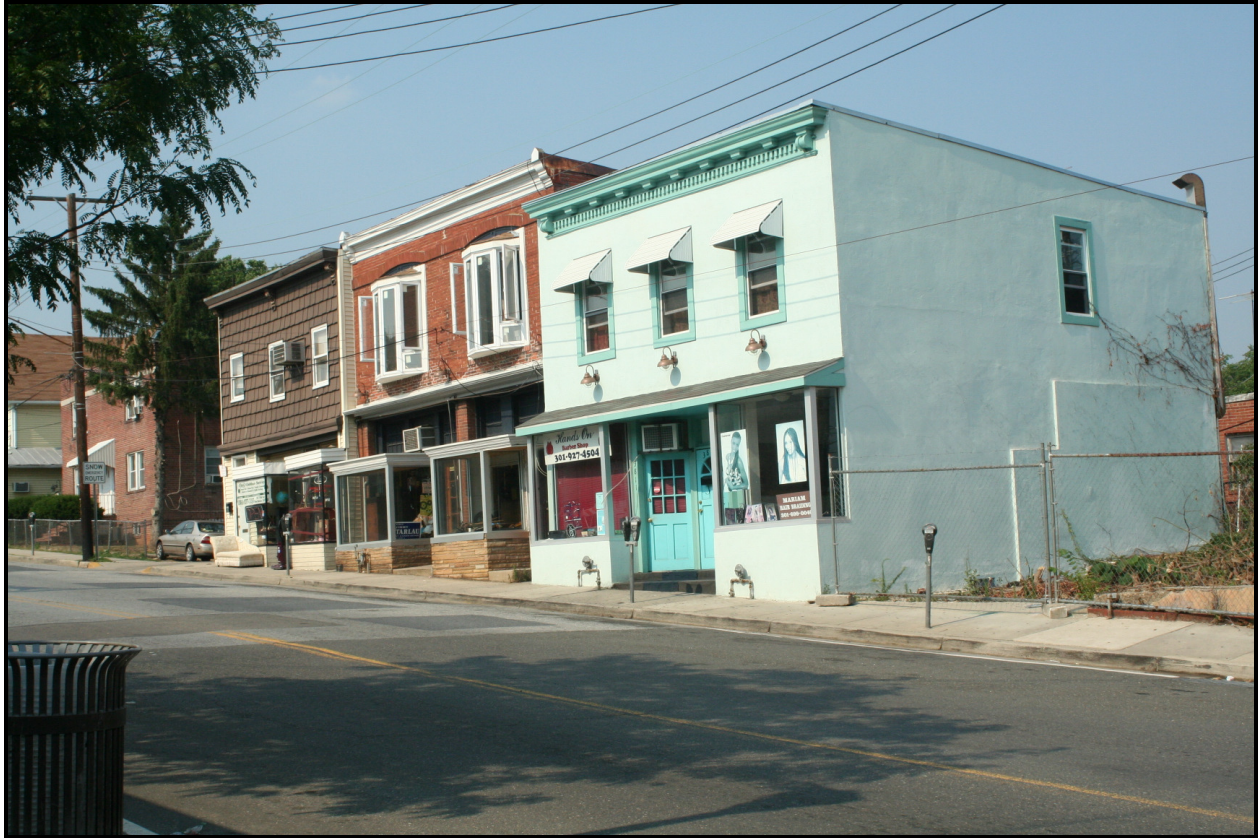
Looking northeast, 3807-3815-3817 34th Street ( EHT Traceries, 2007 )
