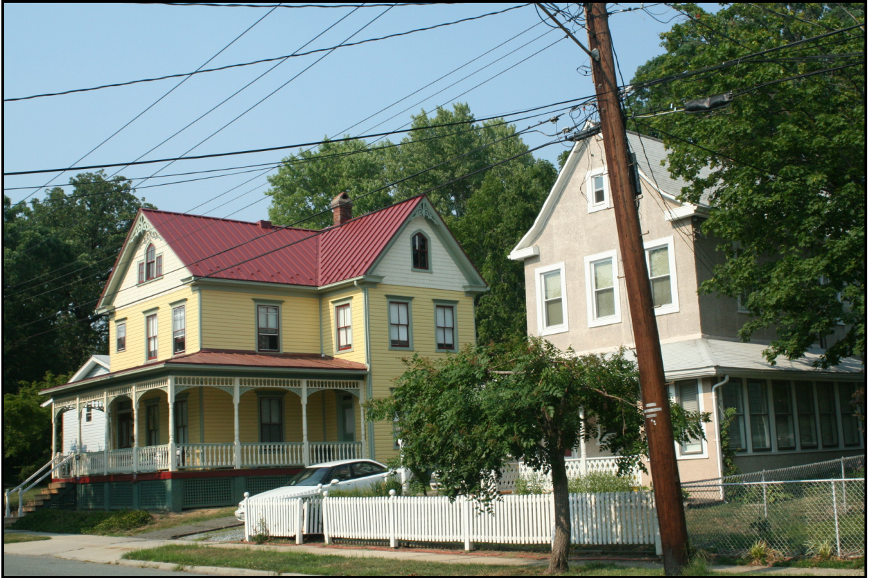
Looking southeast, 4013-4011 30th Street ( EHT Traceries , 2007)
