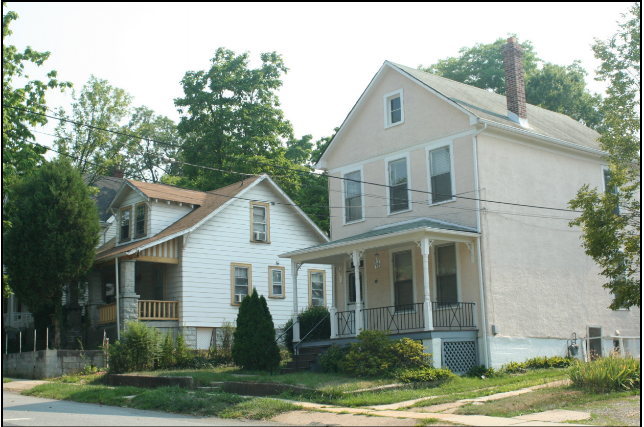
Looking south, 4112-4110 33rd Street ( EHT Traceries , 2007)
