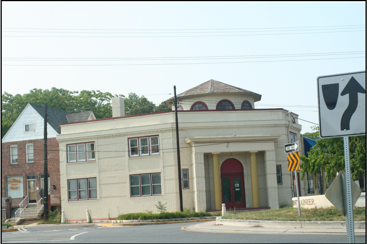
Looking northwest, Prince George's Bank (PG: 68-013-02), 3800 34th Street ( EHT Tracerics, 2007 )
