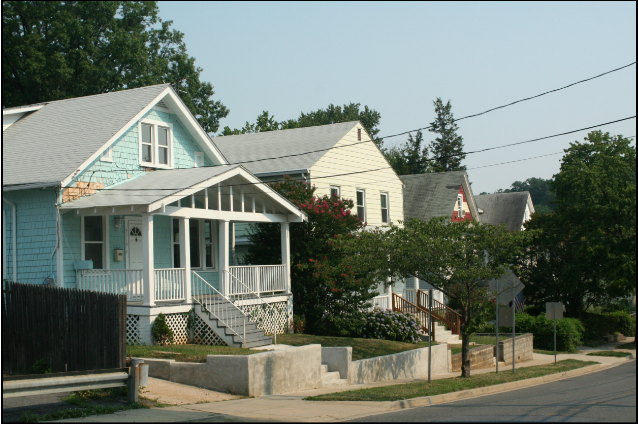
Looking southeast, 3719-3713 34th Street ( EHT Traceries , 2007)
