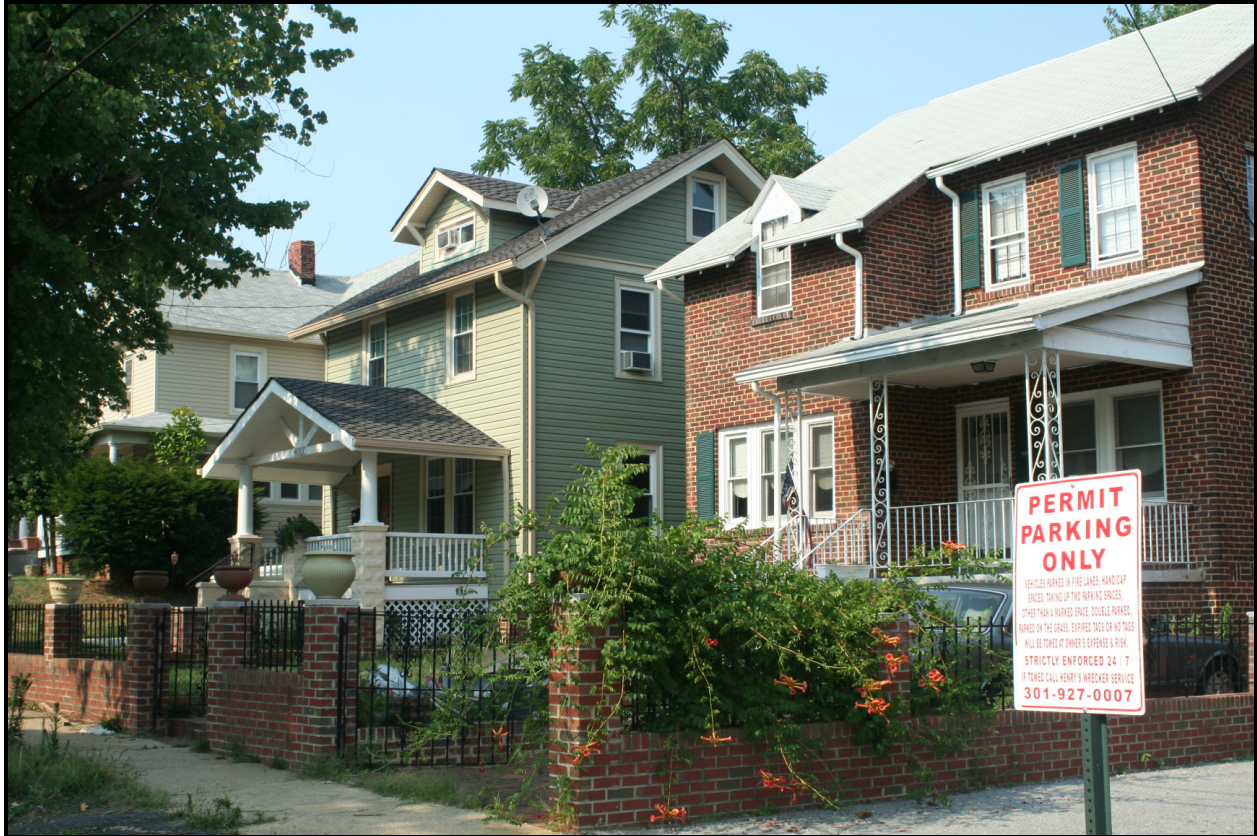
Looking northeast, 4005-4007-4009 29th Street ( EHT Traceries, 2007 )
