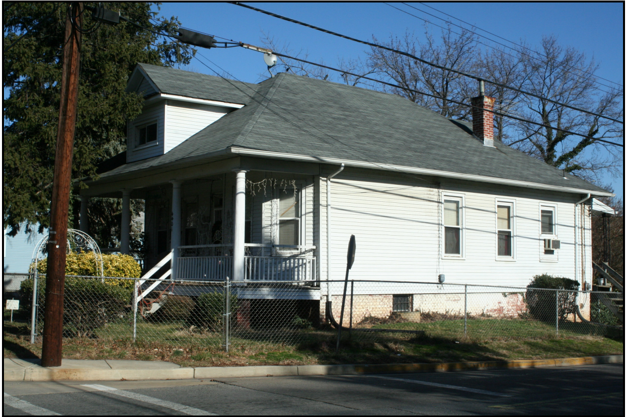
Looking northeast, 4401 40th Street ( EHT Traceries, 2008 )
