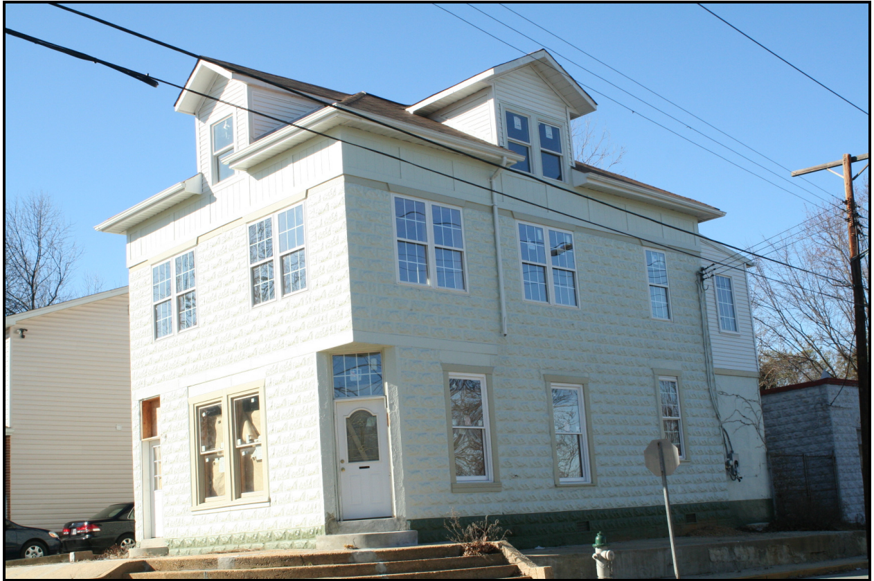
Looking northwest, 4204 37th Street ( EHT Traceries , 2008)
