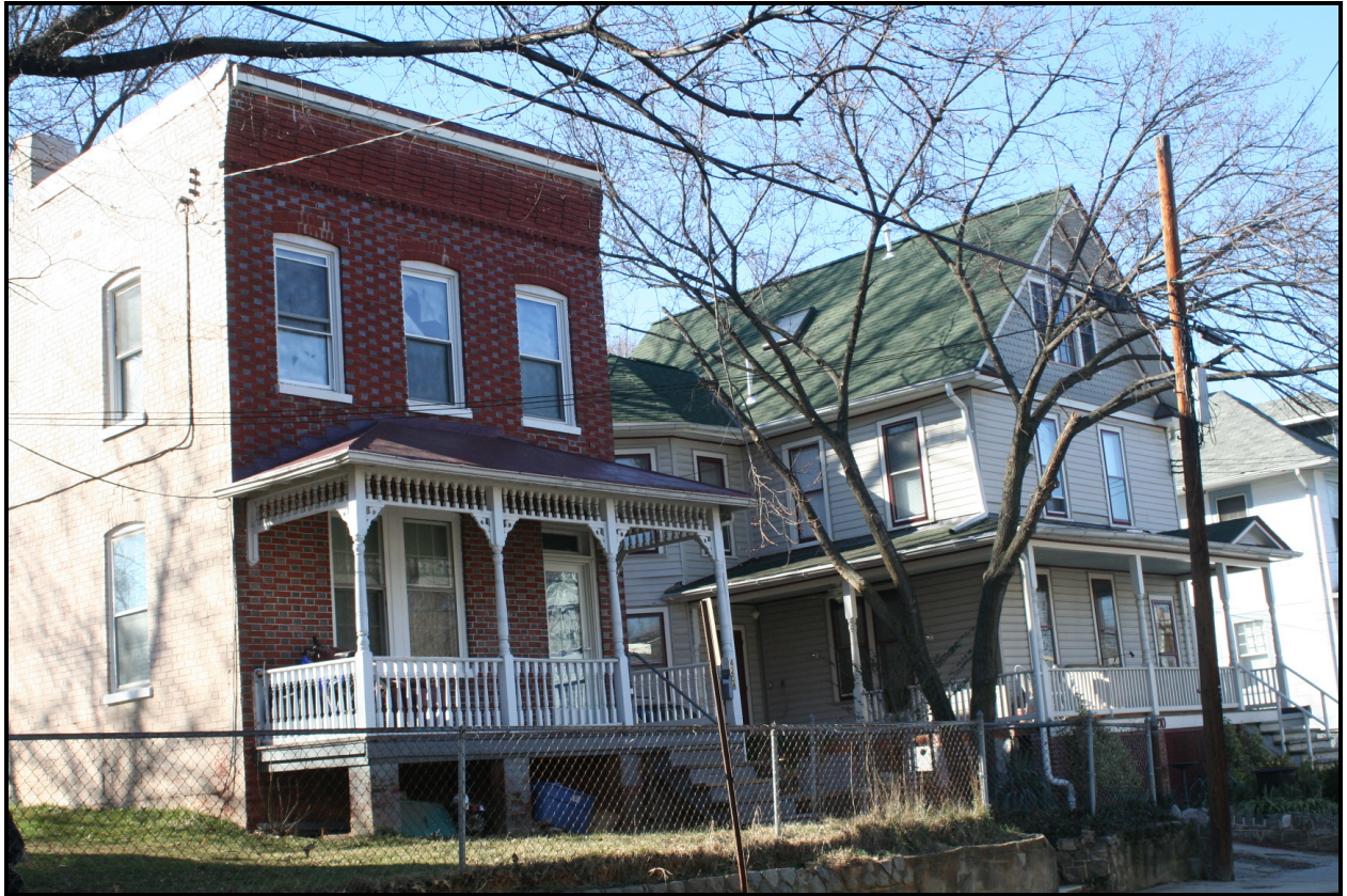
Looking northwest, 4208-4210 34th Street ( EHT Traceries , 2008)
