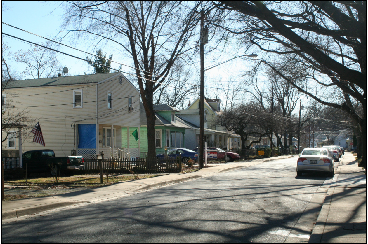
Looking south, 4313-4311-4309 40th Street ( EHT Traceries , 2008)
