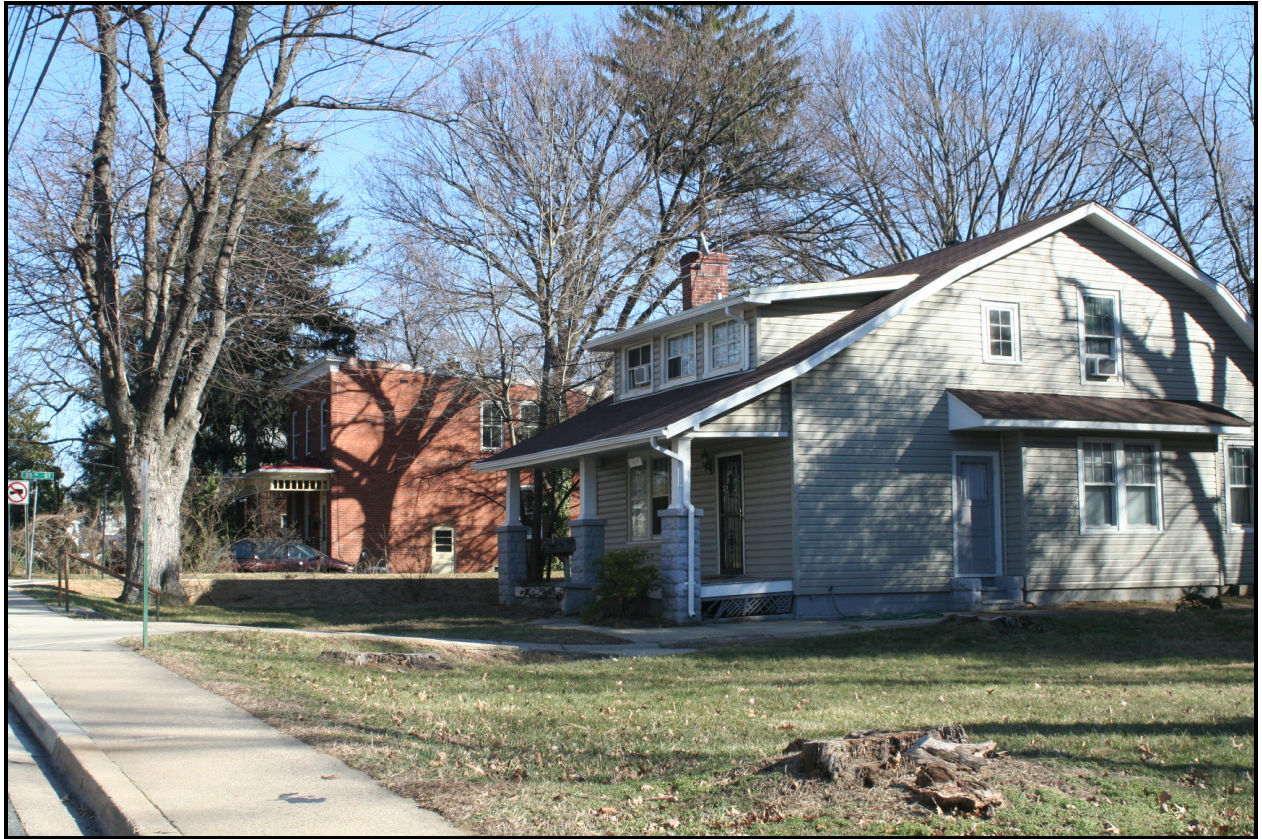
Looking southeast, 3413-3503 Webster Street ( EHT Traceries, 2008 )
