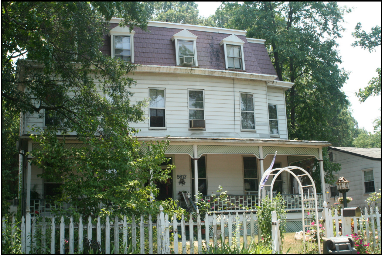
Looking northeast, 5617 Ruatan Street, Wolfe House (PG: 67-022-025) ( EHT Traceries , 2007)
