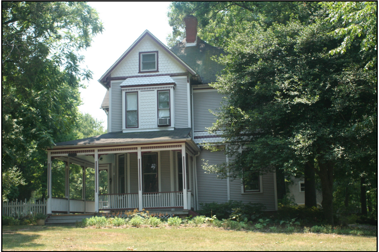
Looking southwest, 5805 Ruatan Street, Cross House (PG: 67-022-013) ( EHT Traceries , 2007)
