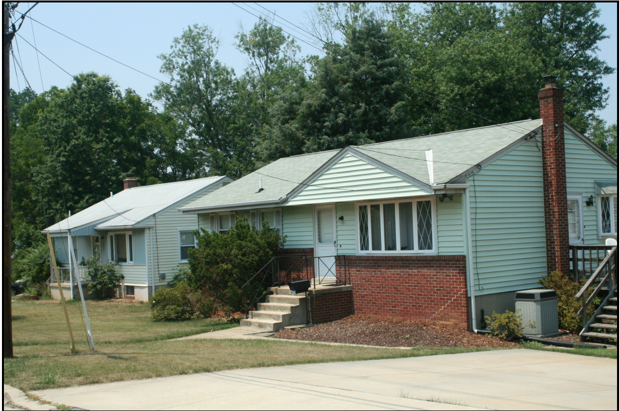
Looking west, 5612-5610 Seminole Street ( EHT Traceries, 2007 )
