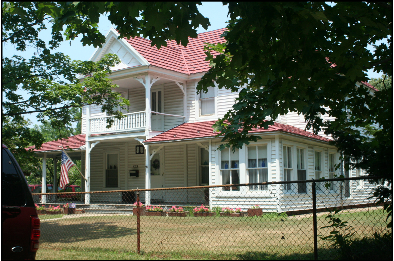
Looking northwest, 5712 Ruatan Street ( EHT Traceries , 2007)
