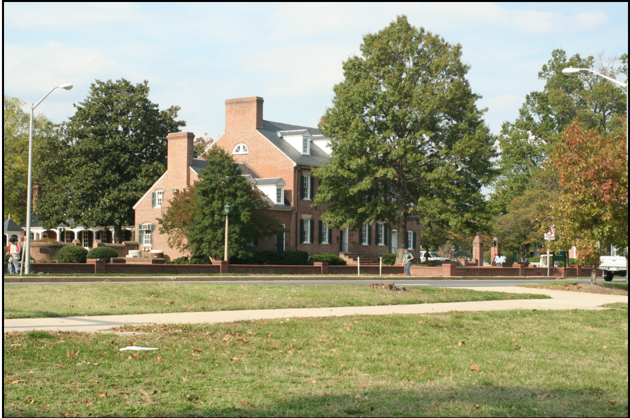
Looking northwest, Rossborough Inn (PG: 66-035-02), southeast corner, façade ( EHT Traceries, 2007 )
