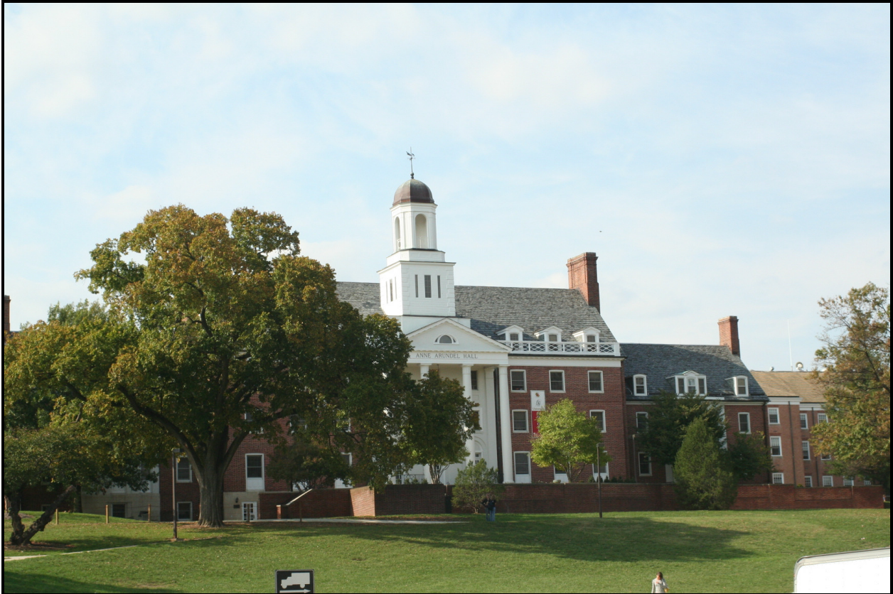
Looking northwest, Anne Arundel Hall, façade ( EHT Tracerics, 2007 )
