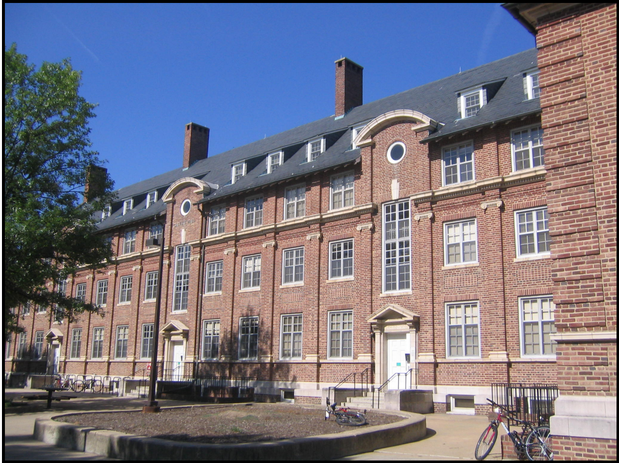
Looking west, Calvert Hall (PG: 66-035-07), façade ( EHT Traceries , 2007)
