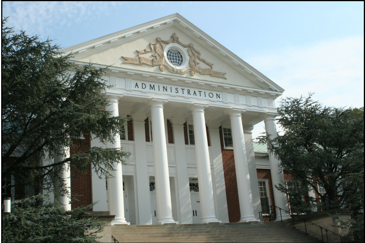
Looking east, Main Administration Building, façade ( EHT Traceries , 2007)
