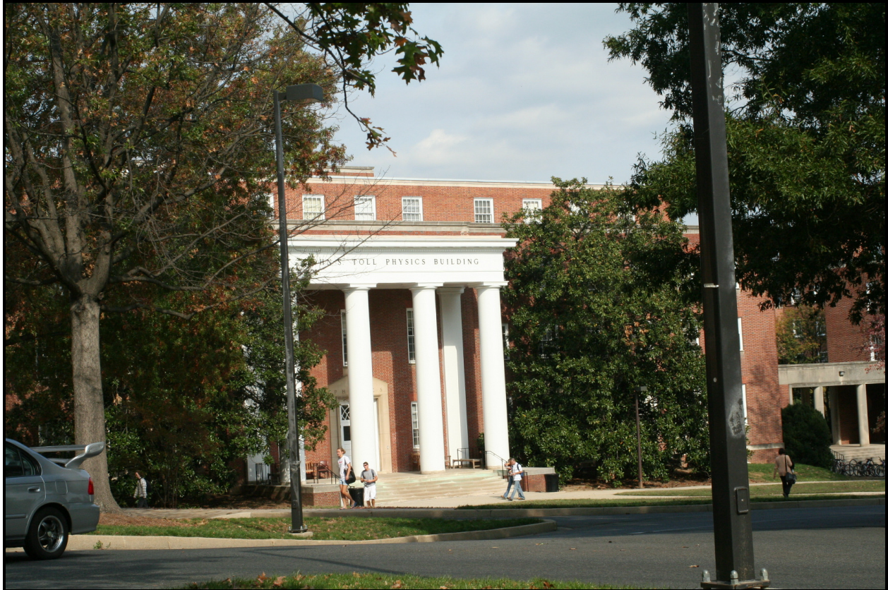
Looking north, Physics Building, façade ( EHT Tracerics, 2007 )
