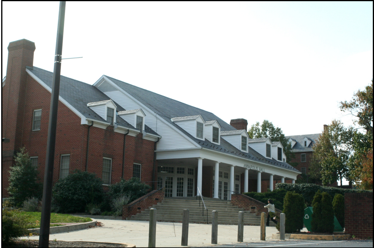
Looking southwest, Annapolis Hall, façade ( EHT Traceries , 2007)
