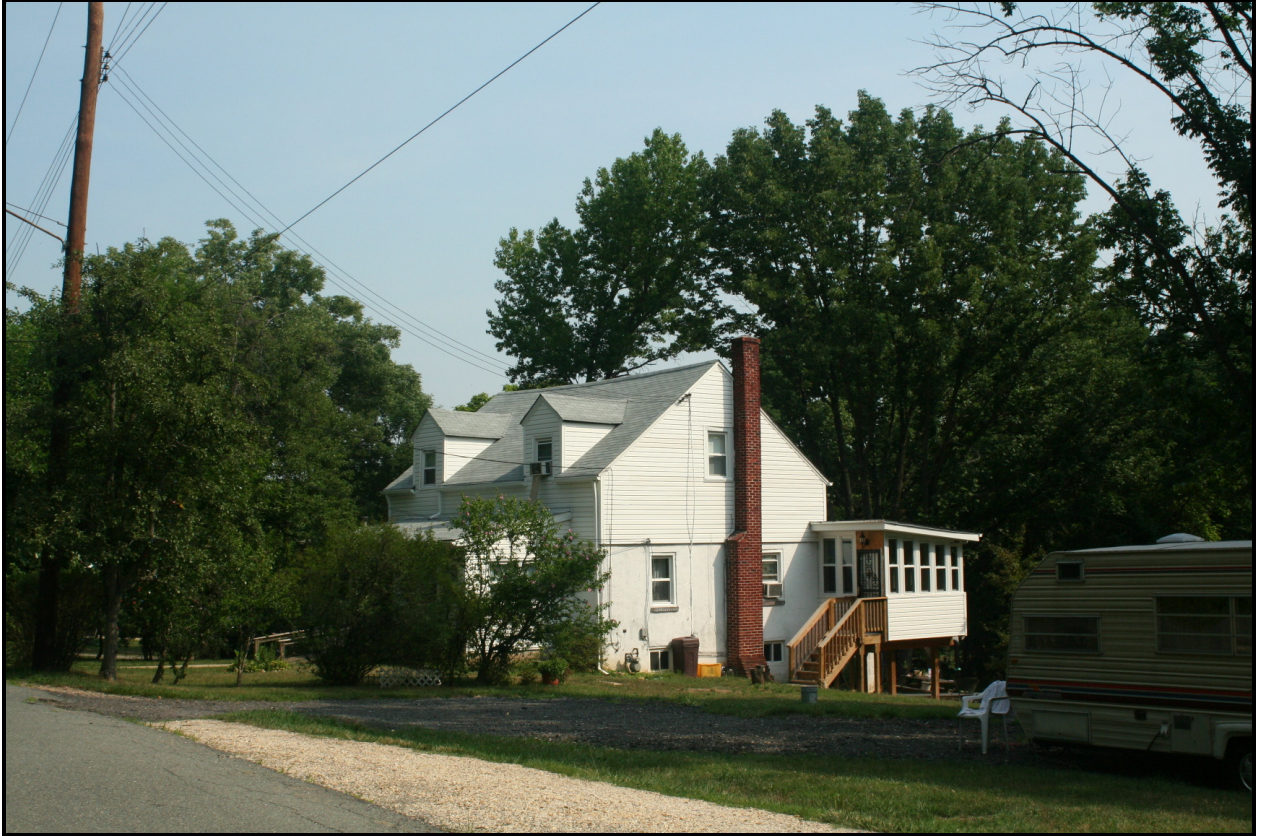
Looking northwest, 7710 Old Muirkirk Road. ( EHT Traceries , 2007)
