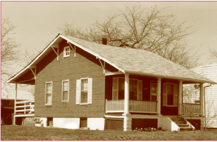
LEFT: This dwelling at 4508 40th Street was an excellent example of an early-twentieth-century suburban bungalow. Note the decorative brackets at the roof line and closely spaced porch balusters. The original wood siding had been covered with brick-textured asphalt siding when this photo was taken in 1990. The house was demolished in 2006.
