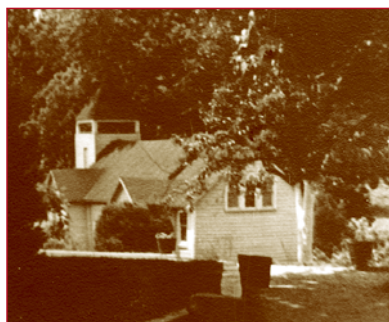
ABOVE: Shown here before 1903, St. Simon's was a front-gabled meetinghouse-style church of wood frame construction, typical of country chapels of the period. Below: This 1942 photo of St. Simon's shows that a square bell tower with a pyramid-shaped roof was added at some point. The church has also been painted a light color. By 1959 it would be clad in dark asphalt shingles. (Both photos courtesy the Reverend Francis P. Willes, St. Thomas' Parish Archives.)
