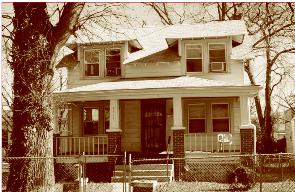
This substantial early twentieth-century Craftsman-style house at 4511 40th Street has exposed rafter tails and large, hip-roof engaged dormers. The brick piers with tapered wood half-columns are original but the widely-spaced balusters are a later addition.
