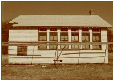
BELOW: The east facade of the 1923 schoolhouse. Note the unusual row of two-over-two windows, each surmounted by the three-light transom.
