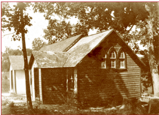
ABOVE: Shown here before 1903, St. Simon's was a front-gabled meetinghouse-style church of wood frame construction, typical of country chapels of the period. Below: This 1942 photo of St. Simon's shows that a square bell tower with a pyramid-shaped roof was added at some point. The church has also been painted a light color. By 1959 it would be clad in dark asphalt shingles. (Both photos courtesy the Reverend Francis P. Willes, St. Thomas' Parish Archives.)
