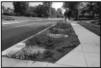
Example of a stormwater filter strip
