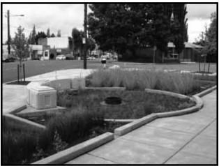
Example of a green street with integrated environmental site design (ESD) stormwater management features
