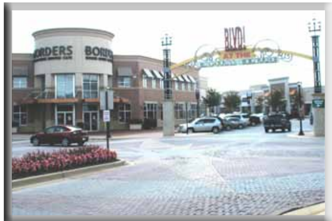
The Boulevard at the Capital Centre
