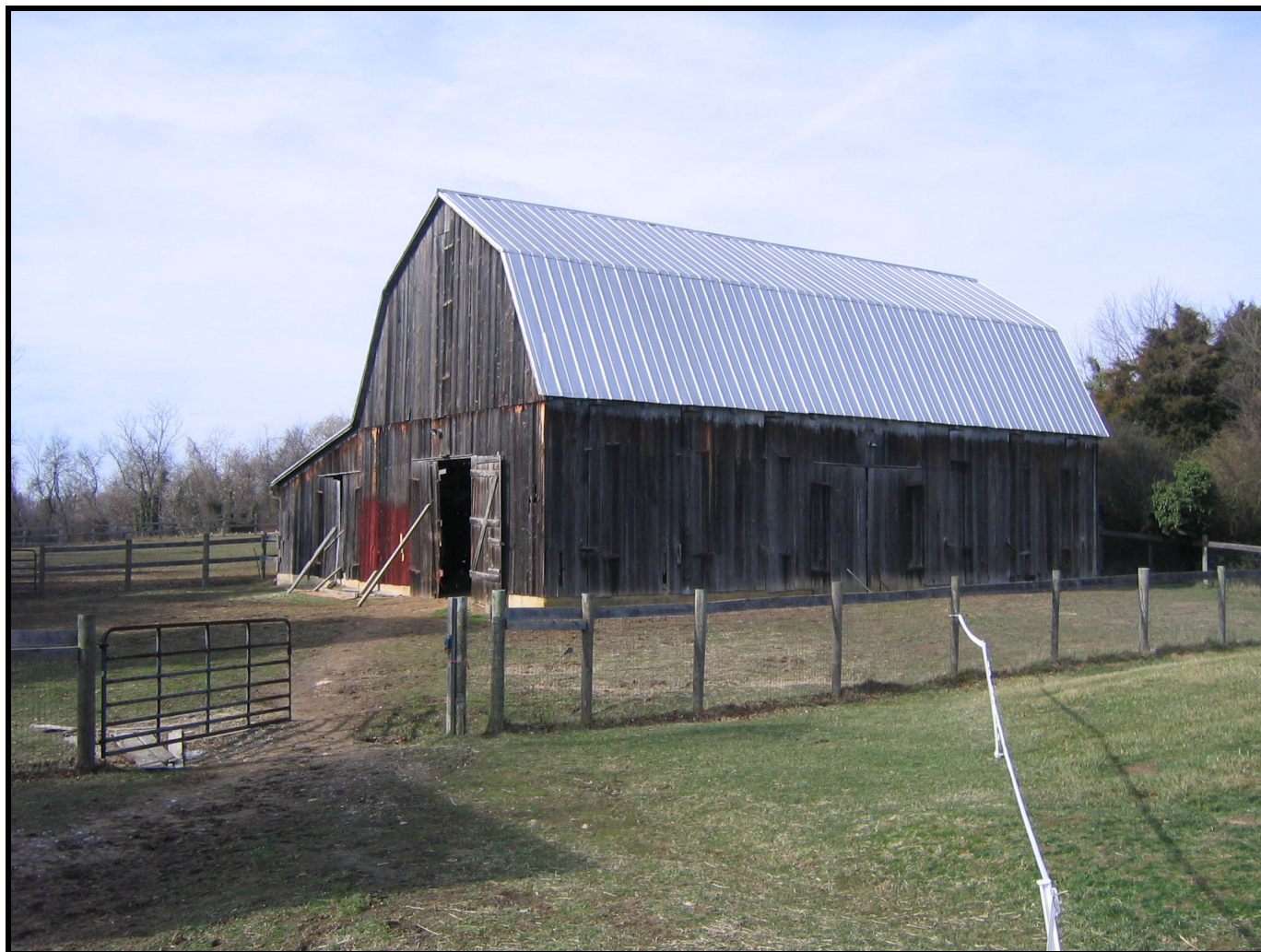
Photo: Barn #2, c. 1920, southeast corner, looking northwest. (January 2008)
