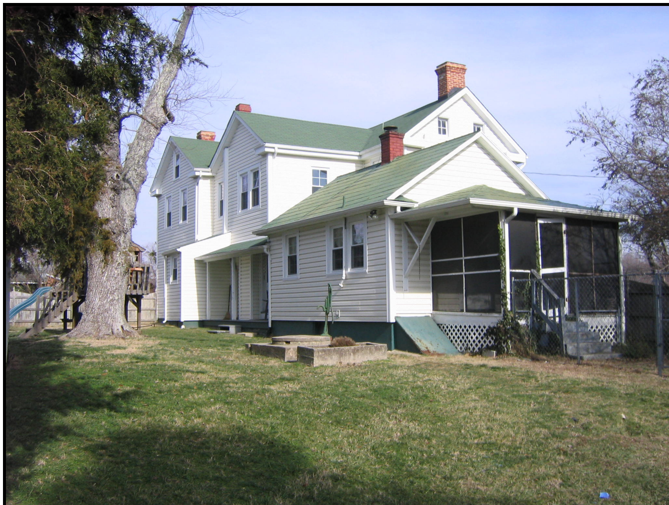
Photo: Mary C. B. Cochrane House, c. 1875, west (rear) elevation, looking northeast. (January 2008)
