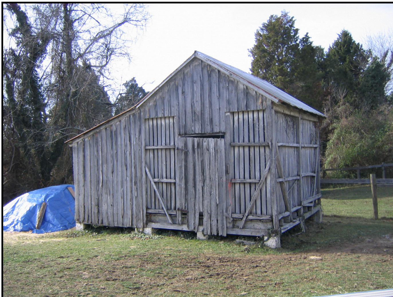
Photo: Barn #1, c. 1900, façade (east elevation), looking southwest. (January 2008)
