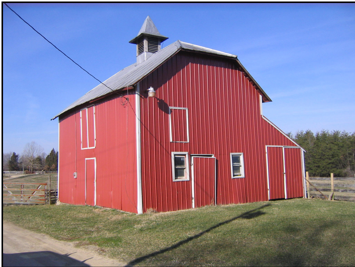
Photo: Barn (2), c. 1888, view of the southeast corner, looking northwest. (January 2008)
