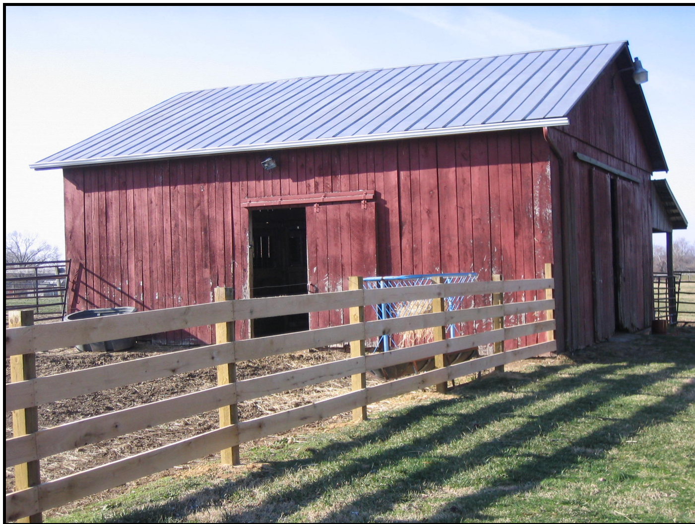
Photo: Barn (1), c. 1940, view of the east elevation, looking southwest. (January 2008)
