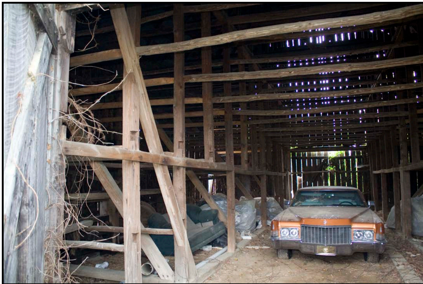
Photo: Sasscer Tobacco Barn, Brandywine, interior, view looking southeast. (August 2009)
