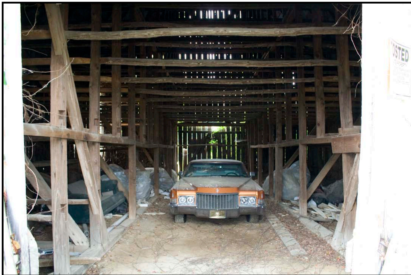
Photo: Sasscer Tobacco Barn, Brandywine, interior, view looking south. (August 2009)
