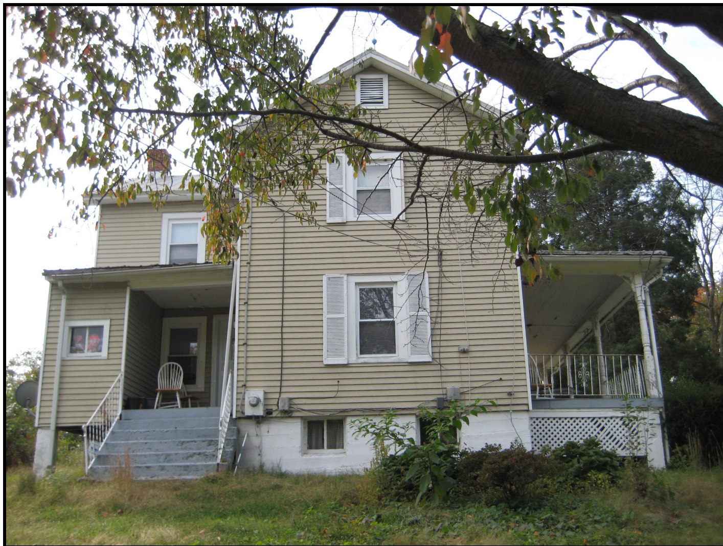
Photo: Proctor House, view of the east (side) elevation, looking west. (November 2007)
