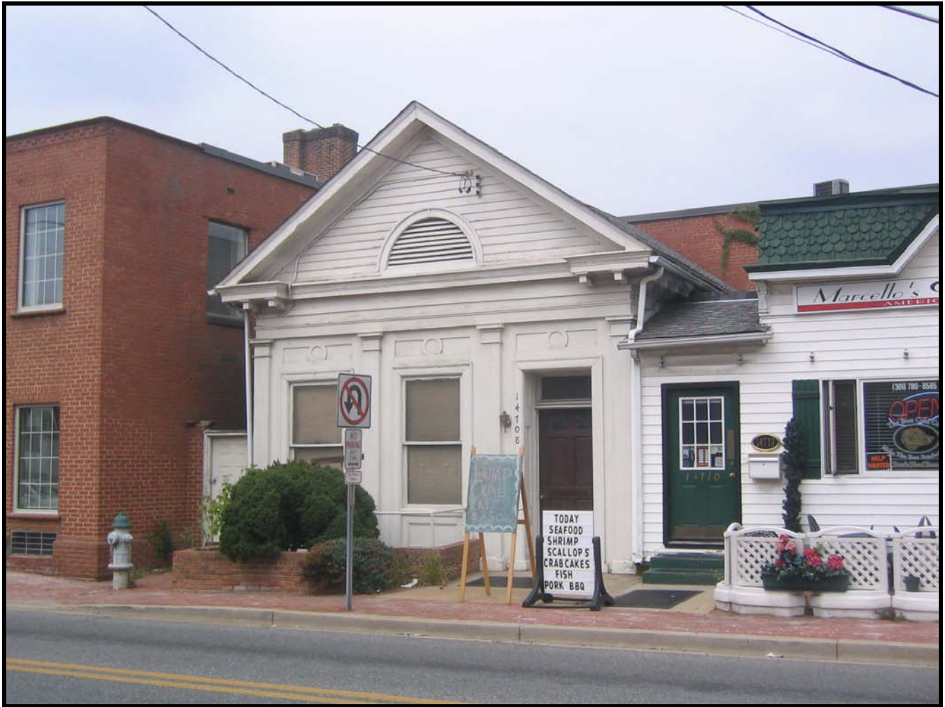
Photo: Magruder Law Office, view of the façade (south elevation), looking northwest. (August 2007)
