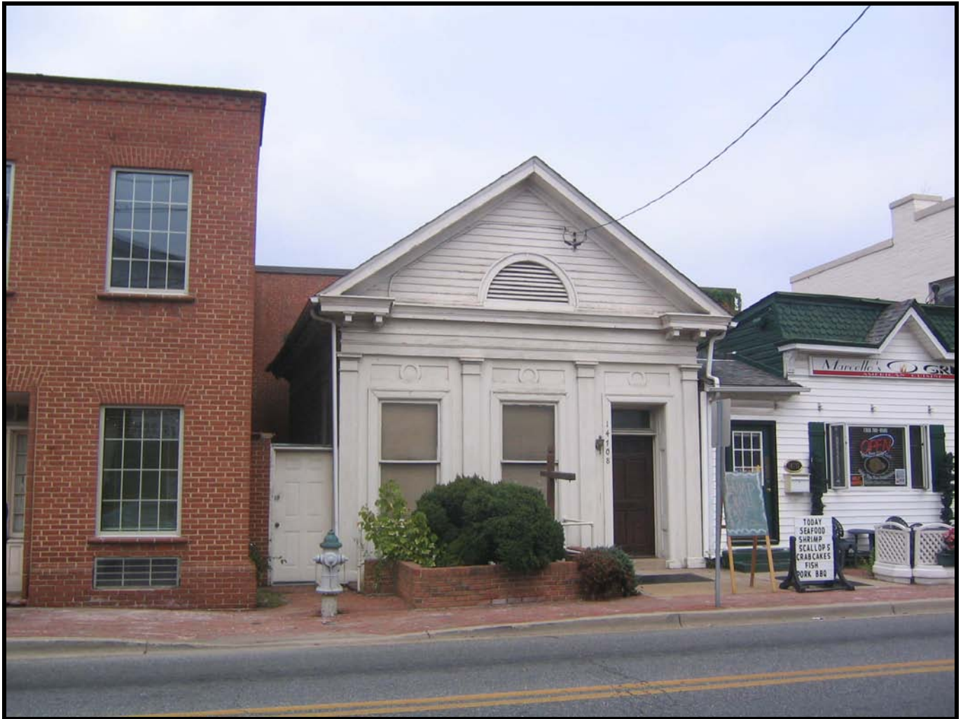
Photo: Magruder Law Office, view of the façade (south elevation), looking northeast. (August 2007)
