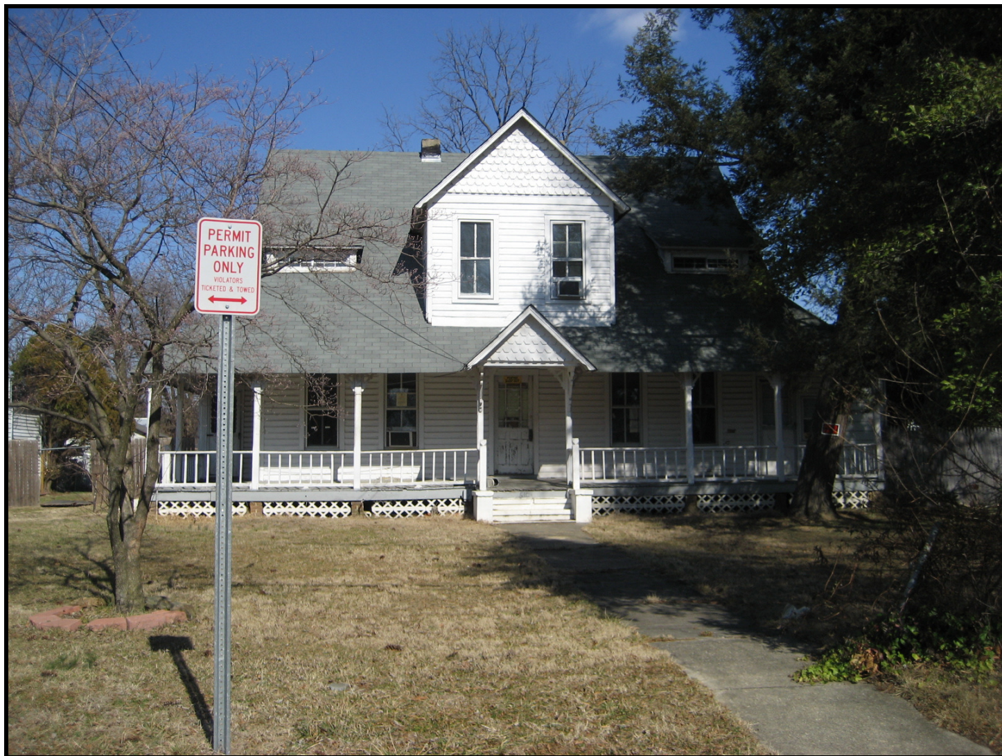
Photo: Poppleton-Roberts House, Edmonston, façade (south elevation), view looking north. (February 2009)
