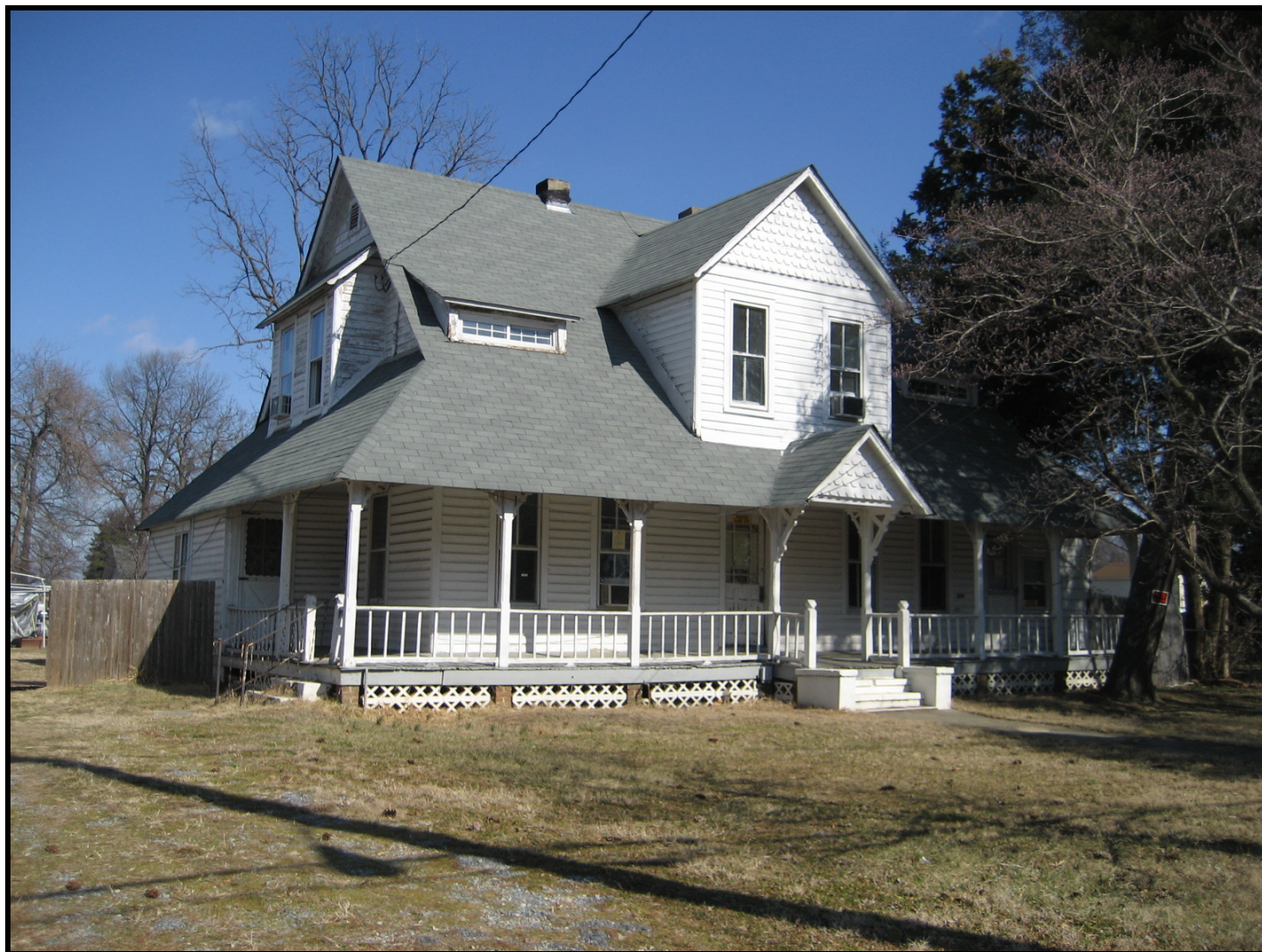
Photo: Poppleton-Roberts House, Edmonston, façade (south elevation), view looking northeast. (February 2009)
