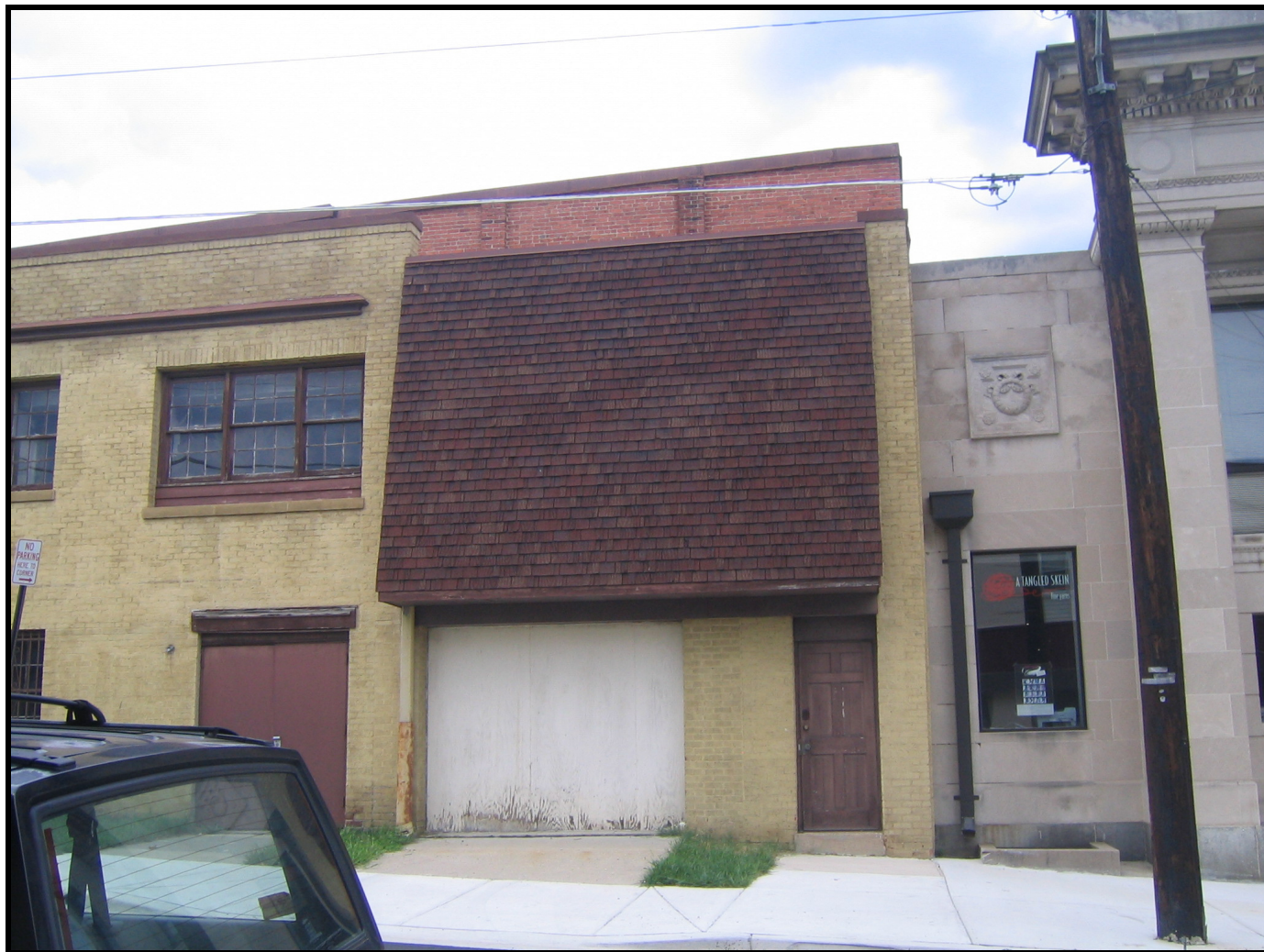
Photo: Professional Building, view of the south elevation addition, looking north.
