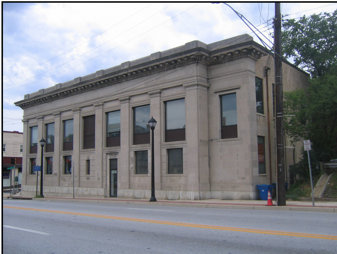
Photo: Professional Building, view of the façade (east elevation), looking southwest.
