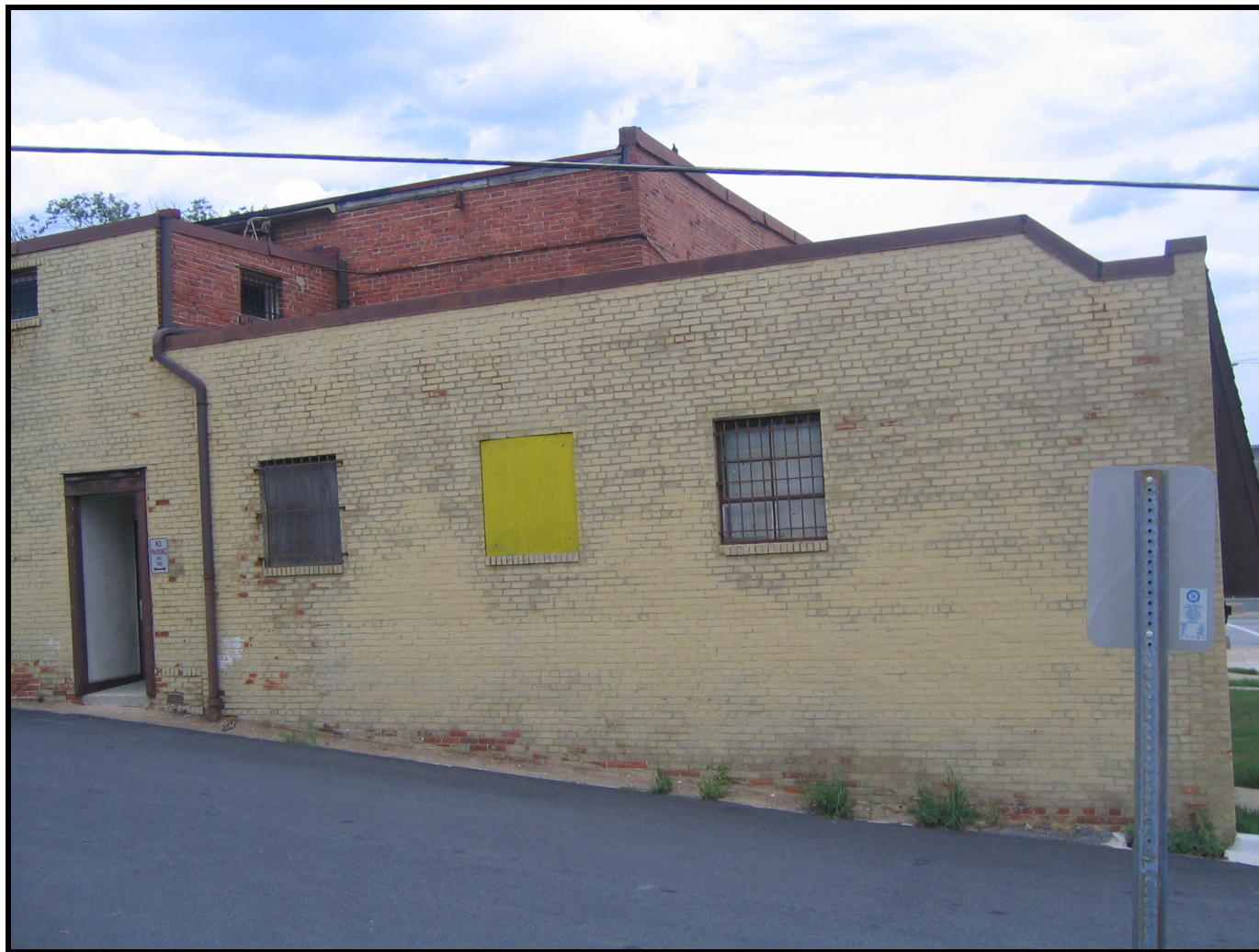
Photo: Professional Building, view of the west elevation, looking east.
