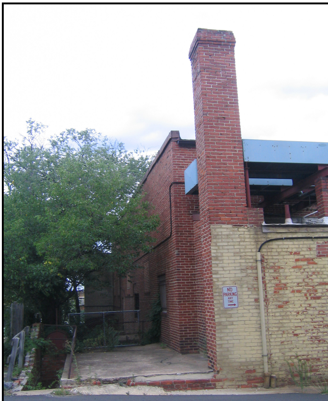
Photo: Professional Building, view of the north elevation, looking east.
