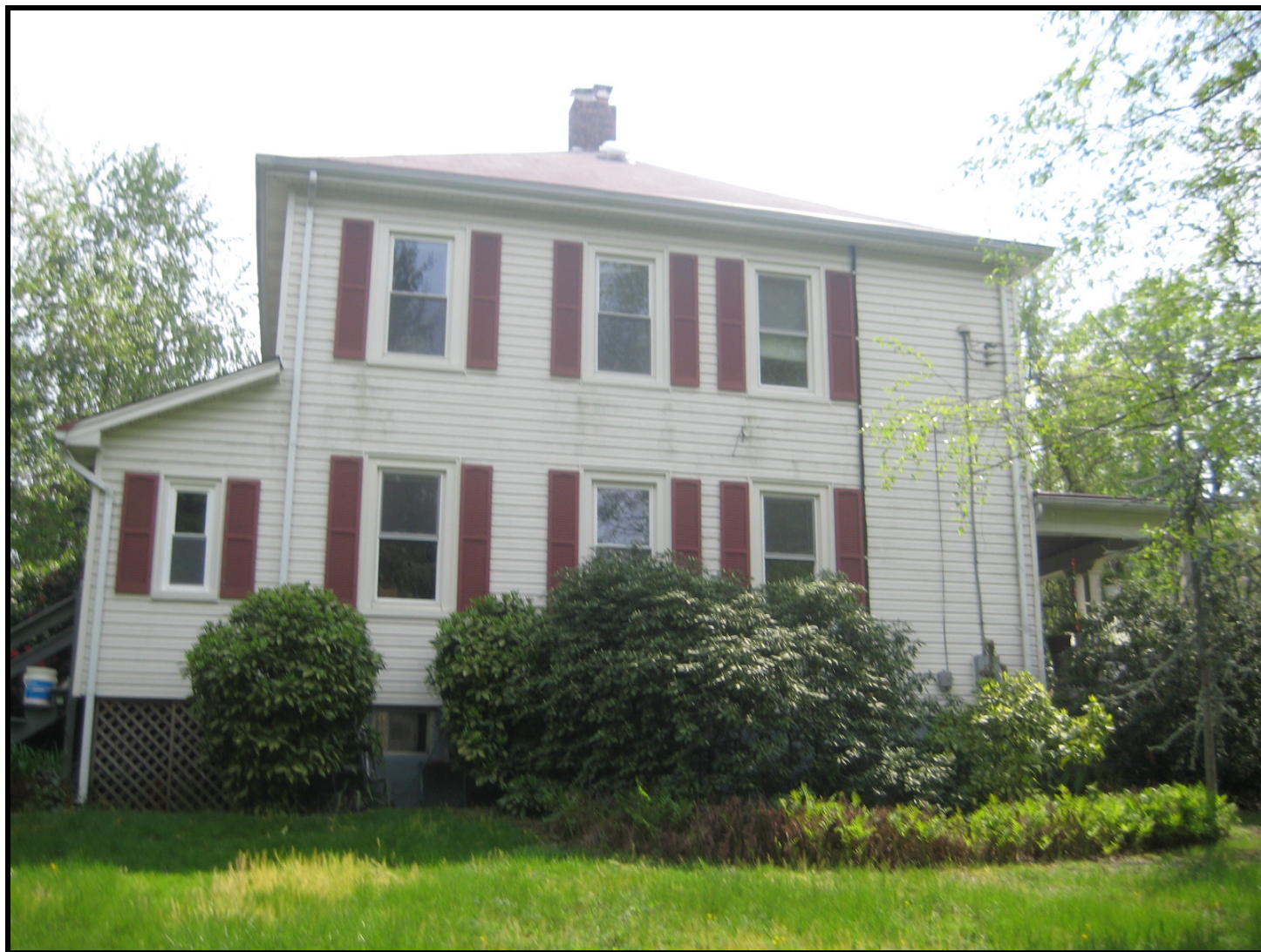
Photo: Traver-Williams House, Berwyn Heights, north (side) elevation, looking south. (April 2008)
