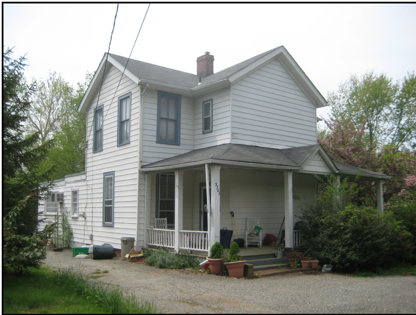
Photo: Yoos House, Berwyn Heights, view of the façade (north elevation), looking southwest. (April 2008)
