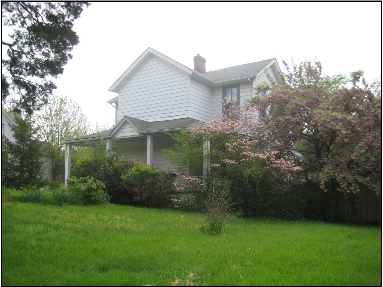
Photo: Yoos House, Berwyn Heights, view of the façade (north elevation), looking southeast. (April 2008)
