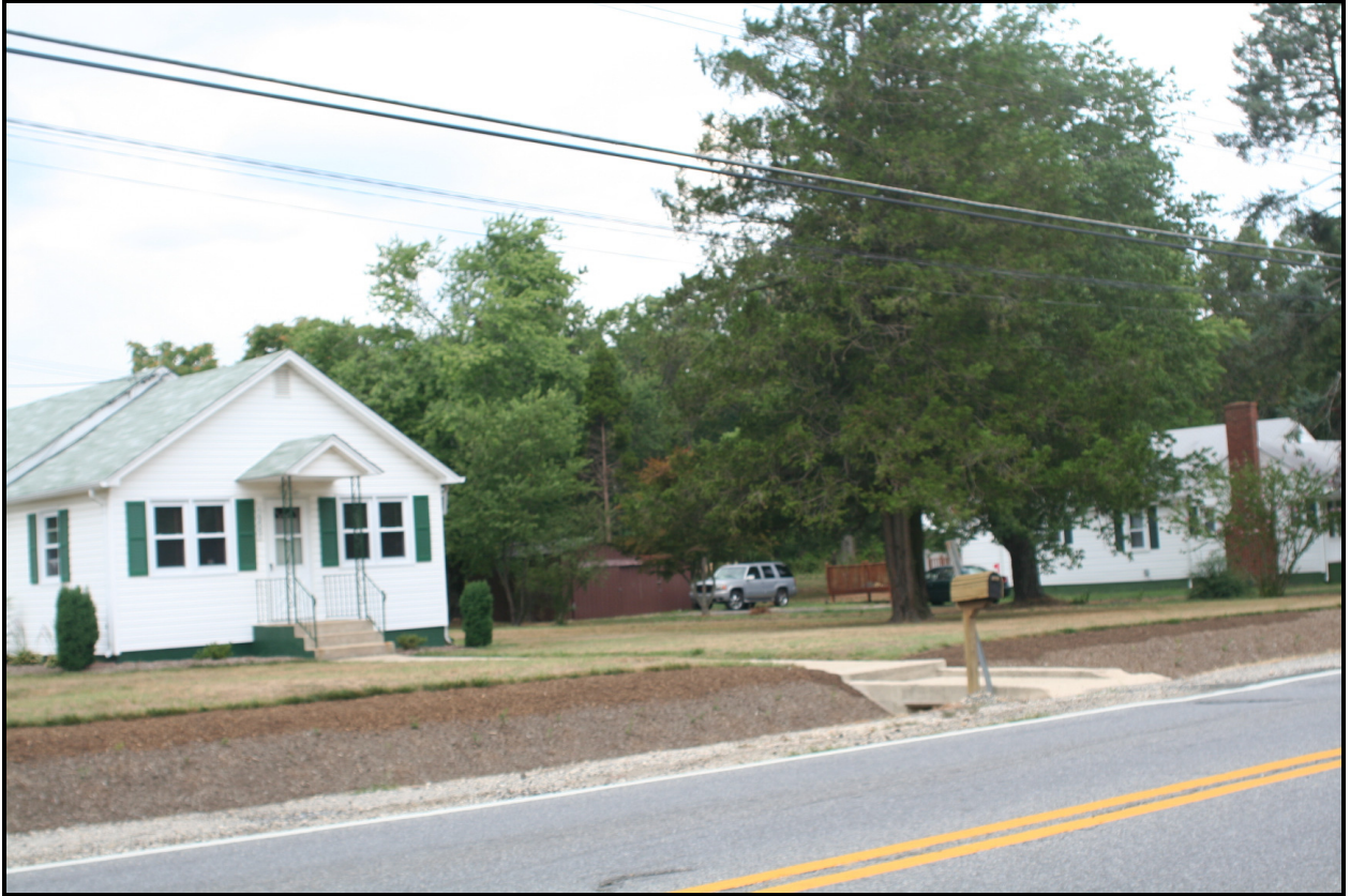
Looking northwest, 10807-10805 Frank Tippett Road ( EHT Traceries , 2007)
